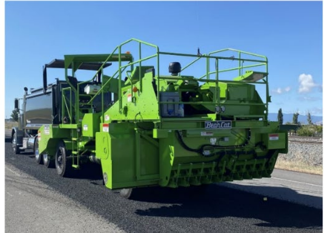
d) Spreading of Aggregate
