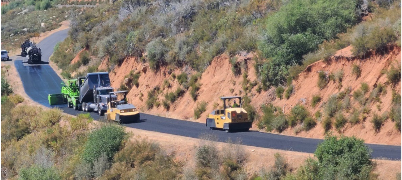
Figure 7-17 Overall View of a Chip Seal Operation
