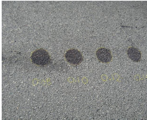
Figure 6-8 Completed Ring Tests
