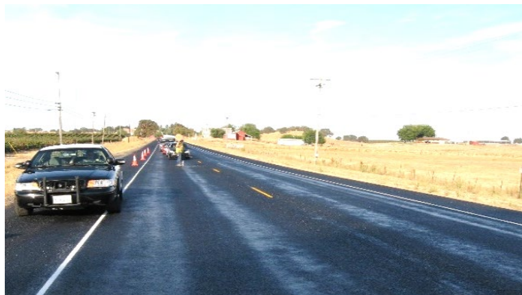
Figure 6-3 Dense Graded HMA with Closed Surface with Bleeding, Not Suitable for Fog Seal or Rejuvenator Seal
