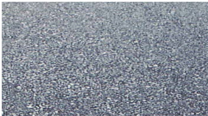
Figure 6-4 Three-year-old Suitable Surface, Open Graded HMA for Fog Seal or Rejuvenator Seal
