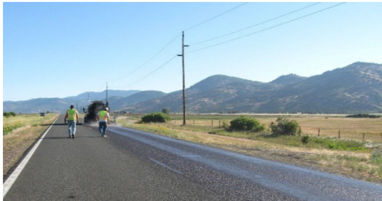
Figure 6-1 Fog Seal Application
