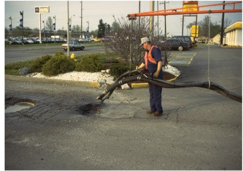
b) Application of Tack Coat
