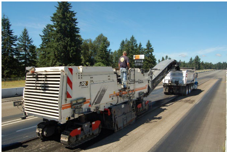
Figure 5-16 Milling Out the Distressed Area
