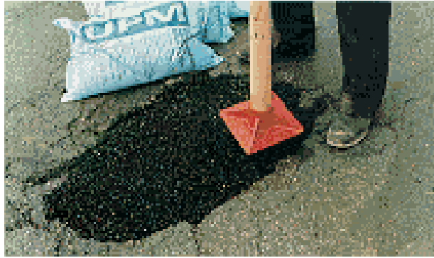
Figure 5-1 Quick Patch Material in Pothole
