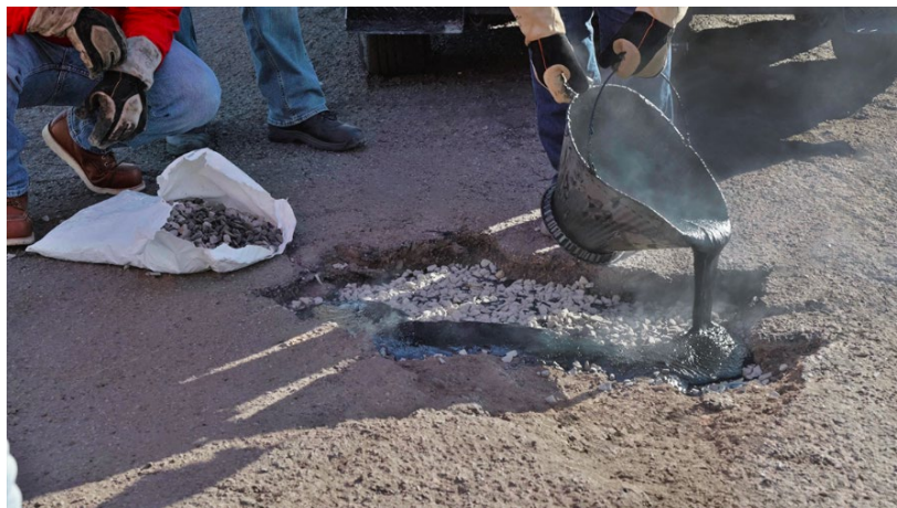
Figure 5-9 Application of Hot Mastic With 'Bulking Aggregate' (Courtesy Crafcro)
