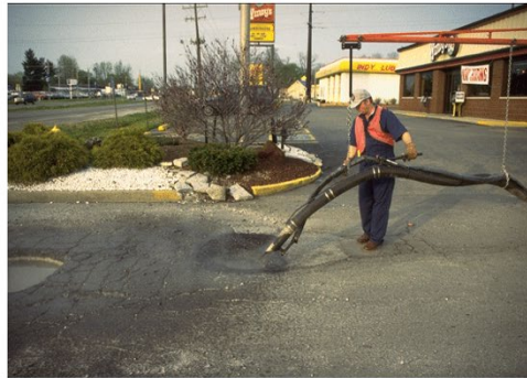
c) Filling the Prepared Hole
