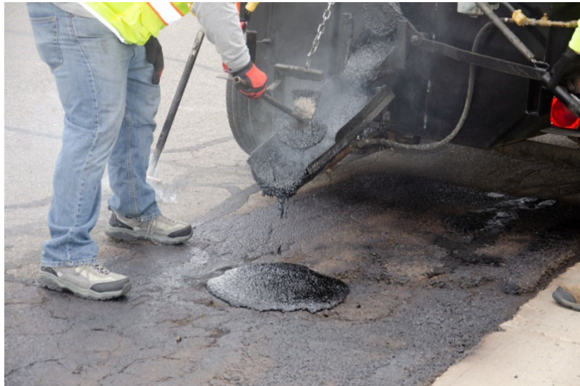
Figure 5-8 Hot Mastic Placement (Courtesy of Maxwell Products)
