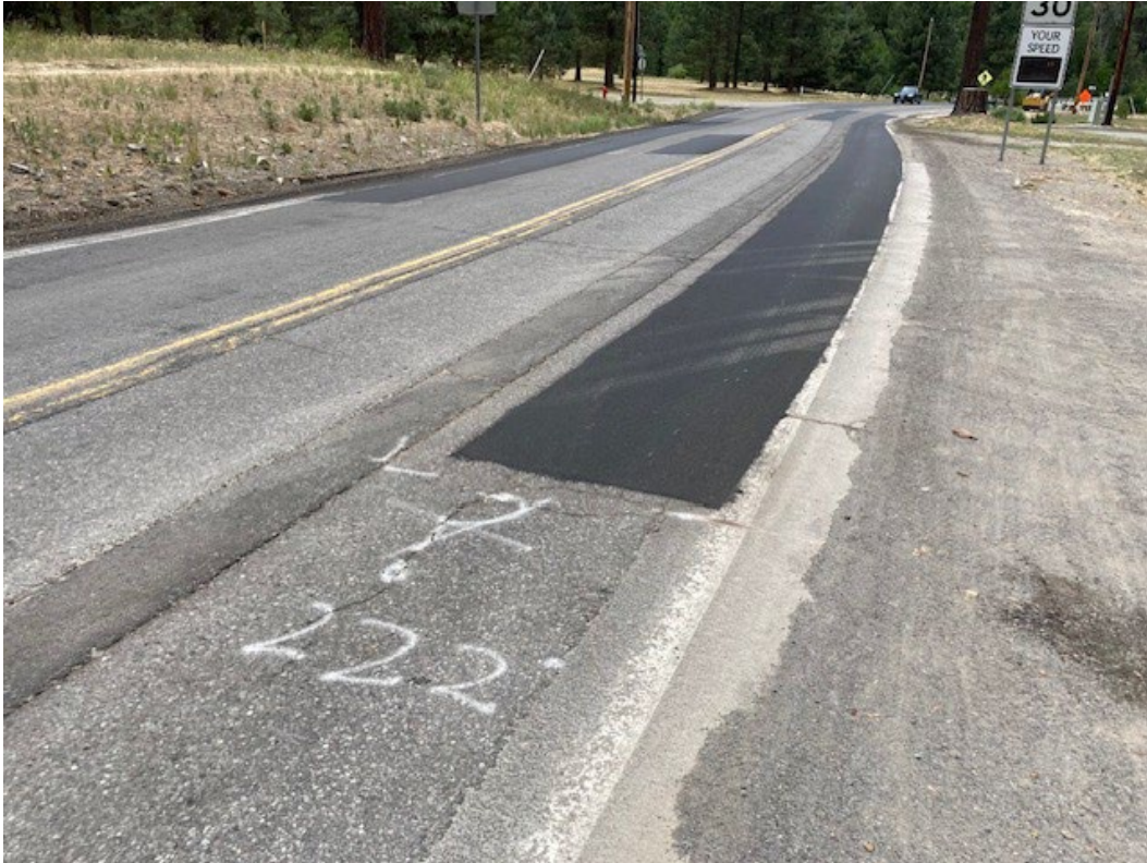
Figure 5-12 Continuous Patch in Wheelpaths
