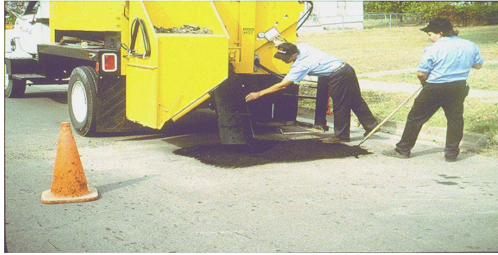
b) Unload Patching Material from Patching Truck
