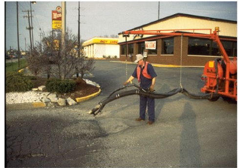
d) Application of Finish Coat
