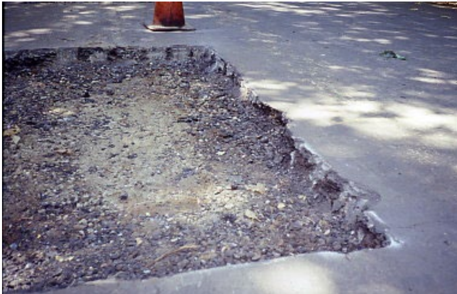
Figure 5-11b Jackhammered Cut Lines
