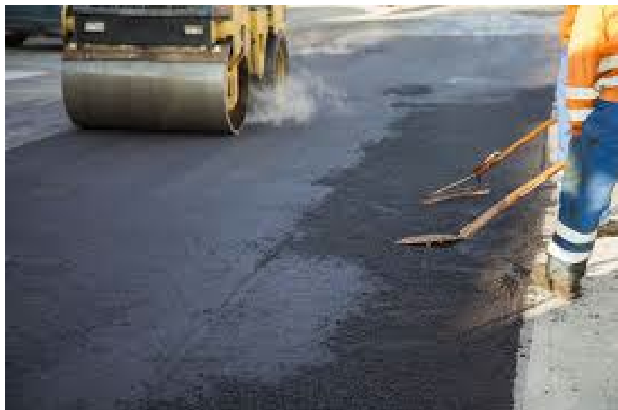
Figure 5-20 Rolling of a Skin Patched Area
