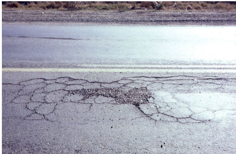
Figure 5-4 Completed Patch Using a Quick-Patch Product
