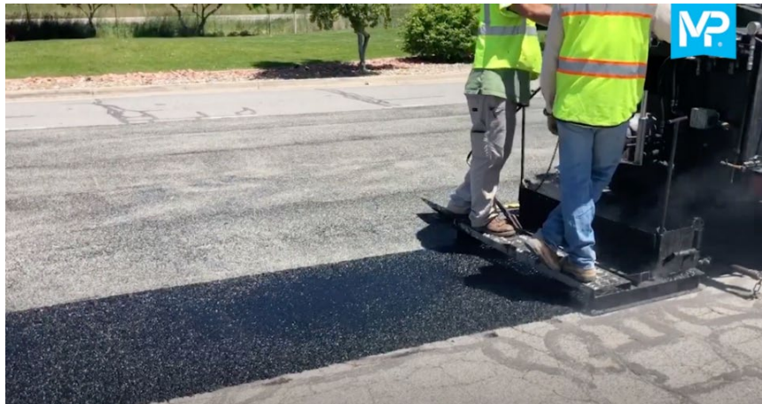
Figure 5-21 Skin Patch with Hot Mastic Material (Maxwell Products)
