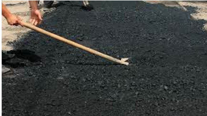
Figure 5-19 Hand Leveling of a Skin Patched Area
