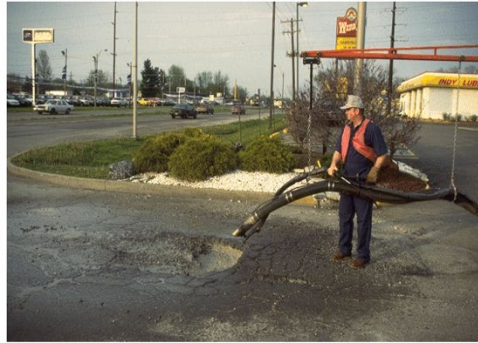
a) Site Preparation
