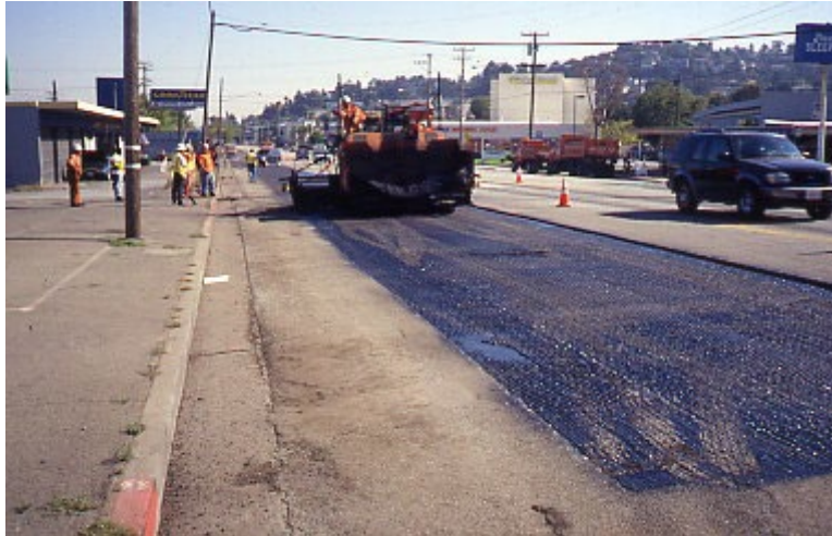
Figure 5-15 Full Lane Width Partial-Depth Milling with Tack Coat
