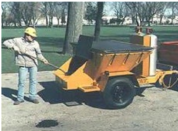
a) Obtaining Hot Patching Materials from Heated Trailer by Hand
