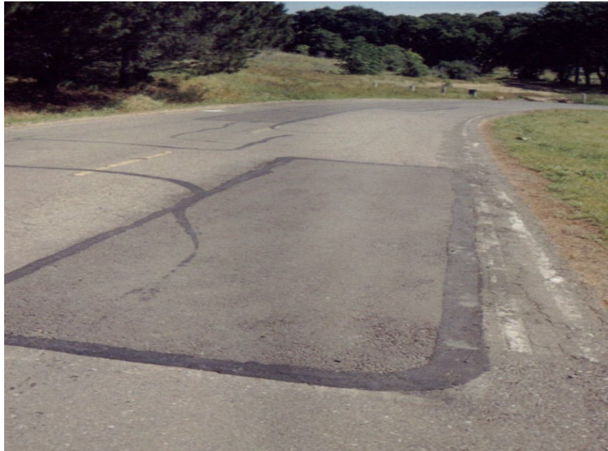
Figure 5-17 Digout Patch with Surface Edge Seal Treatment
