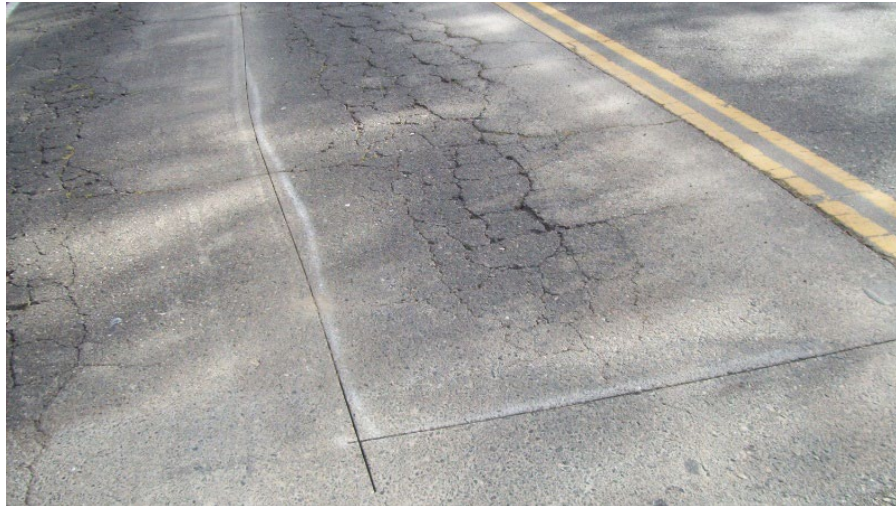
Figure 5-11a Sawcut Lines for a Digout Patch
