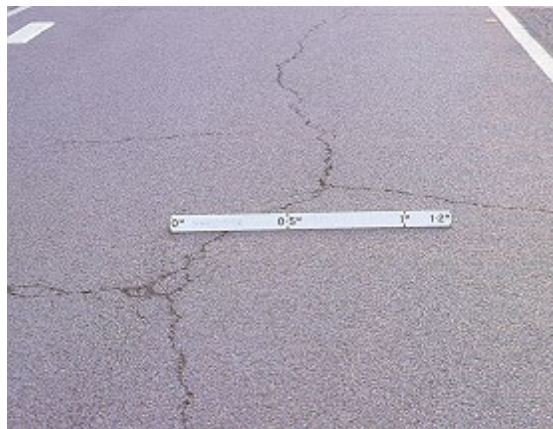
Figure 4-5 Block Cracking
