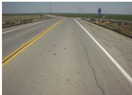
Figure 4-3 Longitudinal Cracking
