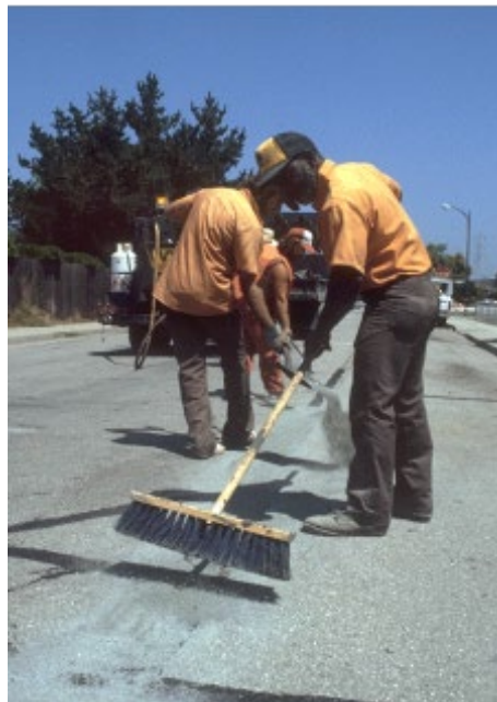
Figure 4-20 Brooming Blotter Sand Coat Over a Treated Crack
