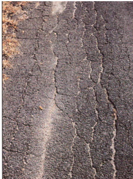
Figure 4-7 Edge Cracking
