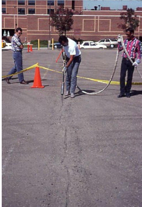
Figure 4-14 Airblast Cleaning of Crack
