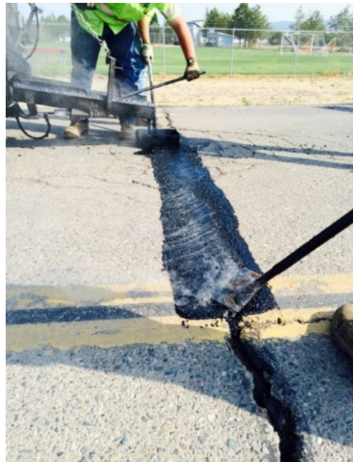
Figure 4-18 Hot Mastic Application
