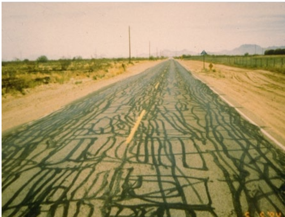
Figure 4-21 Excessive Sealant
