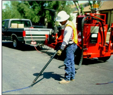
a) Hot Pressure-fed process
