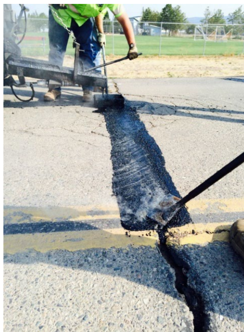
Figure 4-10 Hot Mastic Crack Sealing of a Wide Crack
