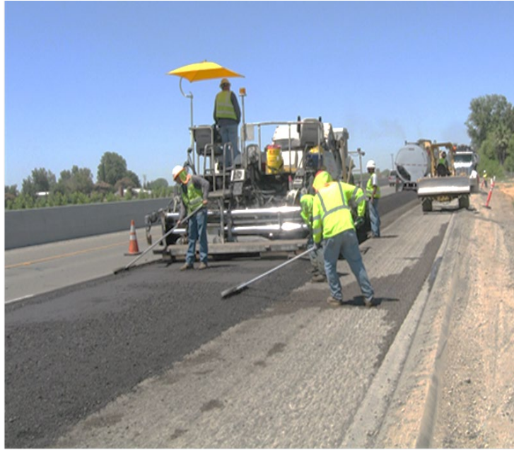
Figure 14-8 PDR Placed with Paver (Courtesy of CP2 Center)
