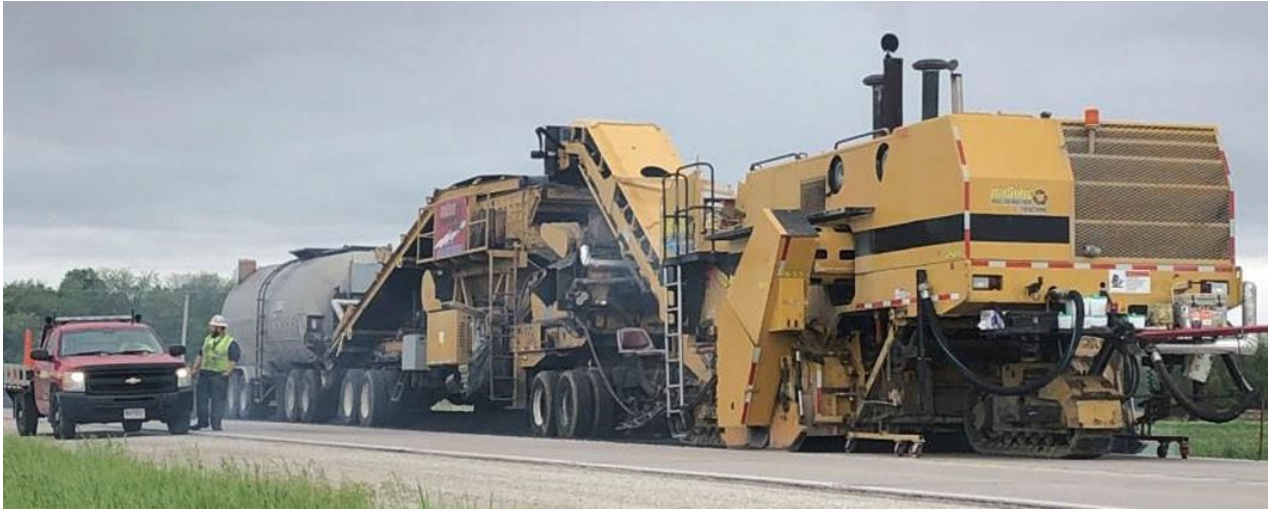
Figure 14-6 PDR Milling Operation (Courtesy Performance Equipment Service Inc.)
