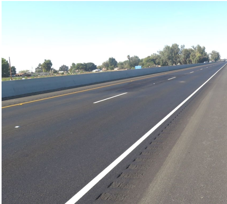
Figure 14-9 Post Construction after RHMA Overlay (Courtesy of CP2 Center)
