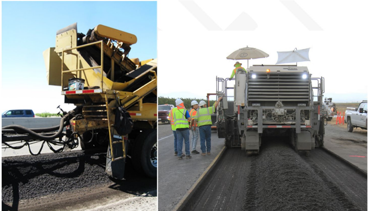
Figure 14-7 PDR in Windrow after Emulsion is Mixed
