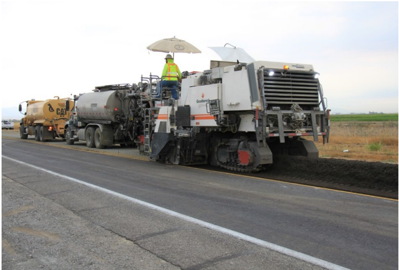
Figure 14-4 PDR Equipment Train
