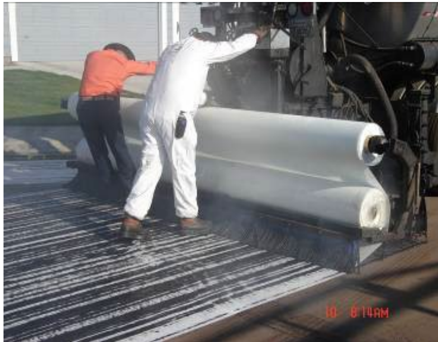
Figure 13-9 Truck Mount Application of Paving Mat
