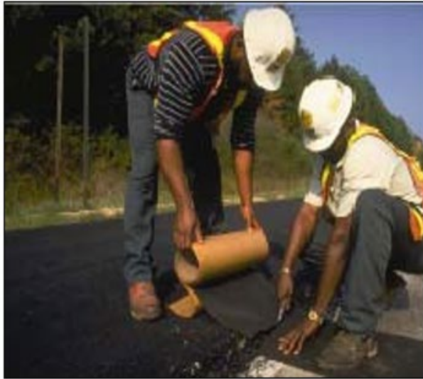
Figure 13-5 Application of Composite Membranes
