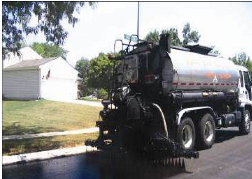
Figure 13-7 Interlayer Binder Application
