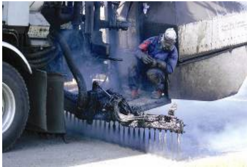
Figure 13-12 Asphalt Rubber Binder Being Applied
