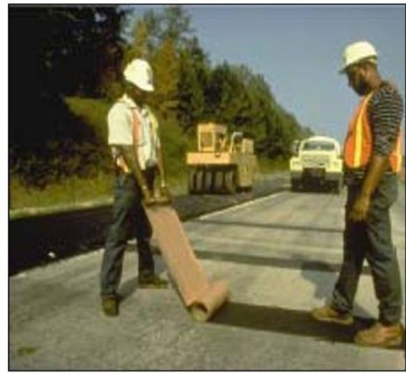
Figure 13-5 Application of Composite Membranes
