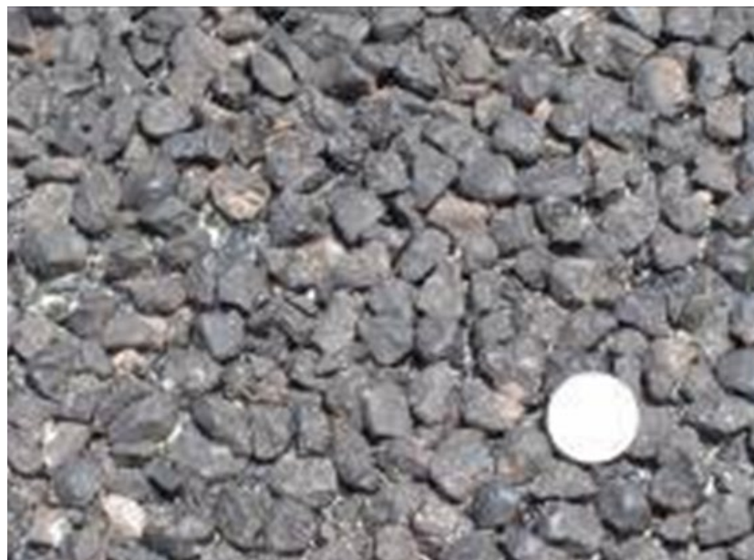
Figure 13-6 Asphalt Rubber Chip Seals
