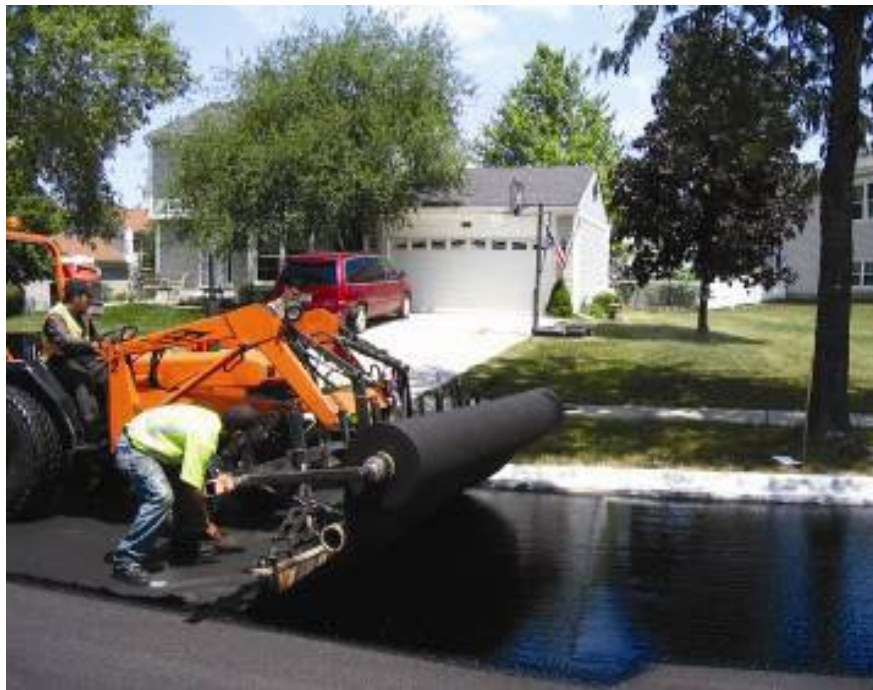
Figure 13-8 Tractor Mount Application of Fabric
