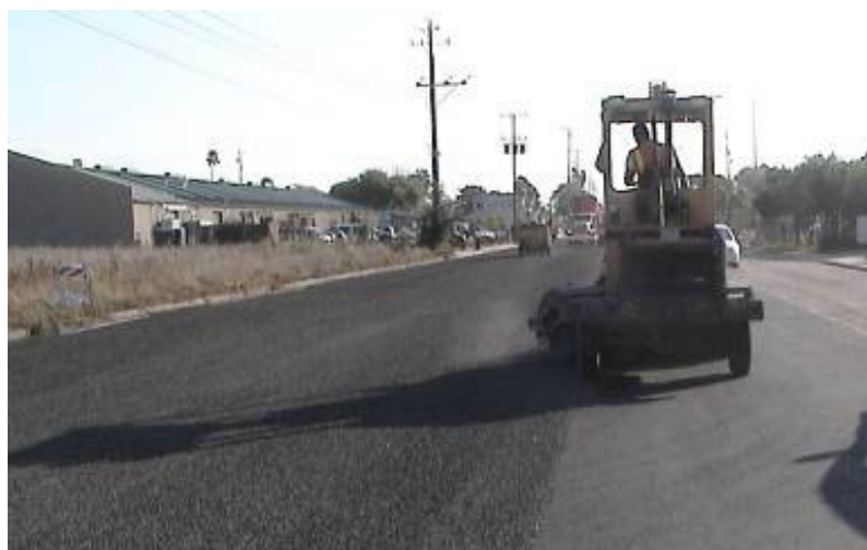
Figure 13-13 Chips Applied and Sweeping Edge for 2 nd Pass
