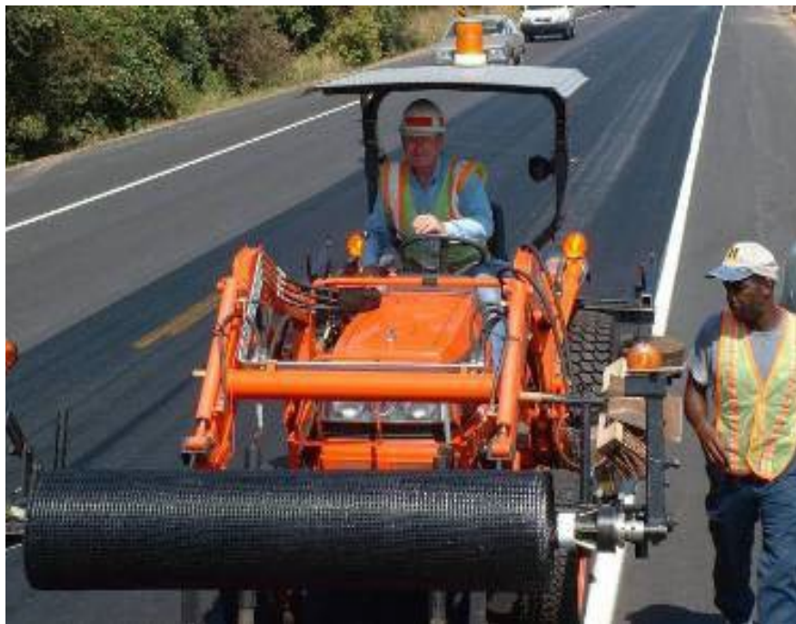
Figure 13-10 Tractor Mount Paving Grid Installation
