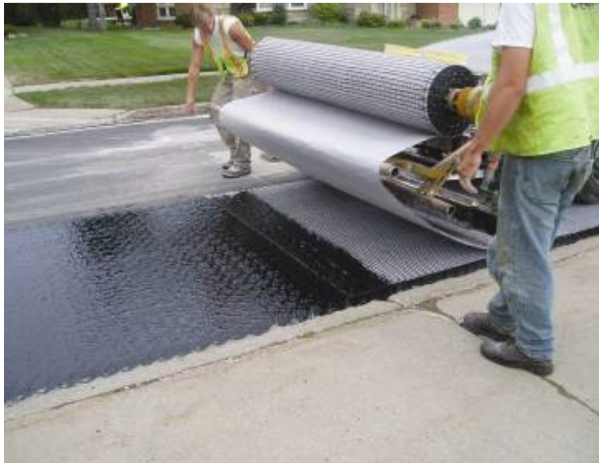
Figure 13-11 Composite Paving Grid Installation
