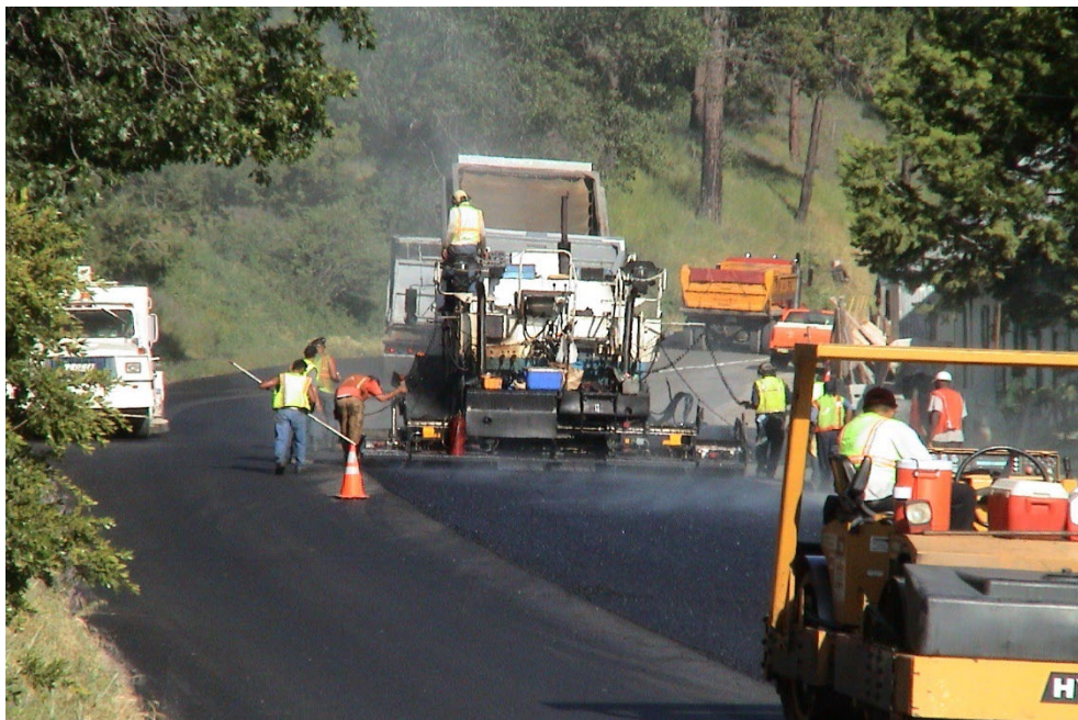
Figure 12-5 Roller Position During Application (Alvarez, 1992)
