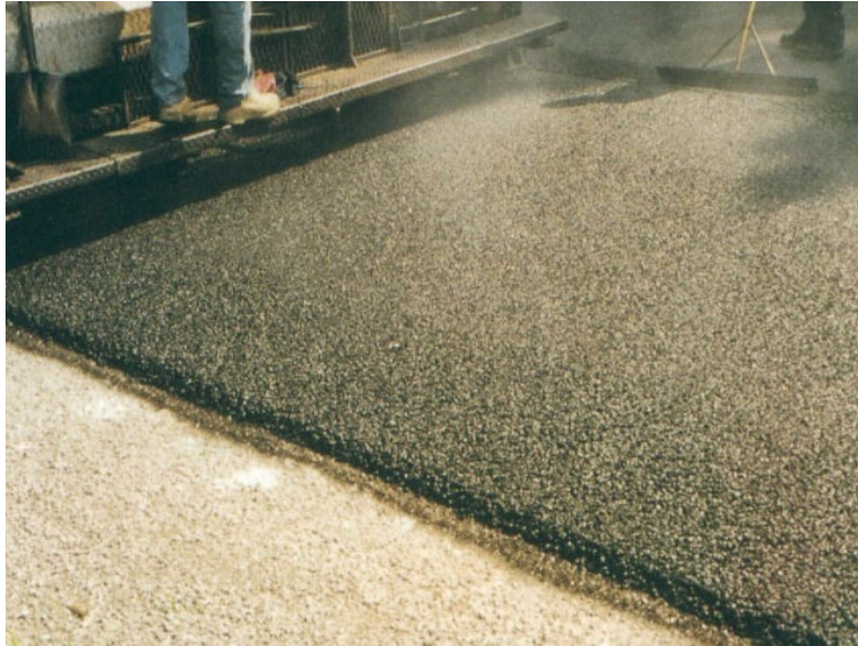
Figure 12-4 Freshly Laid BWC (Alvarez, 1992)
