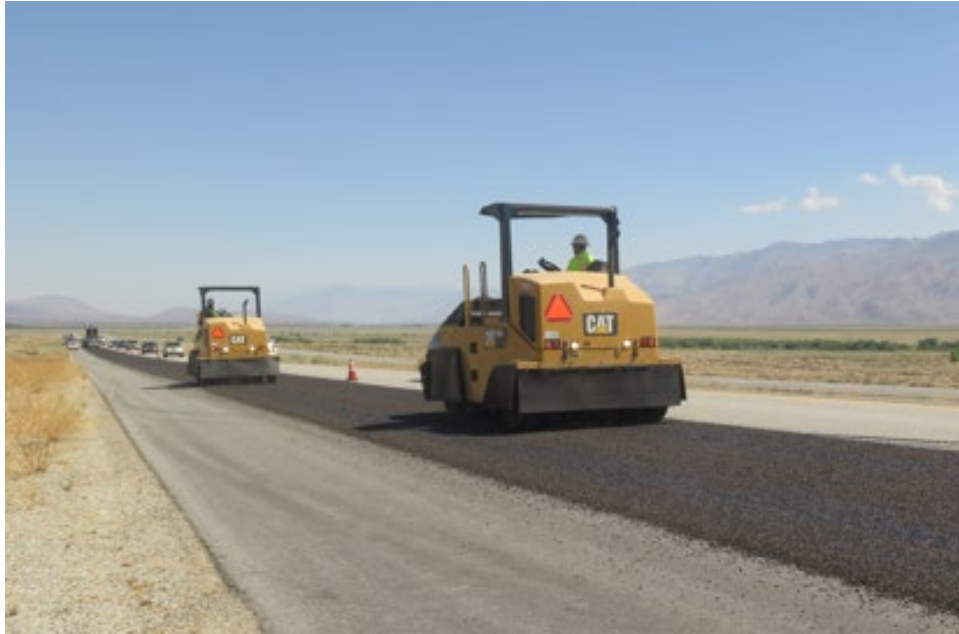
Figure 10-13 Multiple Rollers Compacting Freshly Applied Chips
