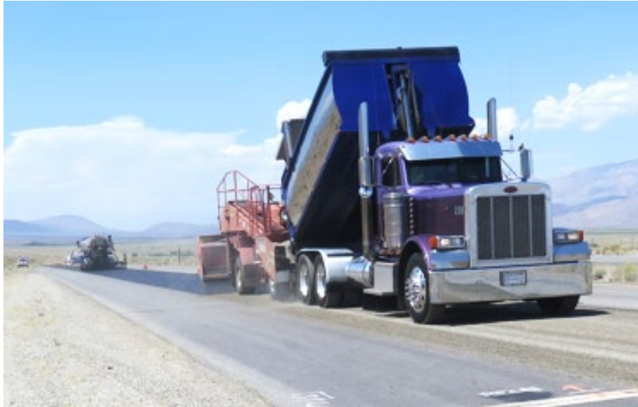
Figure 10-17 Rear-Dump Haul Truck Emptying Chips into Spreader
