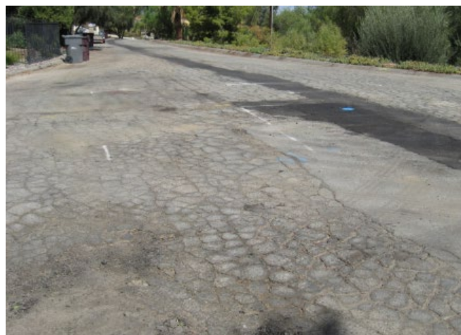
Figure 10-4 PCI < 10 (Very Poor Condition) (Courtesy of County of Riverside Transportation Department, Pavement Management Report 2015)
