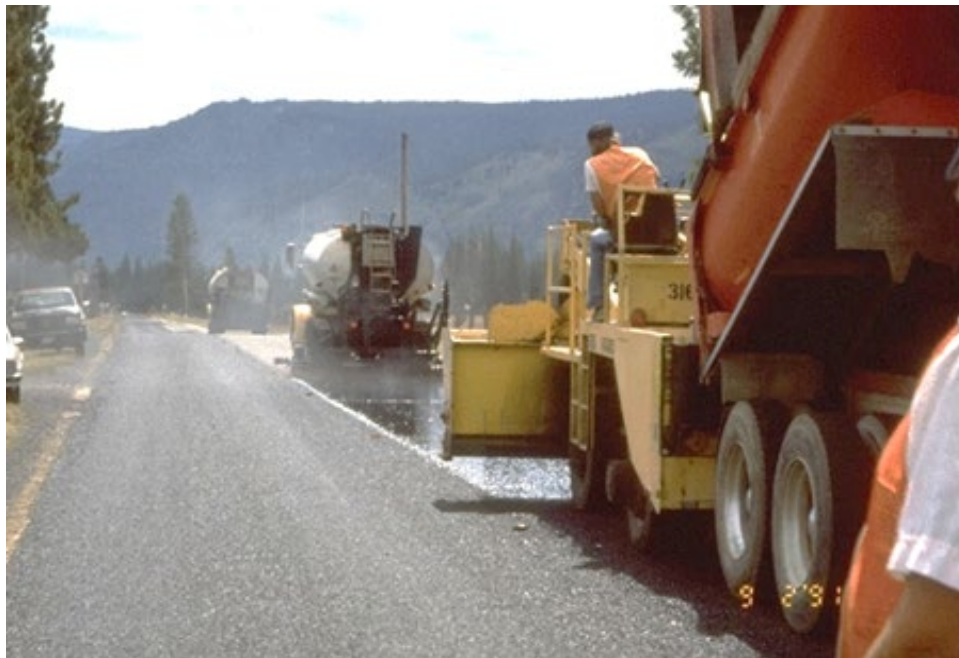
Figure 10-12 Chips Applied by Bear Cat Spreader
