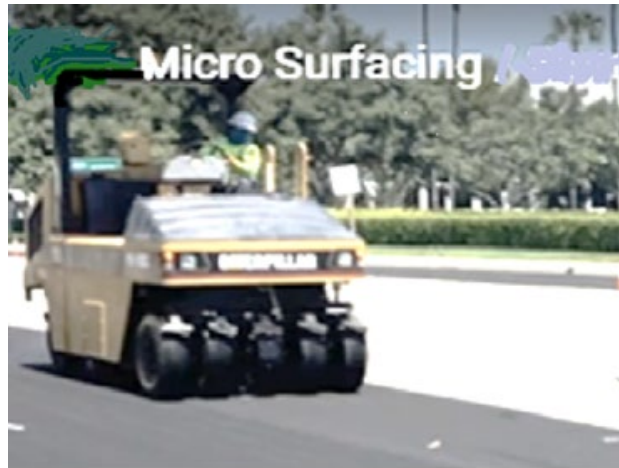
Figure 10-10 Rolling a Micro Surfacing (Courtesy of Scott Metcalf, NPPC2021-S2)
