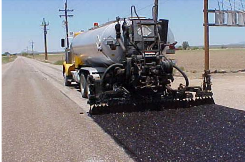
Figure 10-11 Distribution Truck for Chip Seal Binder
