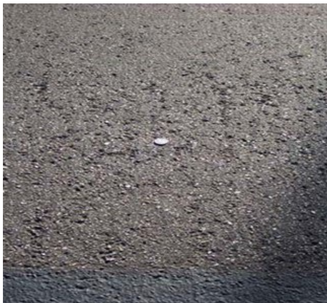
Figure 1-27 Rock Loss
