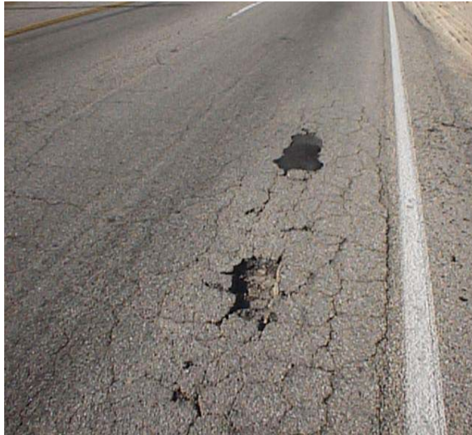
Figure 1-18 Potholes
