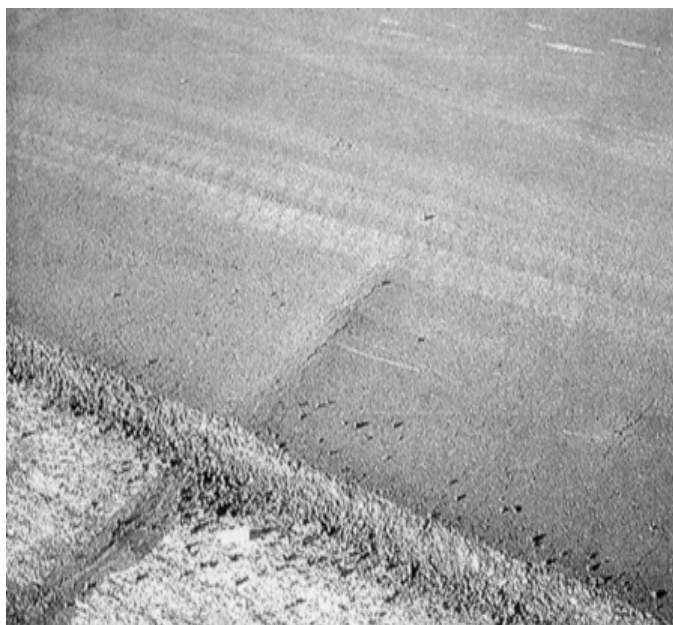
Figure 1-15 Overlay Bumps
