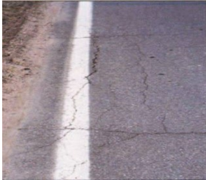
Figure 1-10 Edge Cracks
