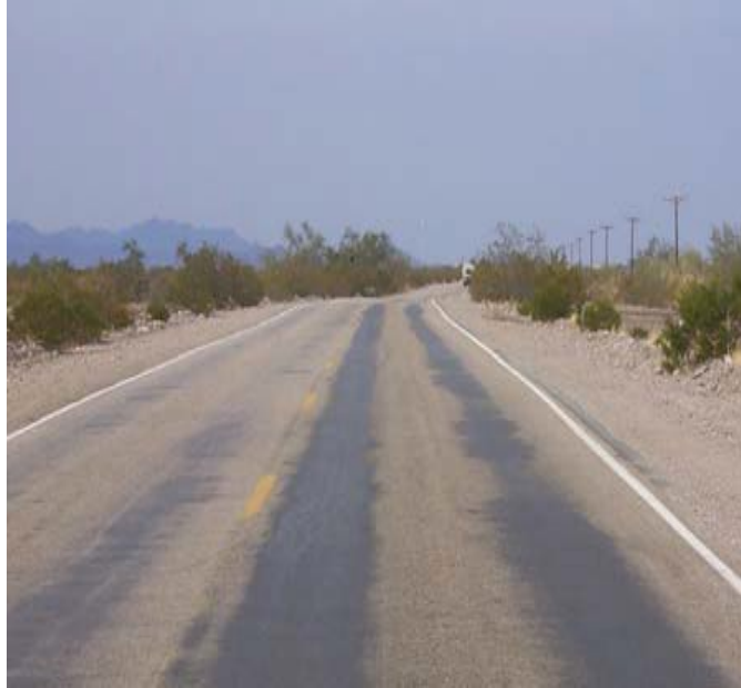
Figure 1-26 Bleeding (HMA)
