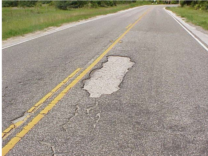
Figure 1-16 Delamination
