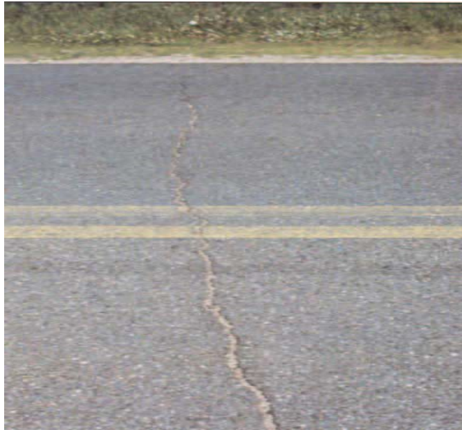
Figure 1-8 Reflective Cracks
