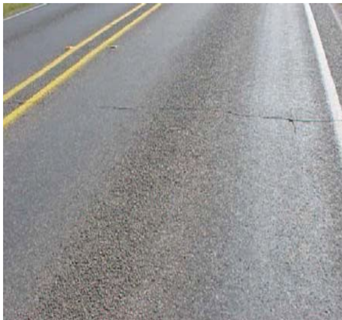
Figure 1-7 Transverse Cracks
