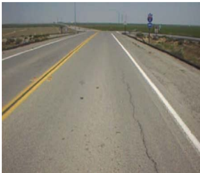
Figure 1-5 Longitudinal Cracks
