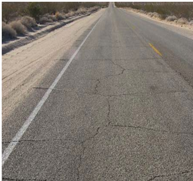
Figure 1-9 Block Cracks
