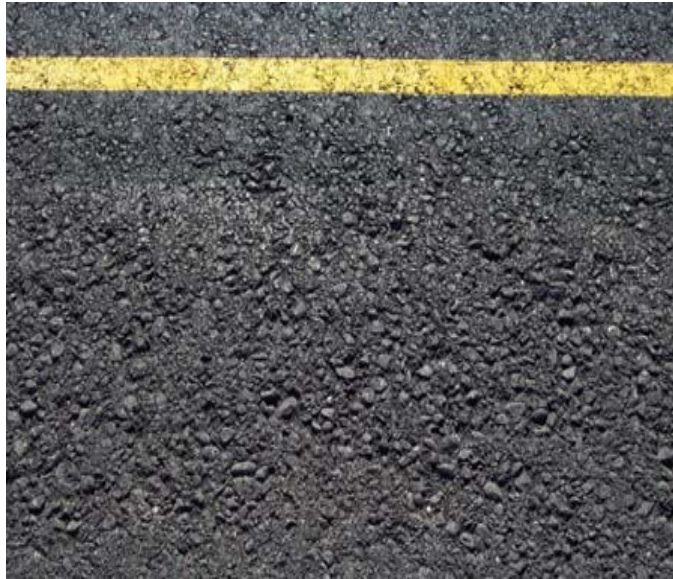
Figure 1-24 Segregation (HMA)
