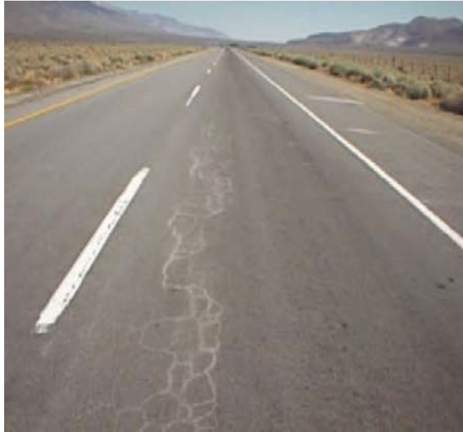
Figure 1-6 Fatigue Cracks
