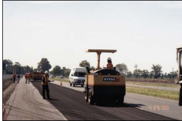
Figure 7-15 Pneumatic (Rubber Tired) Roller
