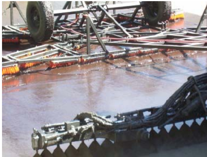
Figure 7-12 Scrub Seal Application
