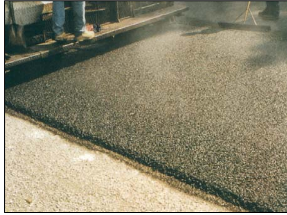
Figure 11-12 Freshly Laid BWC (Alvarez, 1992)
