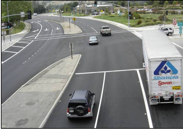
Figure 11-5 District 7 Rt. 103, BWC Gap Graded, Constructed in 2005
