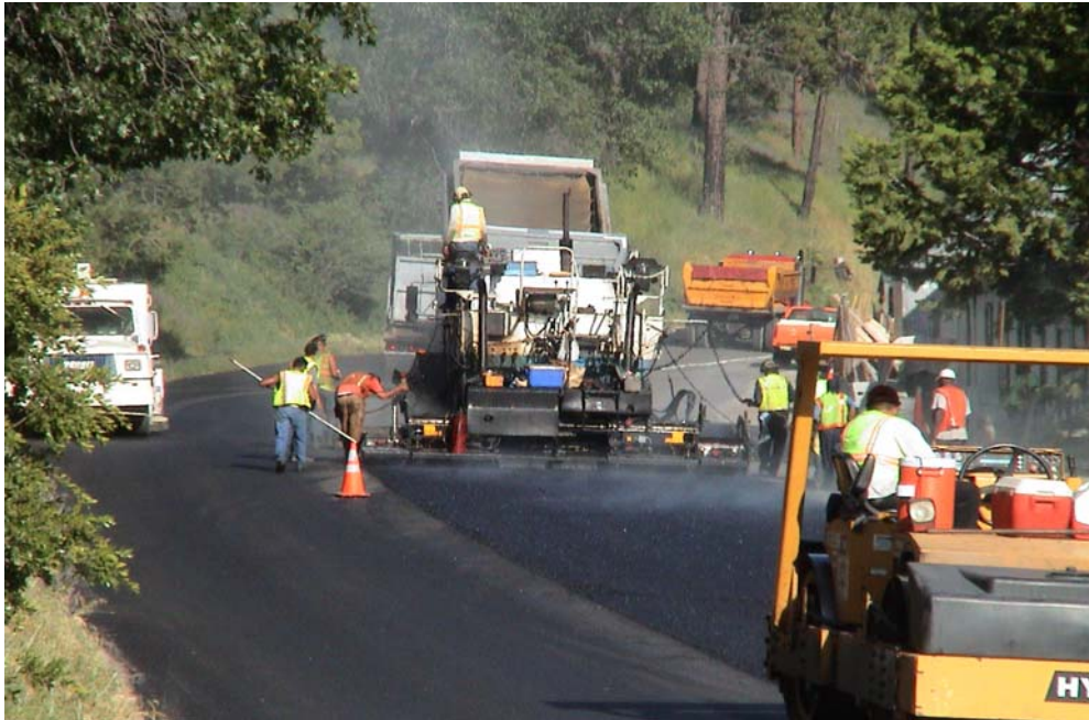
Figure 11-15 Roller Position During Application (Alvarez, 1992)
