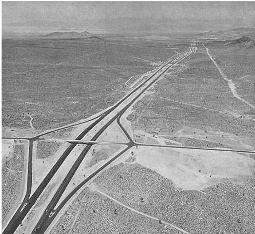
I-15 at Baker Grade (1961)
