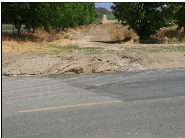
Access road drainage problems (note digout).
