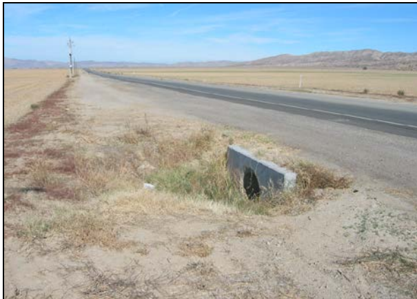
Blocked ditch and culvert.
