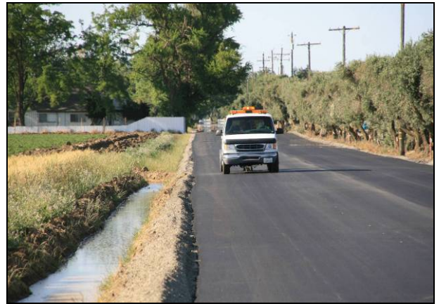
Side ditch used for irrigation water.
