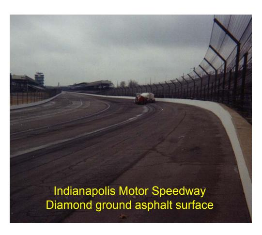
Asphalt pavement can be ground and grooved just like concrete pavement.
