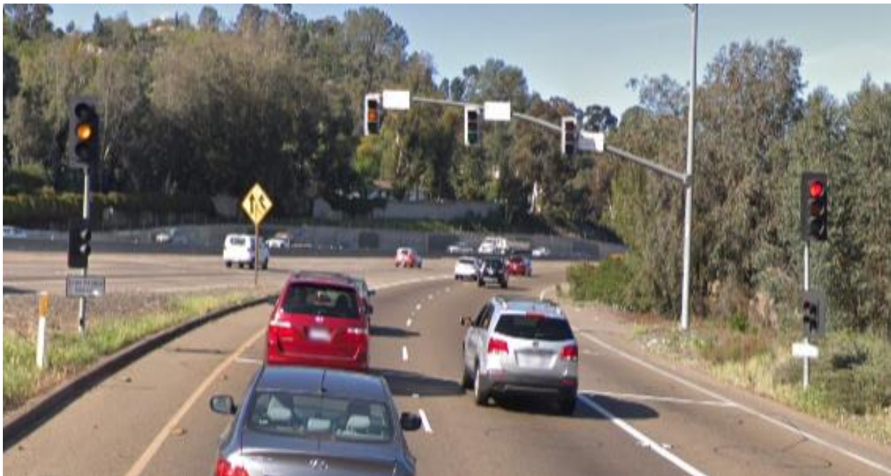
Metering system controlling preferential (HOV) lane
