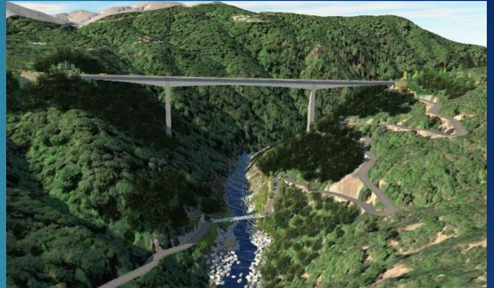
Mosquito Road Bridge 25C0061 – El Dorado County
