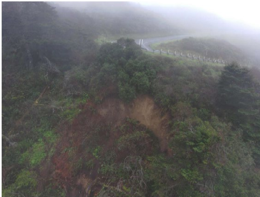
MEN-1-31.15: Head scarp of slide below upper road in switch back
