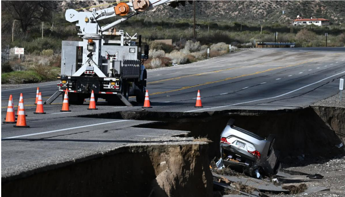
The skies cleared between storms on Thursday, but the damage remained on roads in California, including one in Phelan, Calif., northeast of Los Angeles. William Liang/Associated Press
