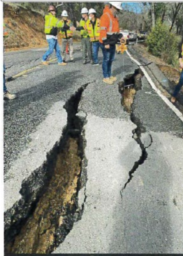
This Photograph Shows: NAP-121-PM 19.5- Slip out and roadway failure along the NB direction
