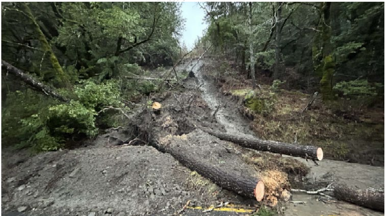
This Photograph Shows: NAP-121-PM 19.5- Slip out and roadway failure along the NB direction
