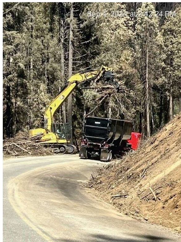
03-BUT-32 – Park Fire -typical Damages
