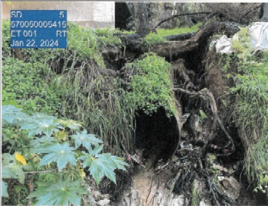
This Photograph Shows: Storm water running underneath the culvert instead of inside the culvert due to rusted invert at the culvert outlet.
