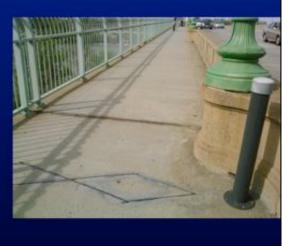
Mobile vs. permanent counters – permanent can only be used at one location, but the counters may provide more robust data.
