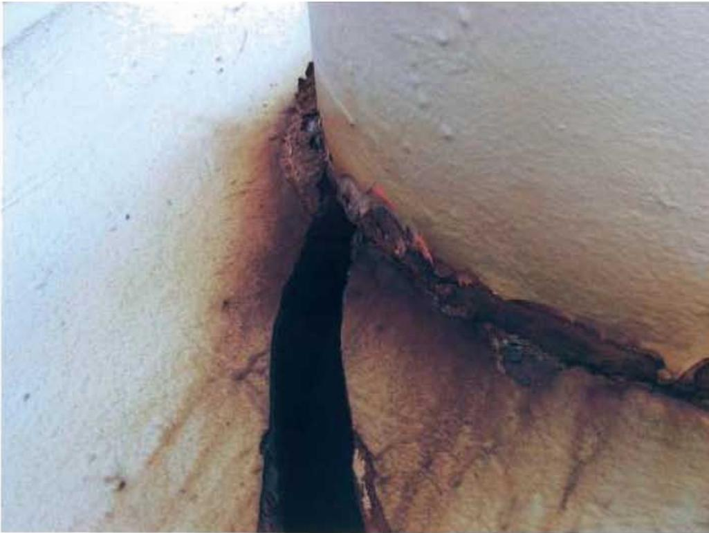
**Fig. 5 Corrosion at sleeve location at end of crack.**
