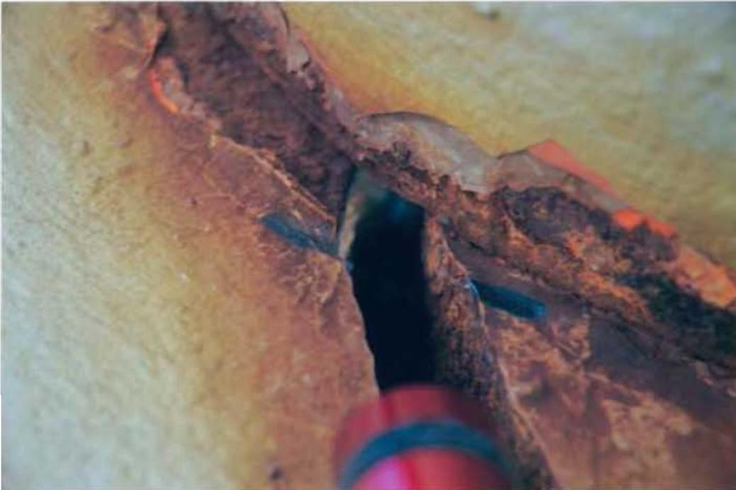
**Fig. 10 Corrosion at pin location.**
