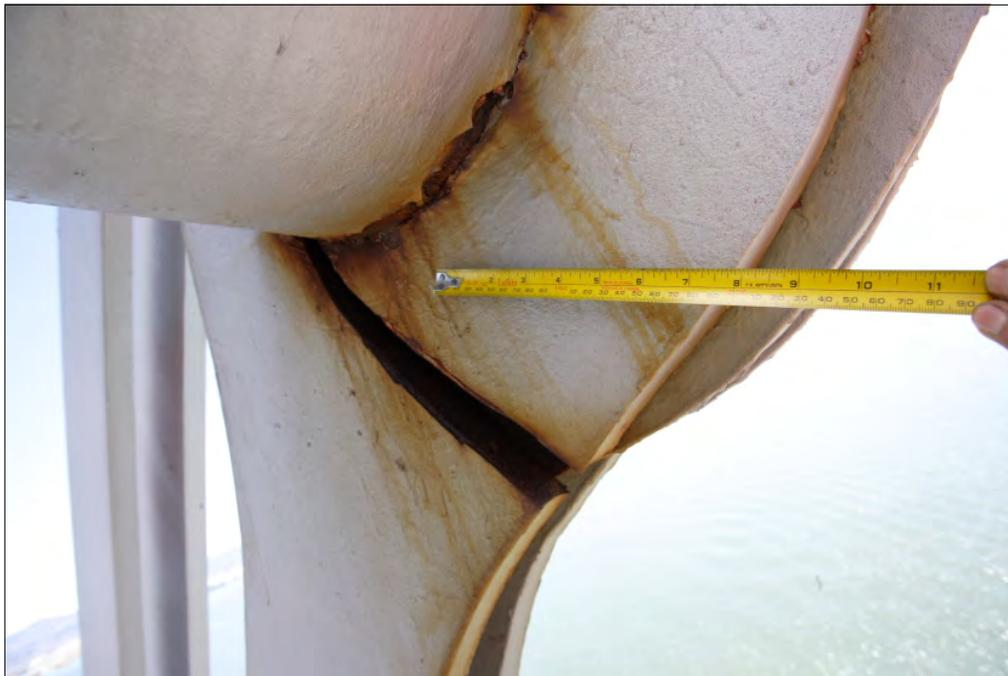
Figure 2: Eye bar showing failure location
