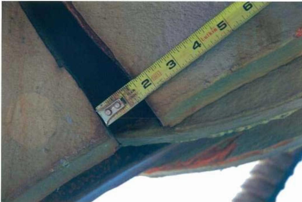
**Fig. 8 Crack opening displacement, outer edge.**
