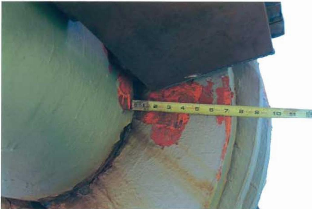
**Fig. 6 Eye bar above crack location.**
