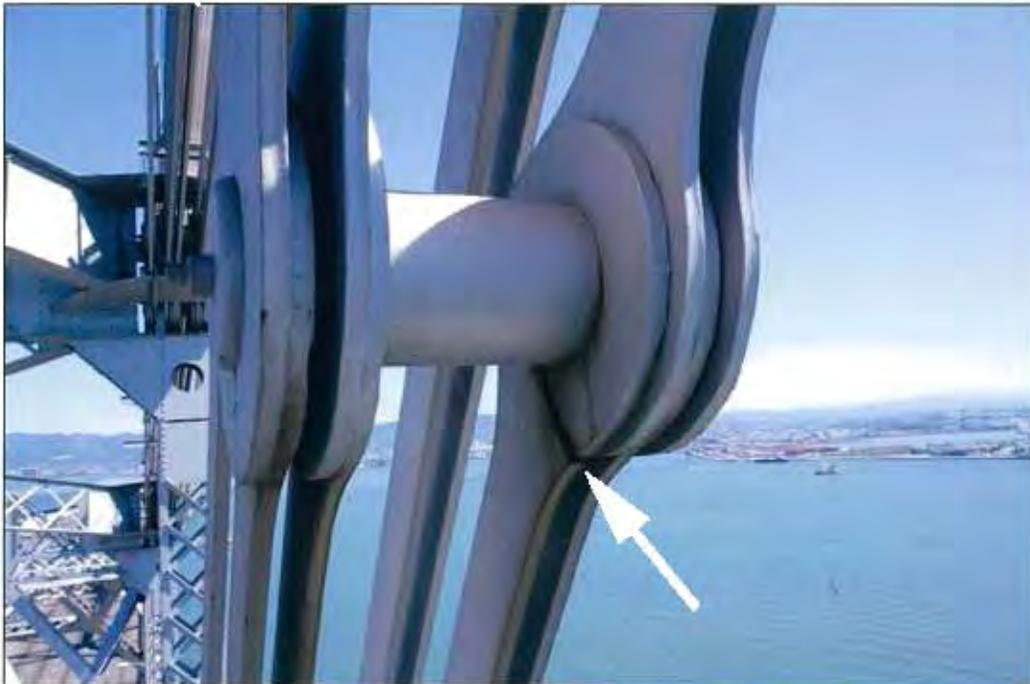
**Fig. 2 Location of cracked eye bar.
