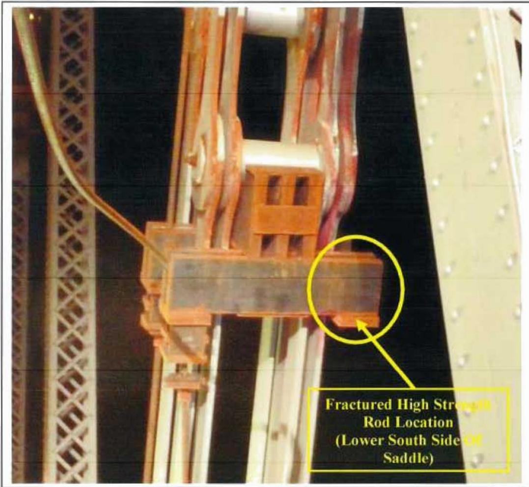
Fig. A Fractured Rod location.
