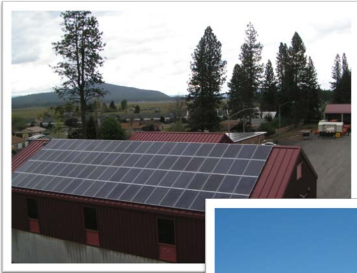
District 2 Burney Maintenance Station
