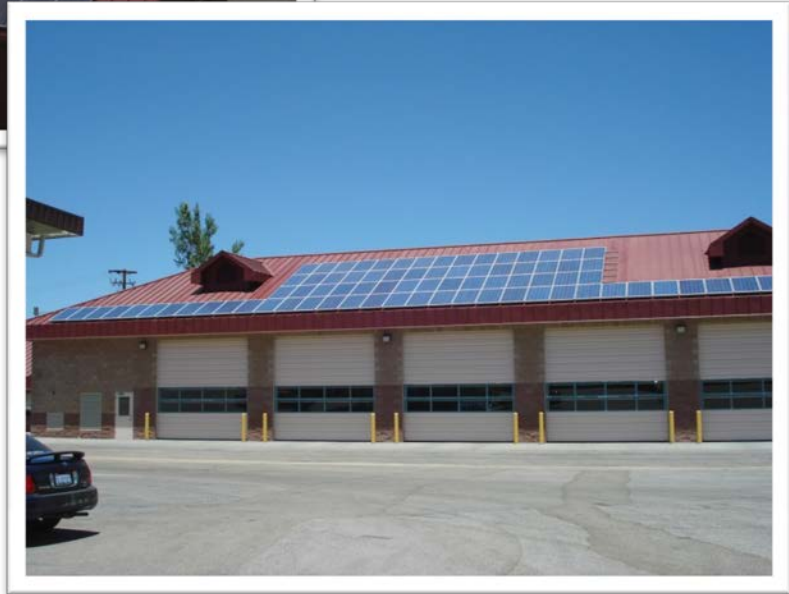
District 6 Lebec Maintenance Station
