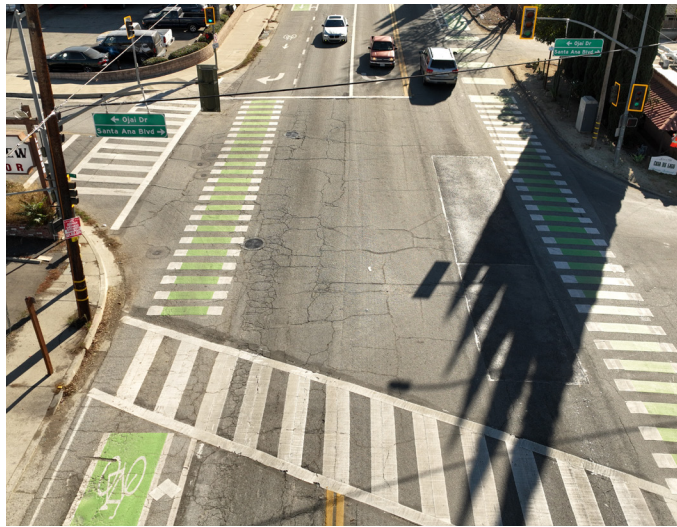
Figure 7: Buffered bike lanes and crosswalks at the intersection of State Route 33 and N. Ventura Avenue in Oak View, CA (District 7).
