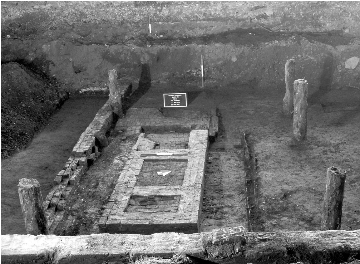
Figure 89. Engine Foundations, Stockton. Developed in a pressurized boiler, steam was piped to the engine where it was injected into a piston chamber that converted its expansion into energy. Steam engines developed strong vibrations due to the action of the piston and had to be securely bolted down to stop the engine from shaking itself from its foundation (Photograph by ASC, Sonoma State University).
