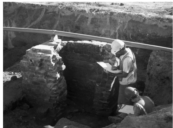
Figure 92. Brick furnace, Stockton's Sing Lee Laundry, operated 1890s–1930s. The business heated water in a boiler mounted above this brick furnace (Photograph by ASC, Sonoma State University).
