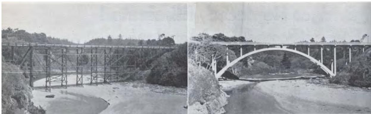
Figure 2: State Route 56 and Jug Handle Creek, Mendocino County, before and after new bridge constructed in 1939.
