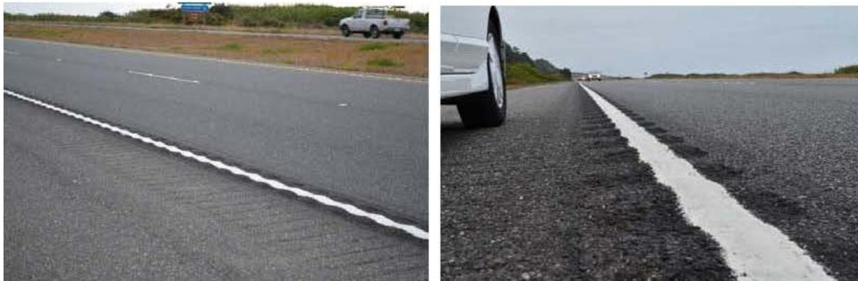
Figure 10: Photographs of mumbles installed on the southbound side of US Highway 101
