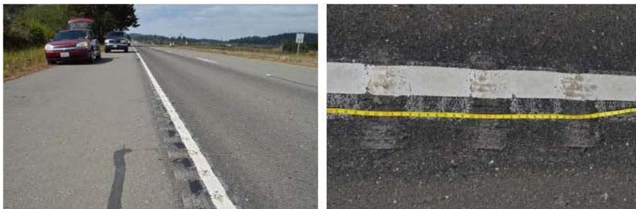
Figure 11: Photographs of ground rumble strips on State Route 299
