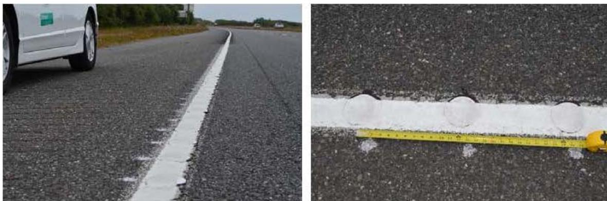
Figure 12: Photographs of Type A raised pavement markers (dots) installed on US Highway 101
