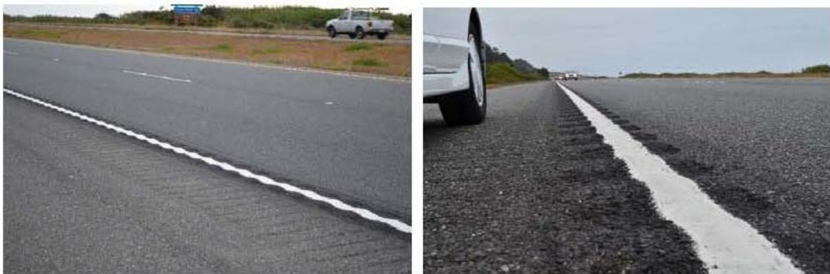
Figure 7: Photographs of mumble strips installed on US Highway 101
