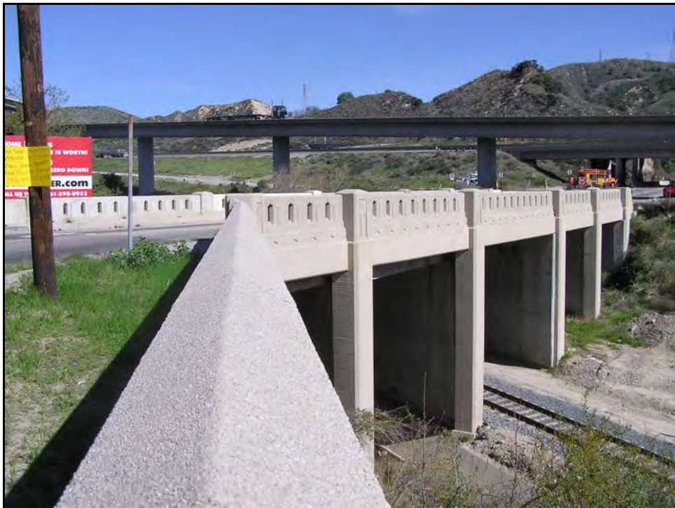
Photograph 4: South side, facing northeast, March 2004
