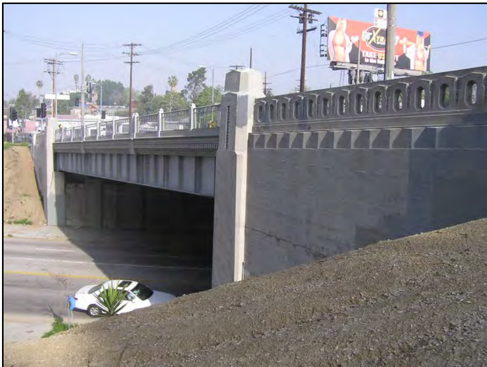
Photograph 2: Southwest side, facing north, March 2004
