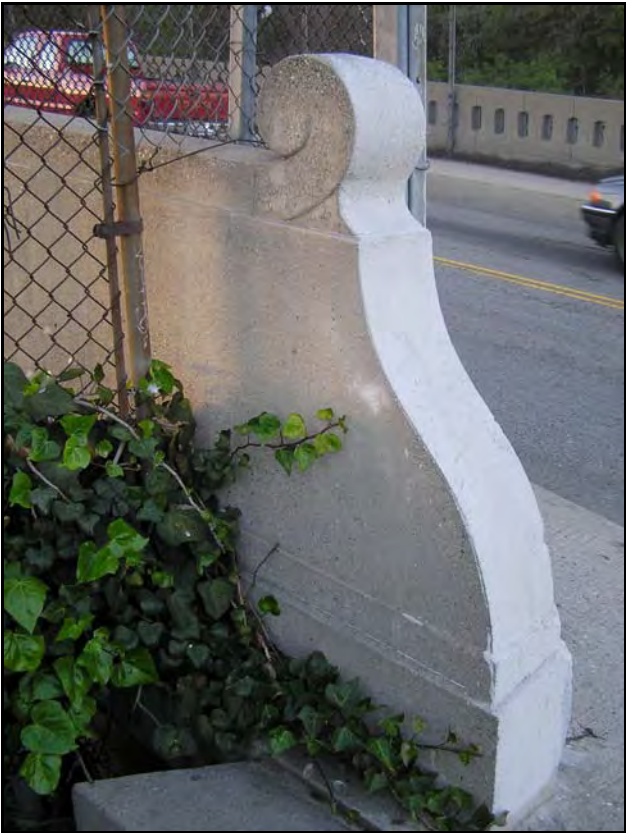
Photograph 4: South side, facing northwest, March 2004
