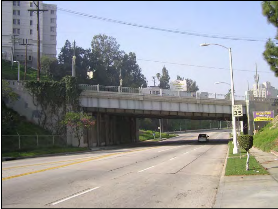
Photograph 1: Northeast side, facing west, March 2004
