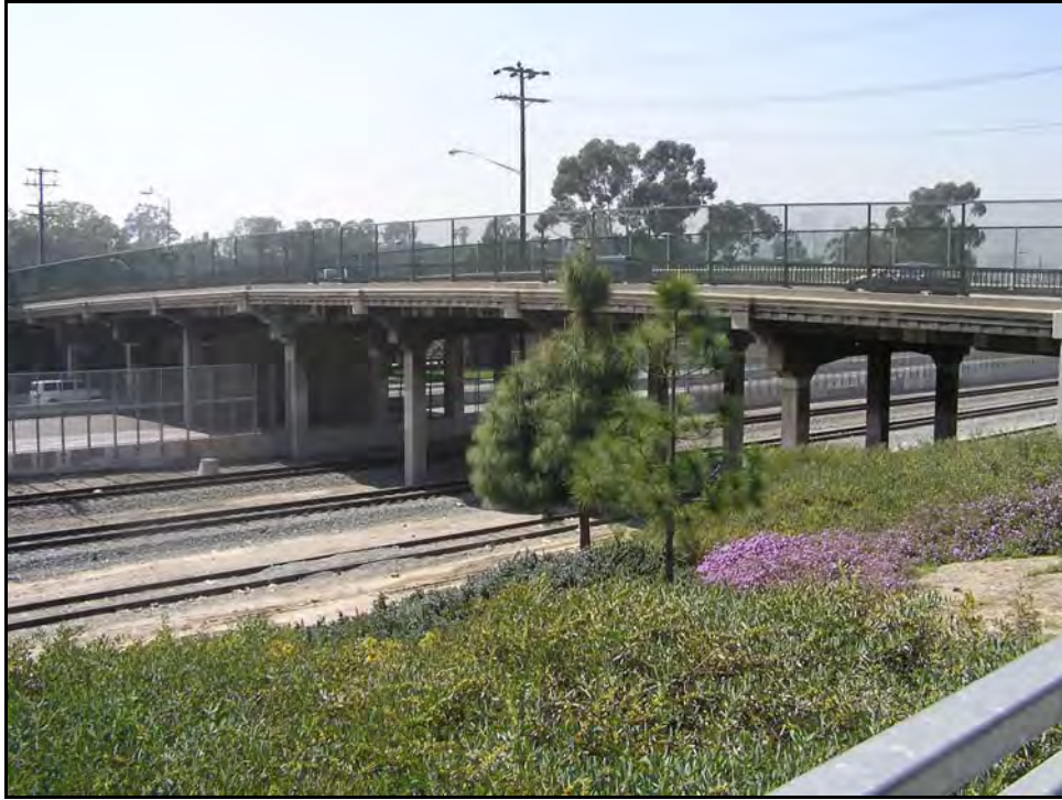
Photograph 1: West side, facing southeast, March 2004
