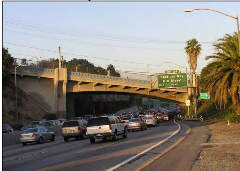
Photograph 1: Southwest side, facing north, March 2004
