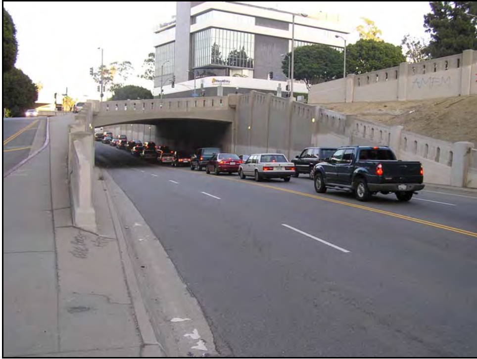
Photograph 1: South side, facing northwest, March 2004
