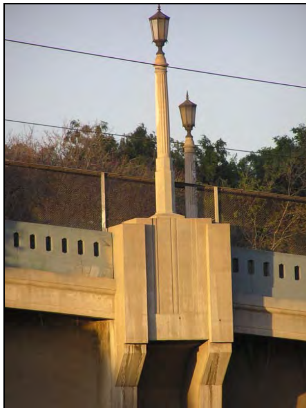
Photograph 2: Southwest corner, facing northwest, March 2004
