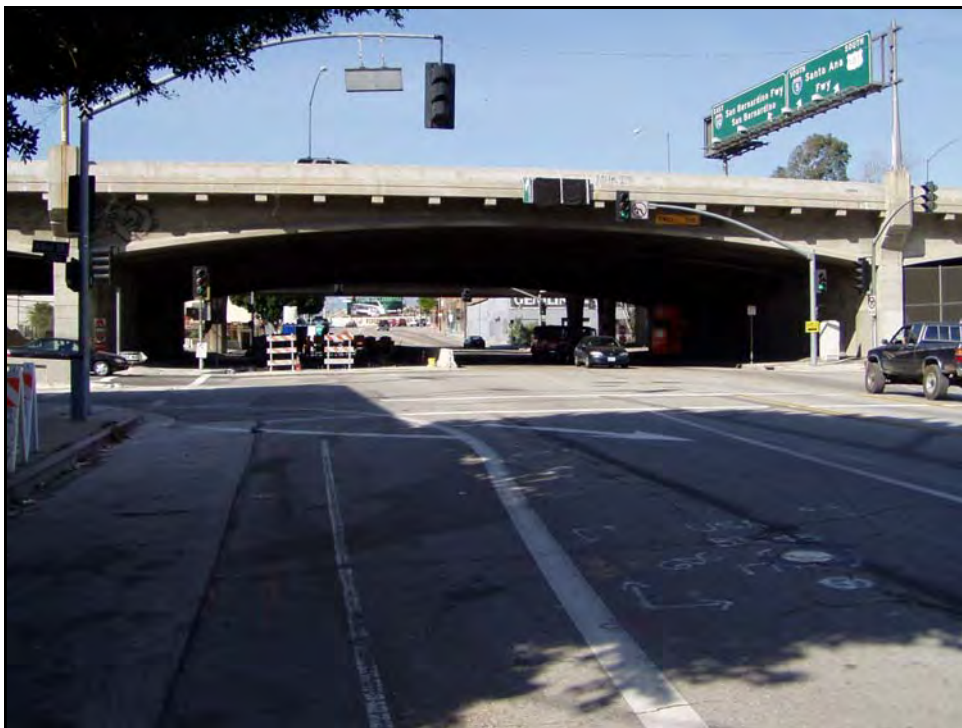
Photograph 4: Facing north on Mission Road, March 2003
