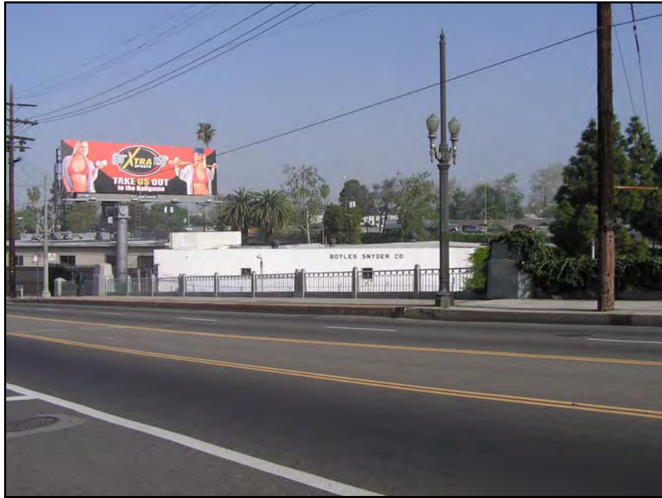
Photograph 3: Deck, Facing northeast, March 2004
