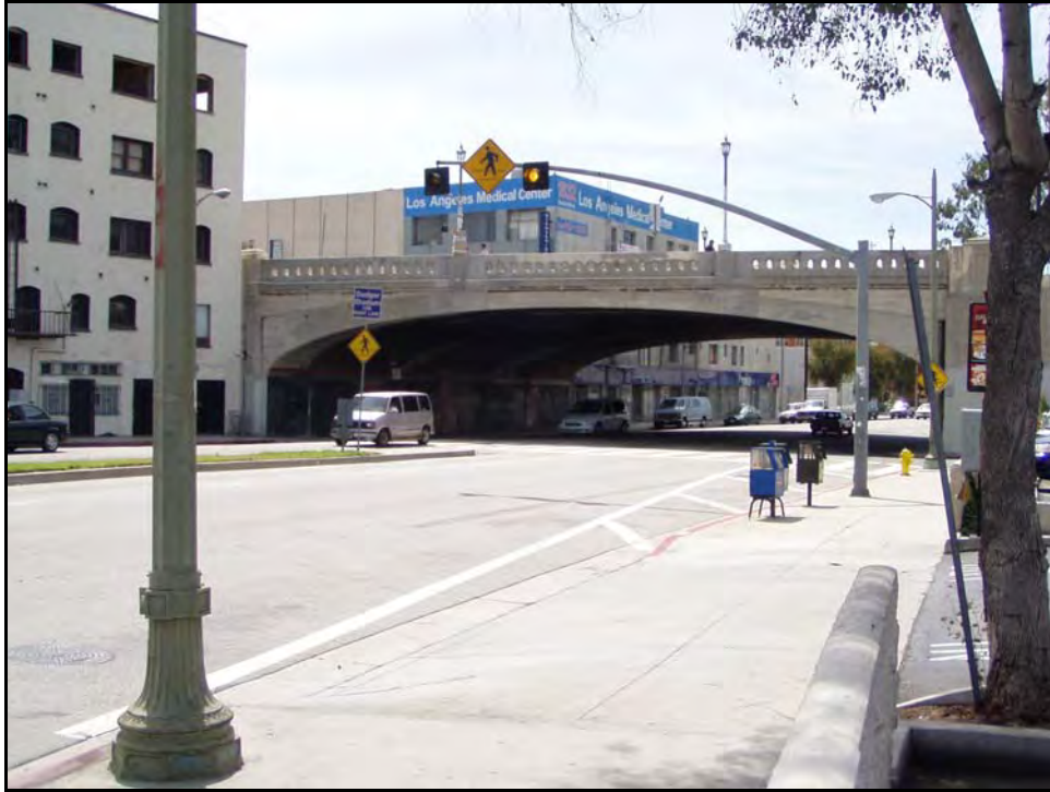
Photograph 1: Facing north, March 2003
