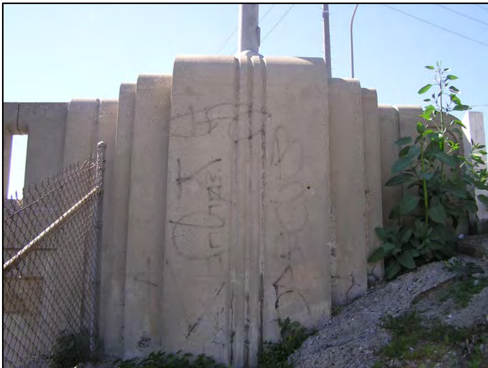
Photograph 4: Facing west, March 2004
