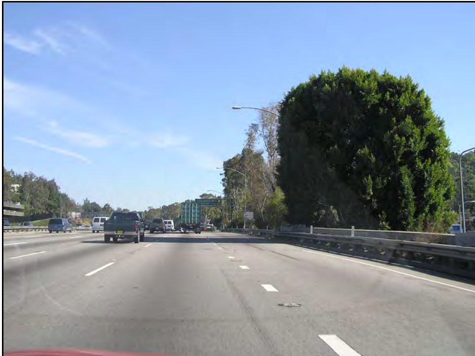
Photograph 2: East railing on deck, facing north, March 2004
