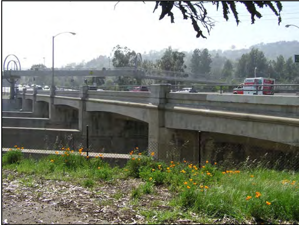
Photograph 1: South side, facing northwest, March 2004
