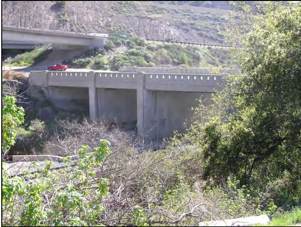
Photograph 1: North side, facing southeast, March 2004
