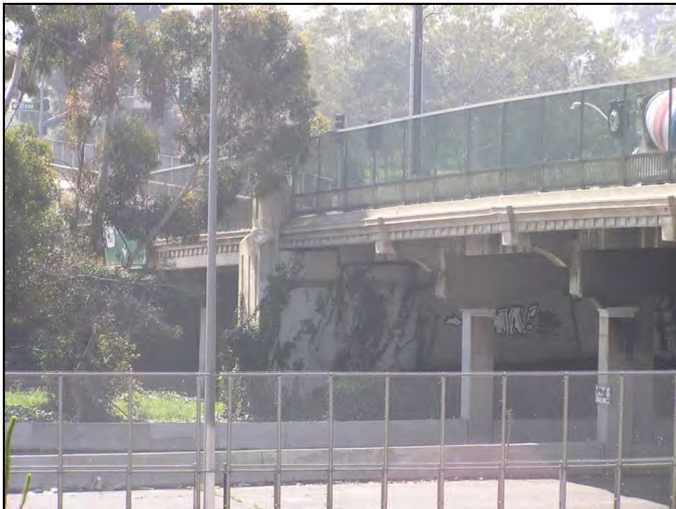
Photograph 2: West side, facing southeast, March 2004
