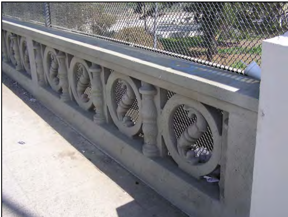
Photograph 4: West side railing, facing northwest, March 2004
