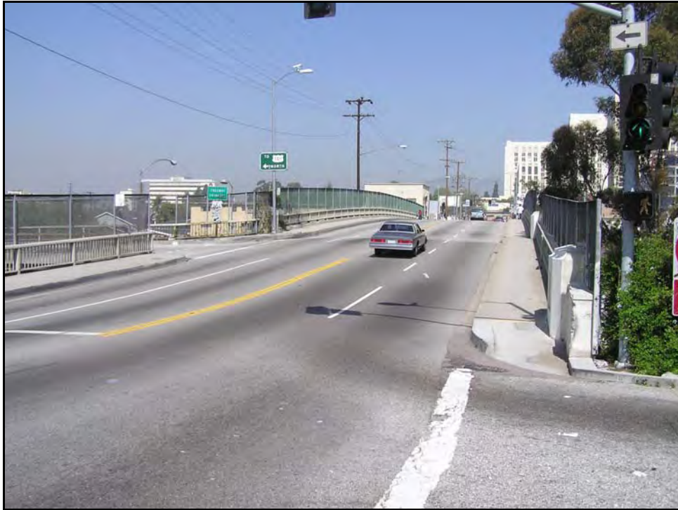
Photograph 3: Deck, facing north, March 2004
