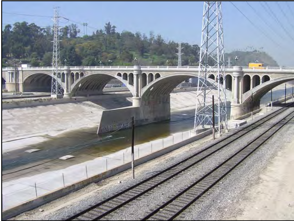
Photograph 1: East end, facing northwest, March 2004
