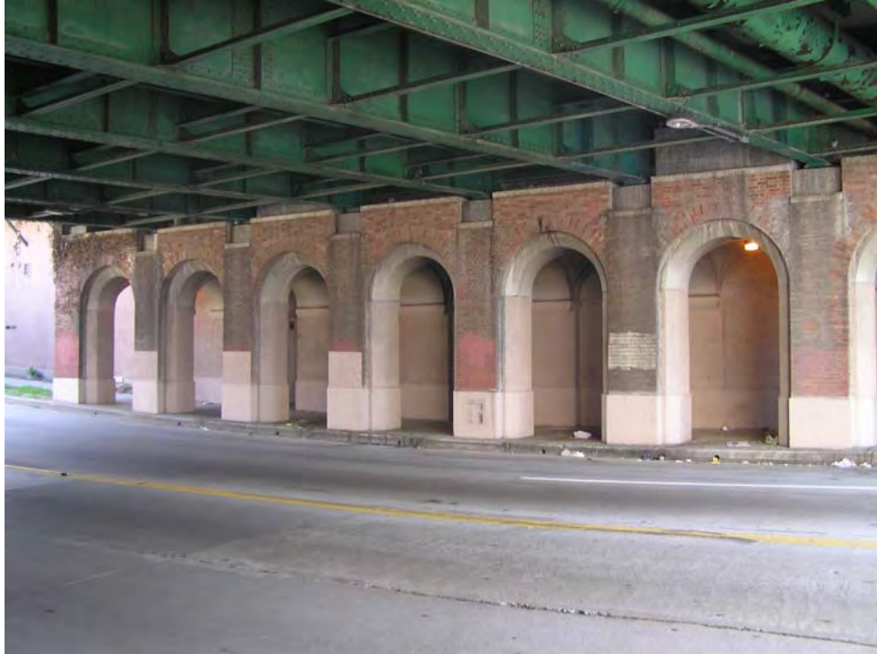
Photograph 3: Eastern walkway, facing east, March 2004
