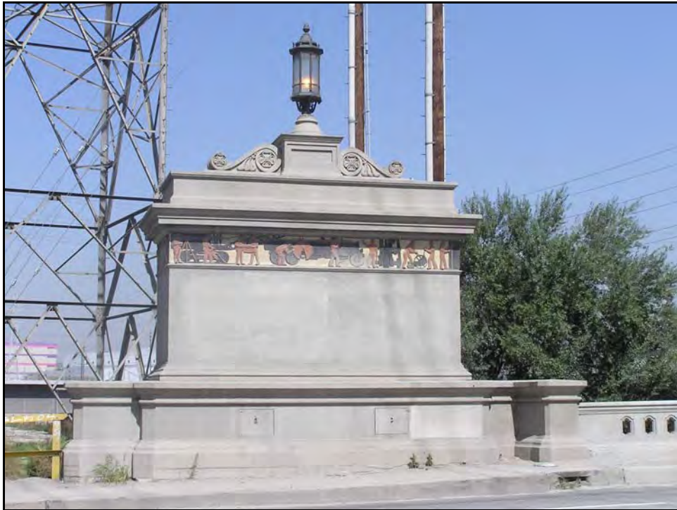
Photograph 3: facing north, March 2004
