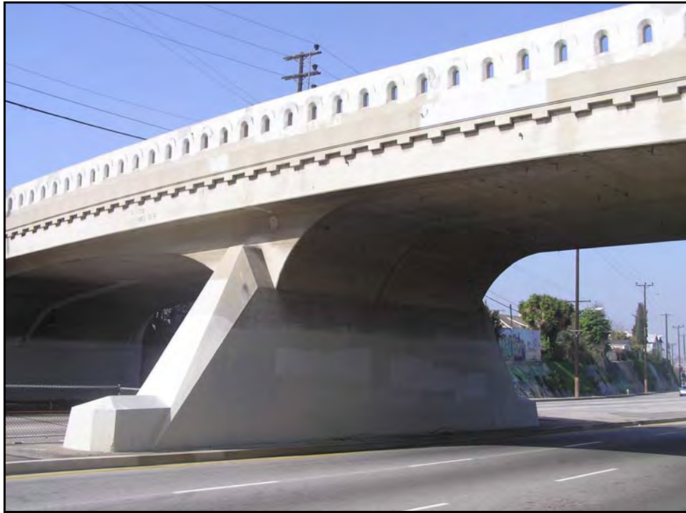
Photograph 5: Center pier, facing south, March 2004
