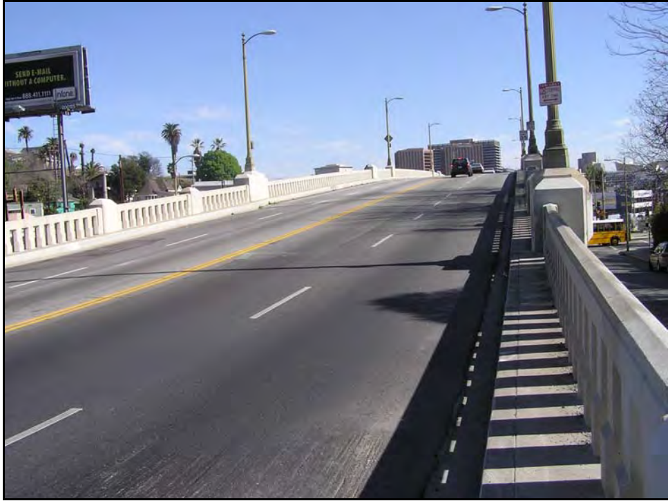
Photograph 5: Deck, facing southeast, February 2004
