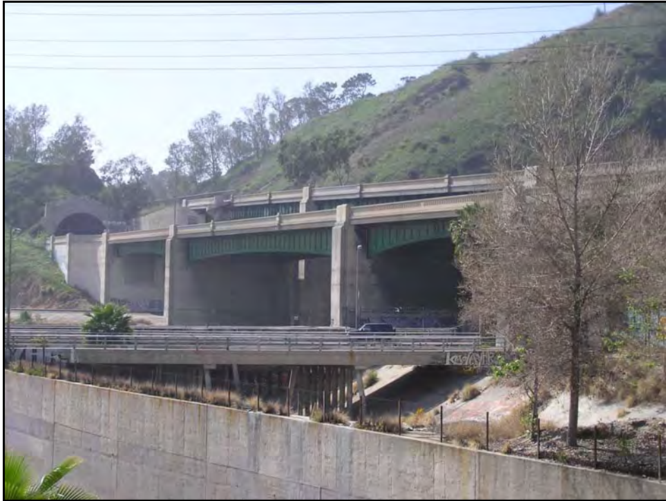
Photograph 1: West end, facing northwest, March 2004
