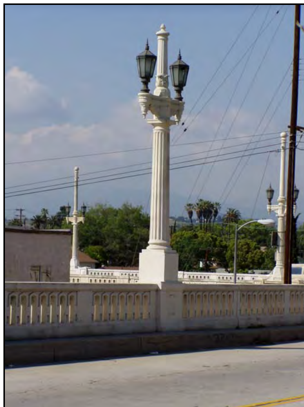
Photograph 4: Facing southwest, April 2003
