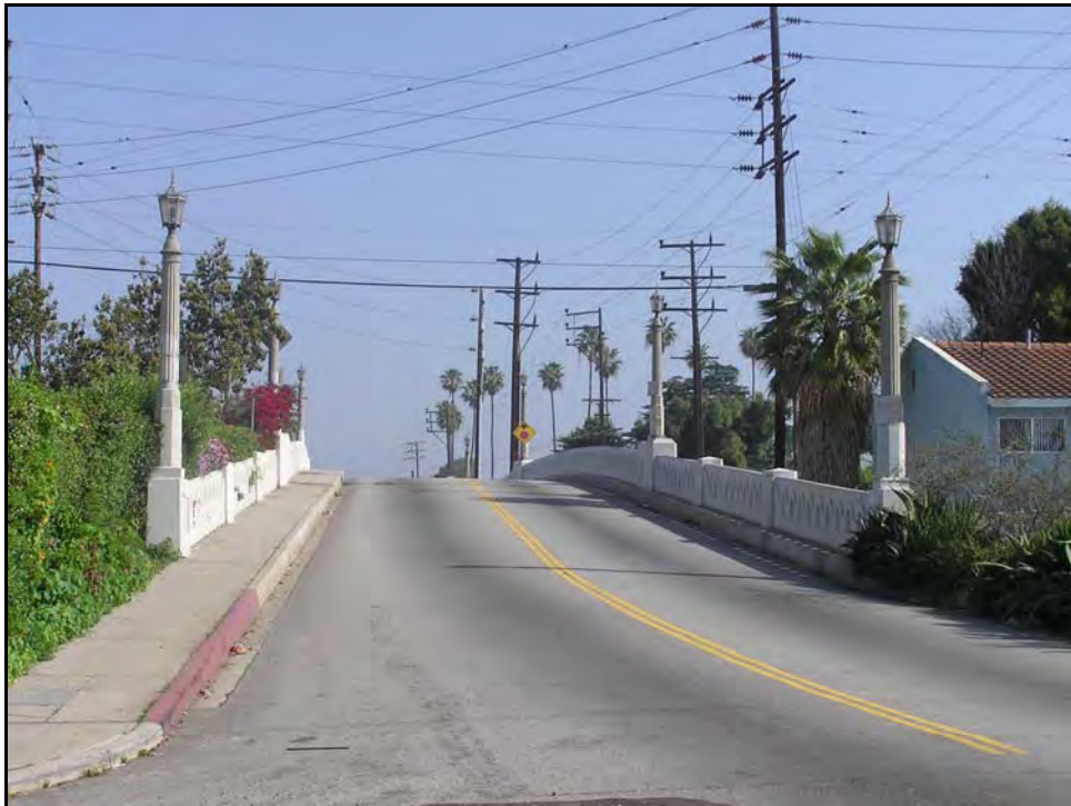
Photograph 2: Deck, facing north, March 2004
