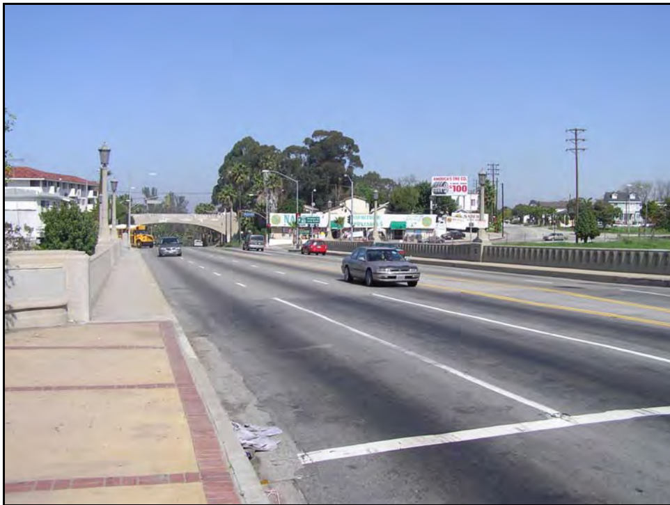
Photograph 2: Deck facing north, March 2004
