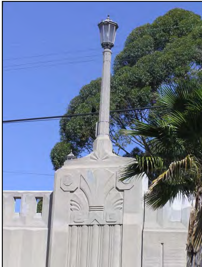
Photograph 4: Facing north, March 2004
