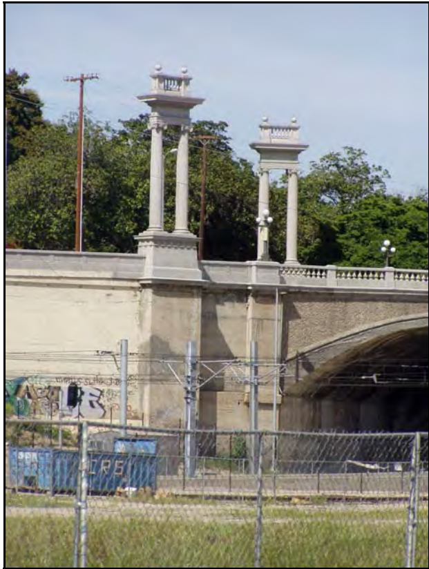
Photograph 3: Facing north, March 2003
