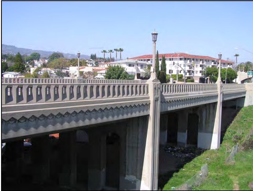
Photograph 1: East side, facing north, March 2004
