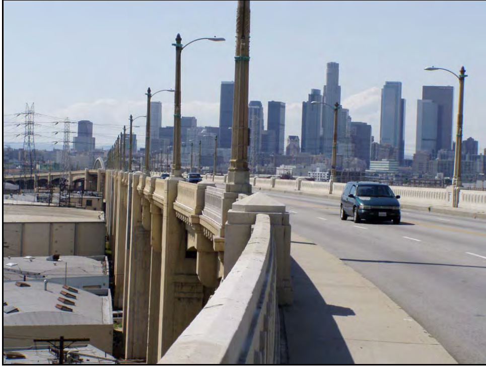
Photograph 5: Deck, facing west, April 2003
