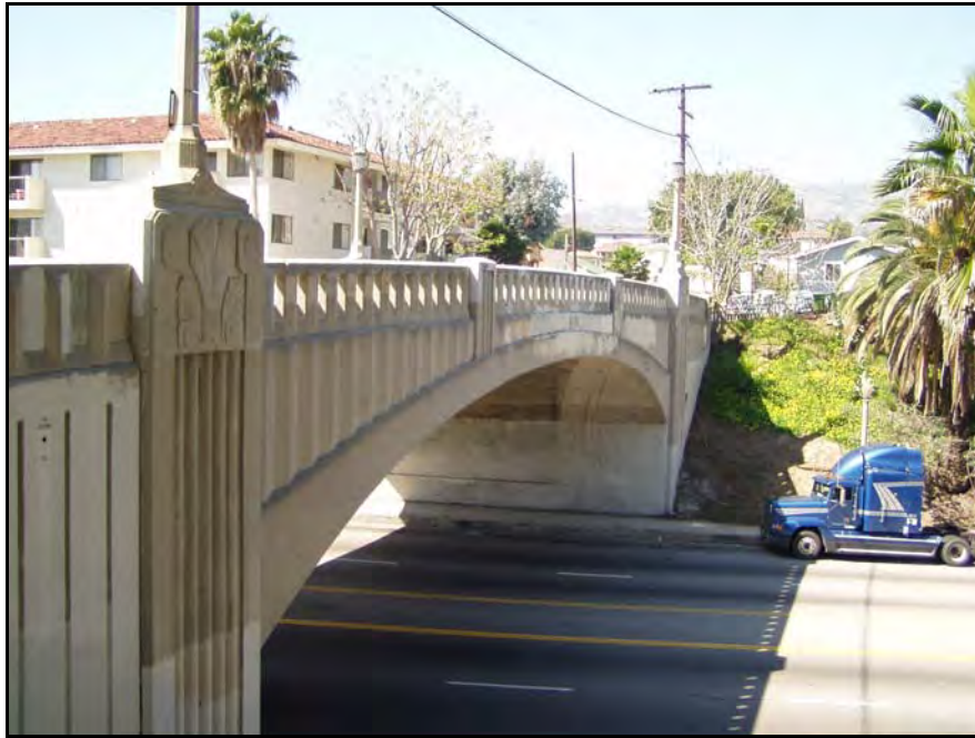
Photograph 3: Facing west, March 2003
