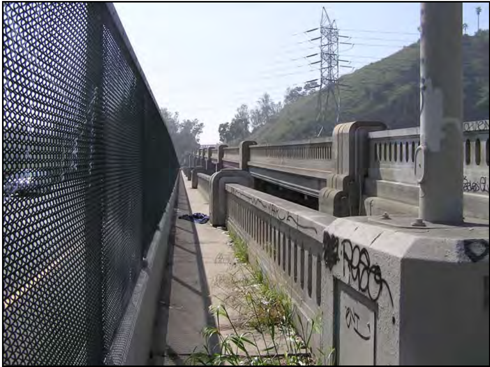
Photograph 3: North railing, facing west, March 2004
