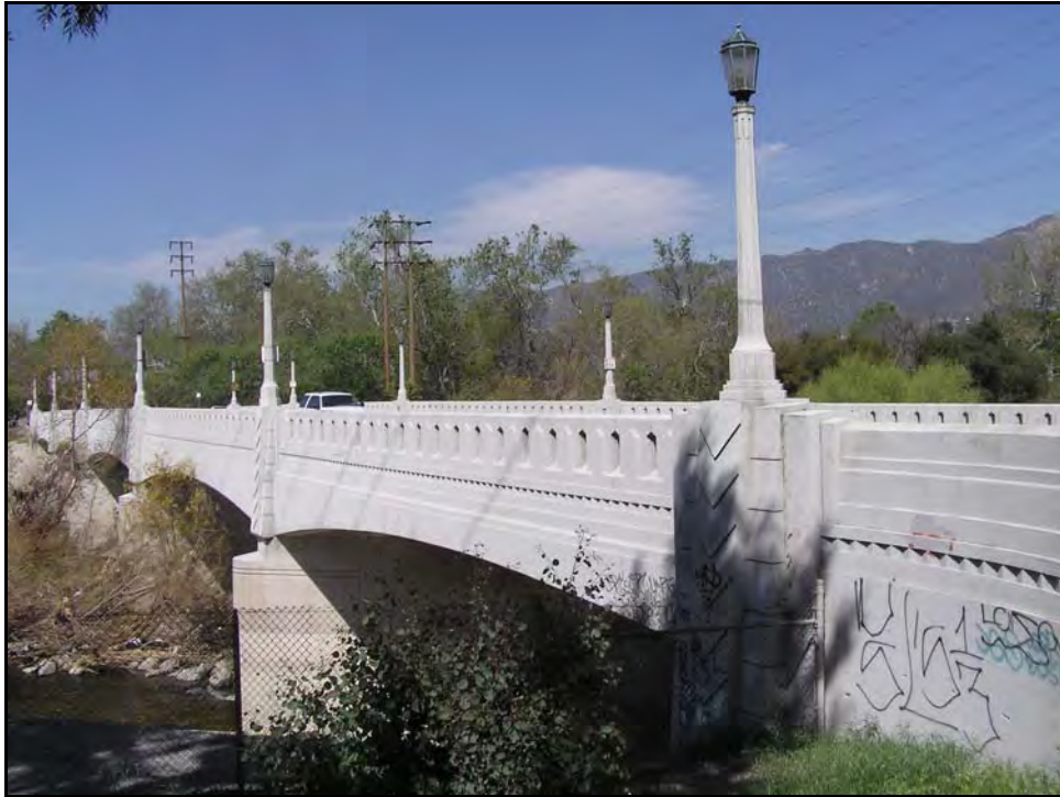
Photograph 1: North side, facing southeast, March 2004
