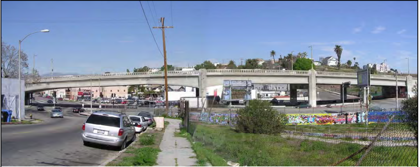
Photograph 1: South side, facing north, March 2004
