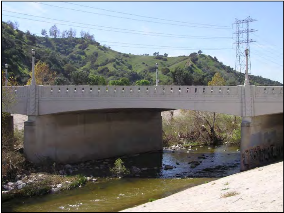
Photograph 3: South side, facing north, March 2004
