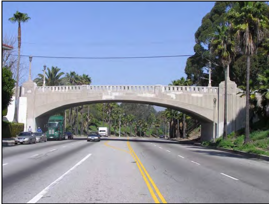
Photograph 1: Facing north, March 2004
