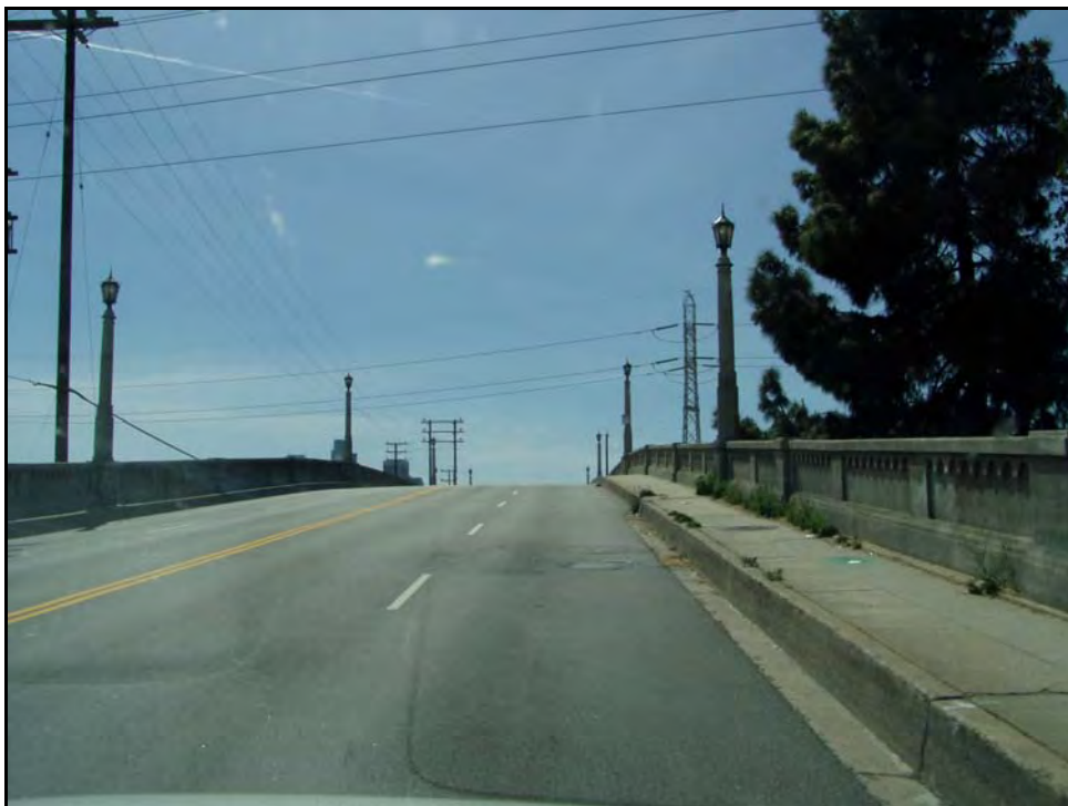
Photograph 2: Facing west, March 2003
