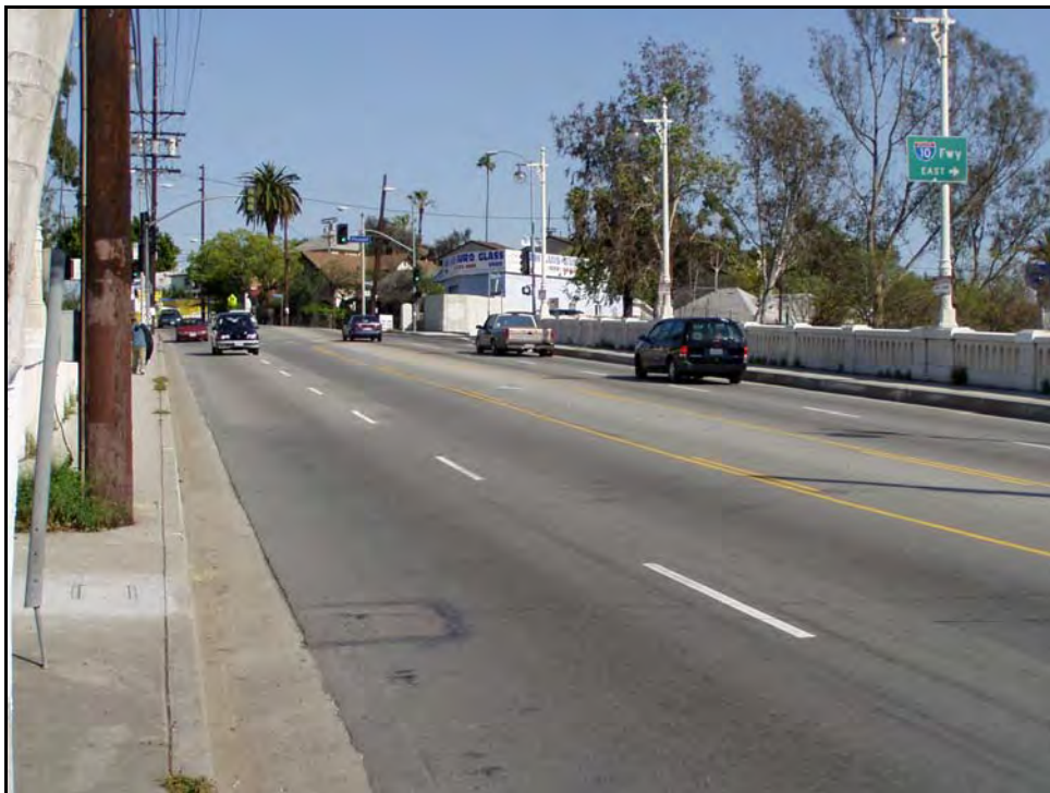
Photograph 2: Deck, facing east, April 2003
