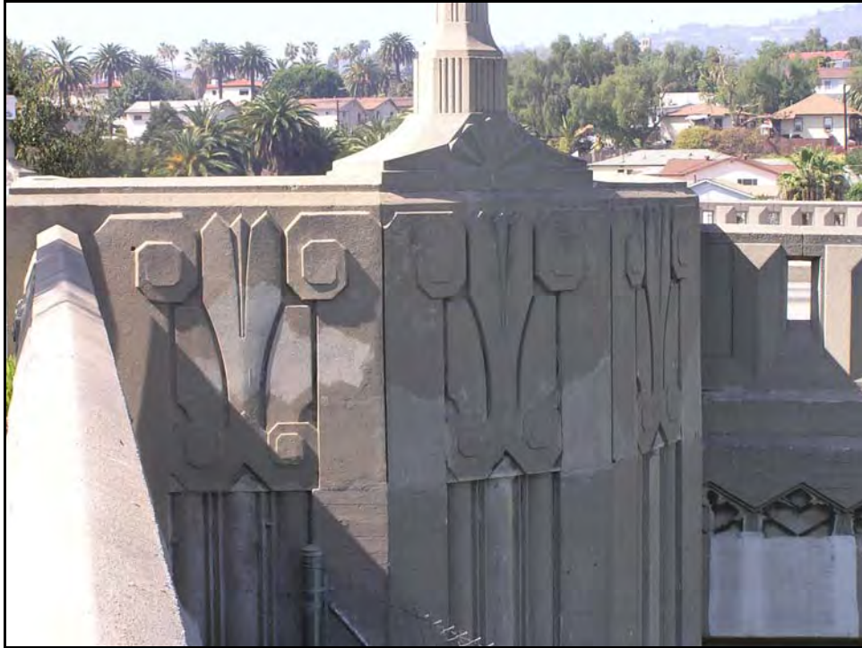
Photograph 3: Southeast corner, facing west, March 2004
