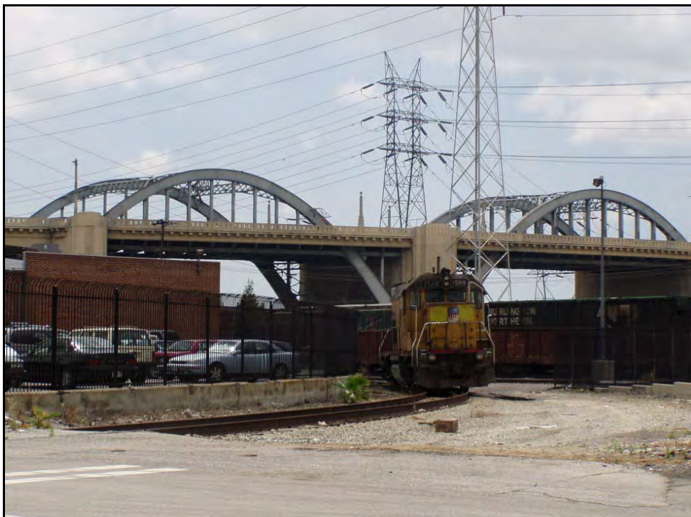
Photograph 2: Facing southwest, April 2003
