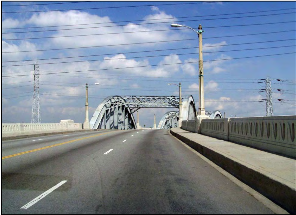
Photograph 3: Deck, facing west, April 2003
