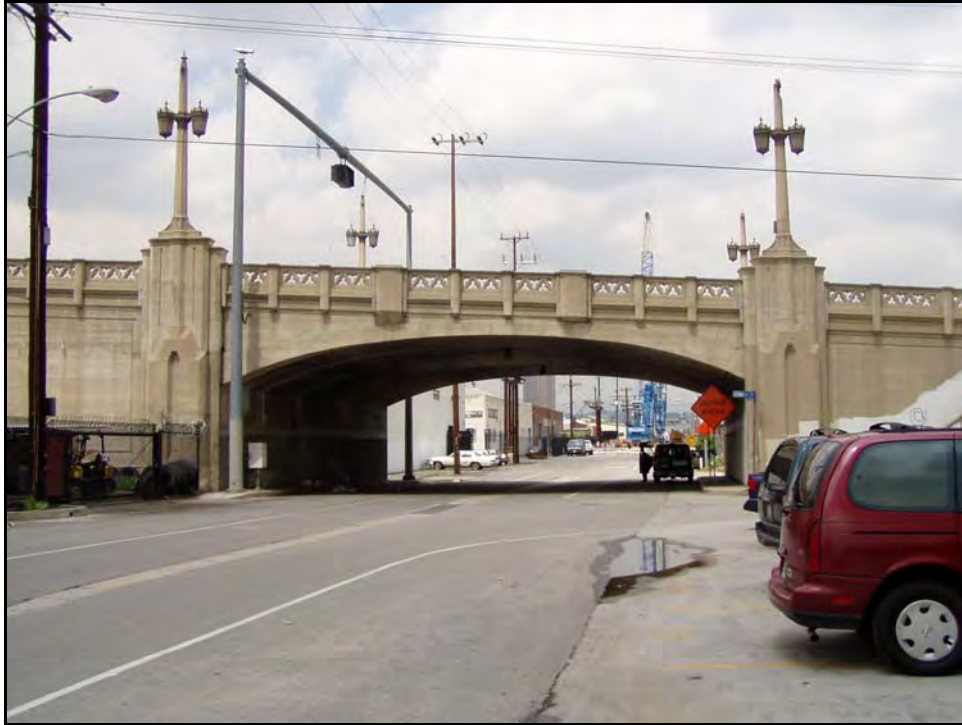
Photograph 3: East end, facing north, April 2003
