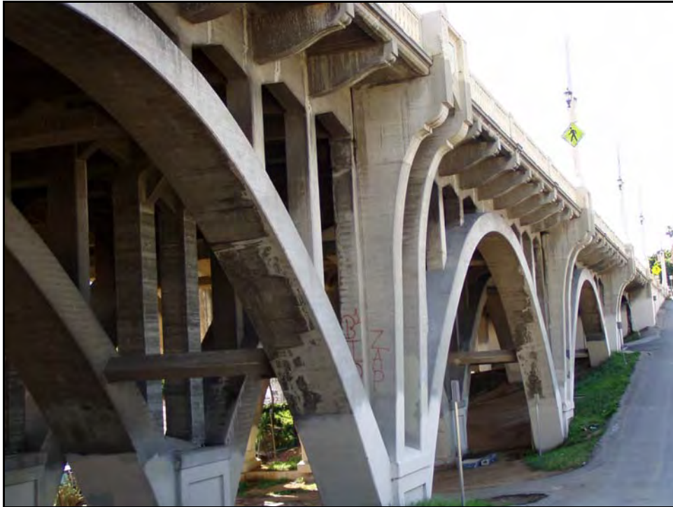
Photograph 1: Facing southwest, April 2003
