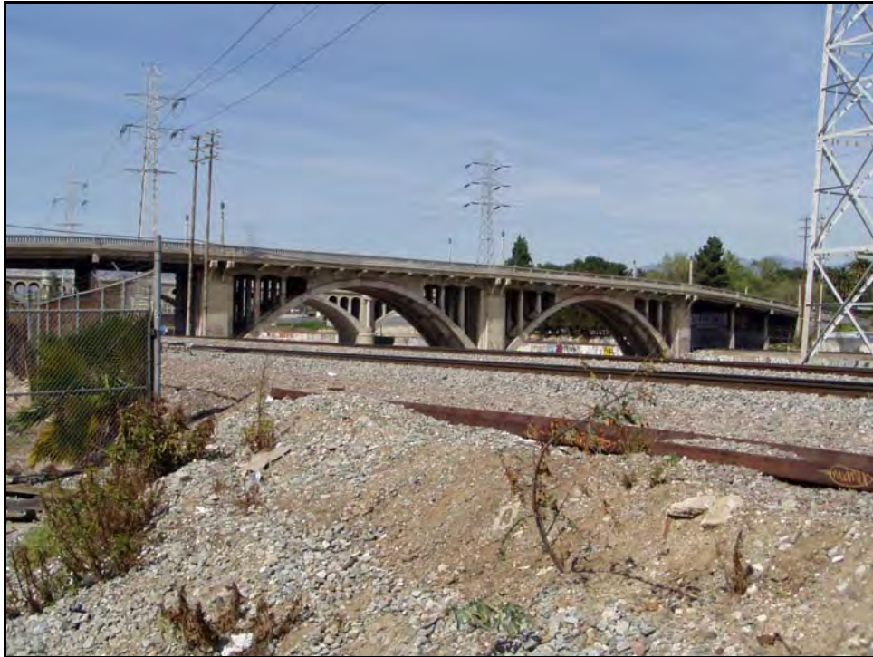
Photograph 1: Facing north, March 2003
