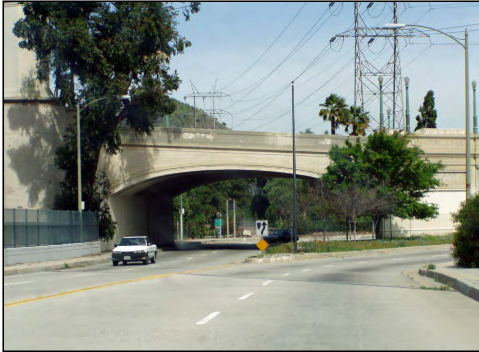
Photograph 1: Facing north, March 2003
