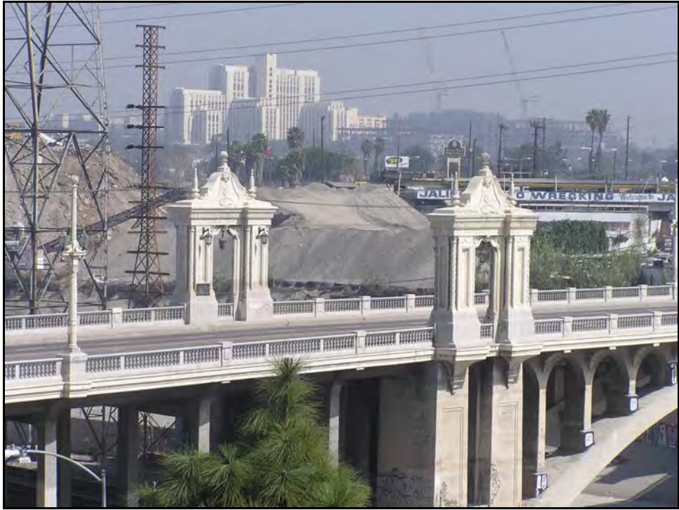
Photograph 3: Facing north, March 2003
