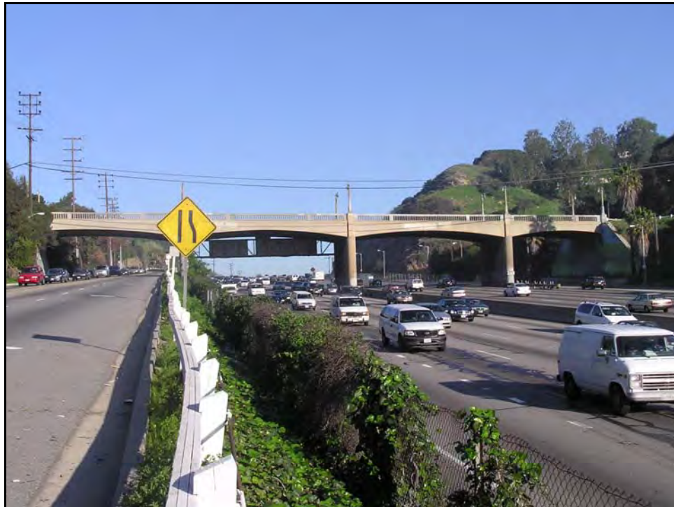
Photograph 1: South side, facing north, March 2004
