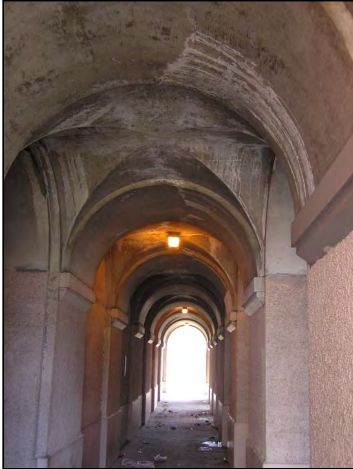
Photograph 5: western walkway, facing north, March 2004
