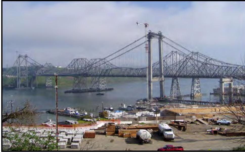
Photograph 4: Carquinez Strait Bridges (23 0015L and 23 0015R), built 1927 and 1958, with new suspension bridge in foreground. February 2003.
