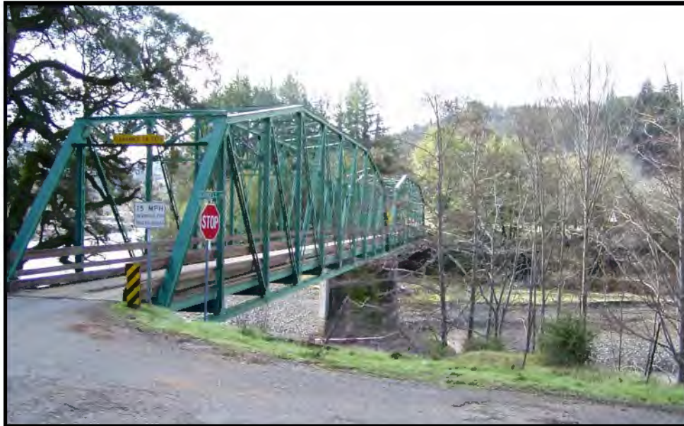
Photograph 8: Mattole River Bridge (04C0055), Mattole Road, built 1920. Example of a Camelback truss. February 2003.
