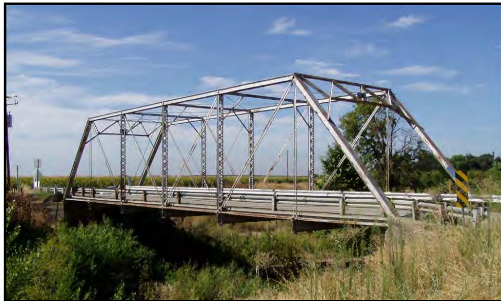
Photograph 6: Butte Creek Bridge on Durnell Road (12C0023), built in 1904. Example of a Pratt truss. August 2003.
