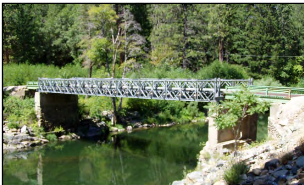
Photograph 11: Rich Bar Road Bridge (09C0041) built over the East Branch of the North Fork of the Feather River in 1951 using abutments and piers from previous bridge built in 1932. Example of a Bailey truss. August 2003.
