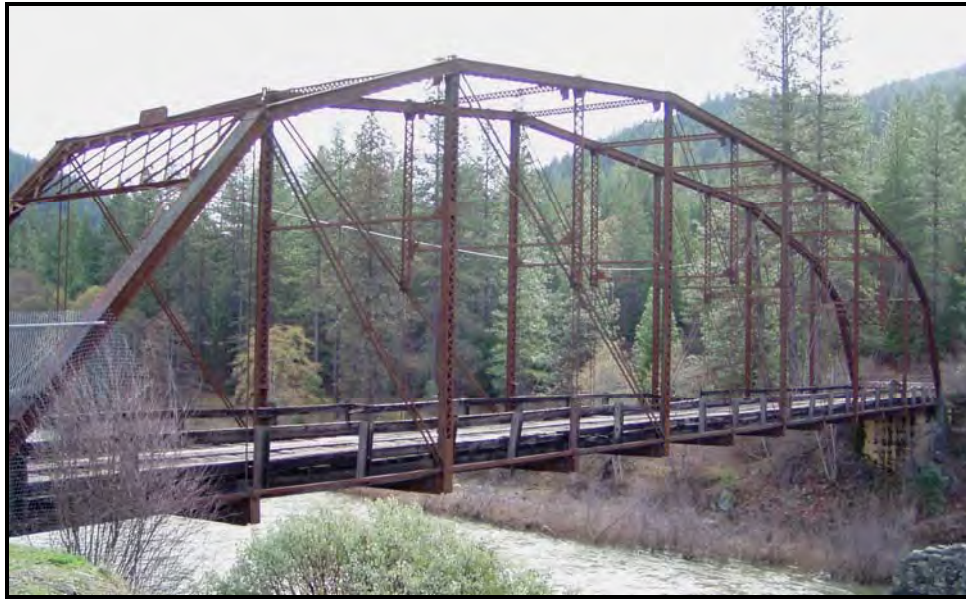
Photograph 10: Scott River Bridge (02C0021), Roxbury Drive, built 1915. Example of a Pennsylvania Petit truss. January 2003.
