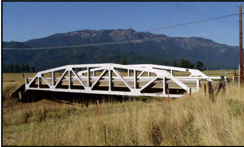
Photograph 5: Lights Creek Bridge (09C0012) on Beckwourth-Greenville Road, built 1947. Example of a Warren truss. August 2003.
