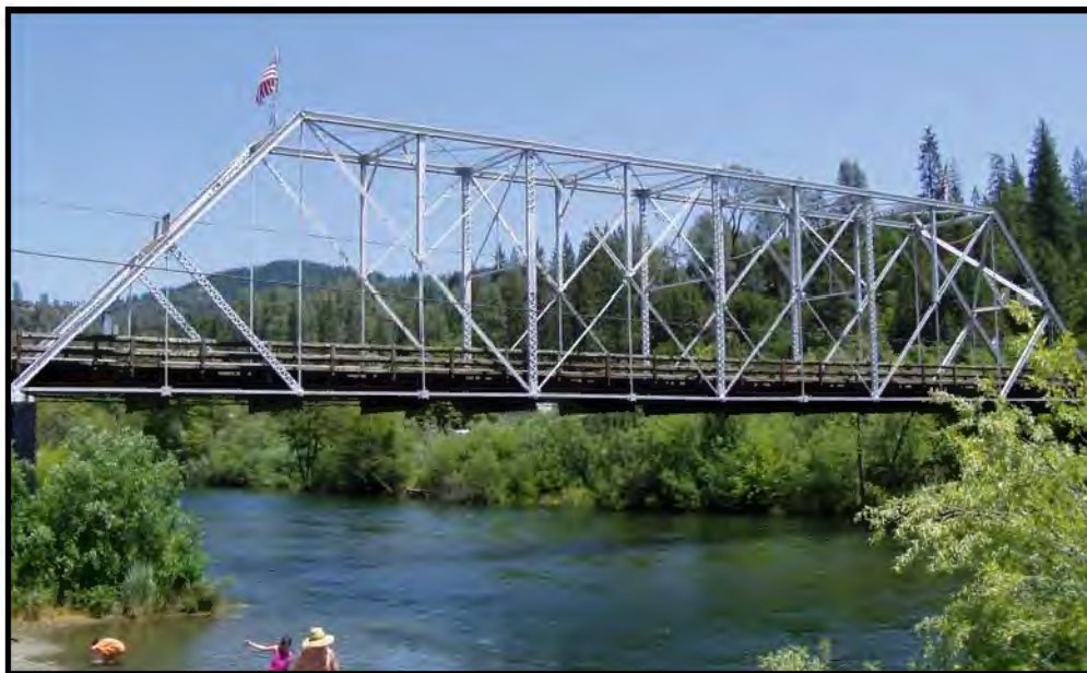
Photograph 9: Lewiston Bridge (05C0032), Turnpike Road over the Trinity River, built 1901. Example of a Baltimore Petit truss. June 2003.
