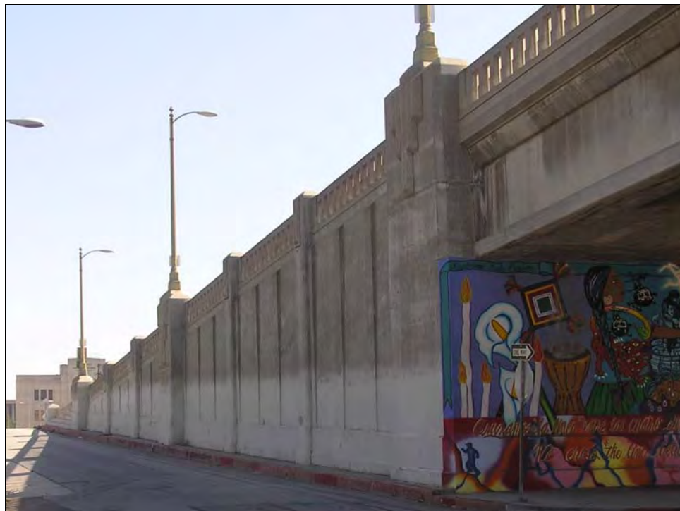
Photograph 4: Glendale Blvd.-Beverly Blvd. Separator (53C0045): Moderne Details
