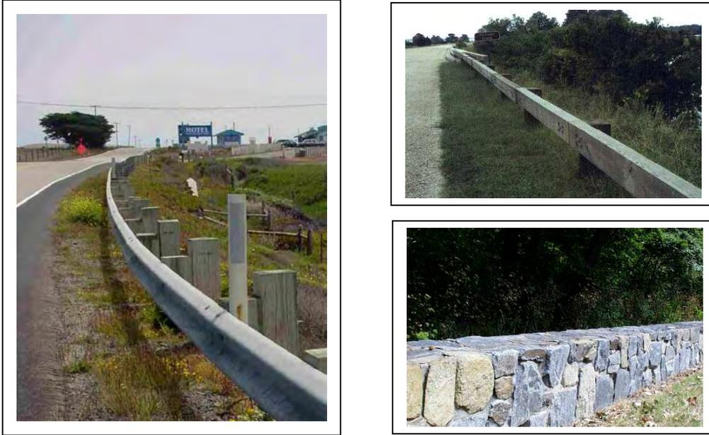
*Figure 20: On the left is a typical example of a galvanized metal beam guardrail that is used extensively along Highway 1 and is among the most common type used along highways throughout the United States. The timber guardrail (above right) is an alternative that could be considered for applications on the Big Sur Coast. The stone masonry guardwall (below right) is not yet available for use in California, but is being reviewed for acceptance in certain applications.*
