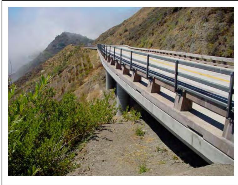
*Figure 11: The Forest Boundary side-hill viaduct completed in 2001. Built to pass over an area of slope instability, the viaduct is typical of major new structures that must be integrated with the historic fabric of Highway 1.*
