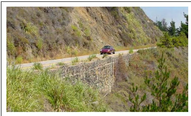
*Figure 17: A stone masonry retaining wall topped by a castellated type of stone parapet, typical of the historic rubble masonry along Highway 1.*
