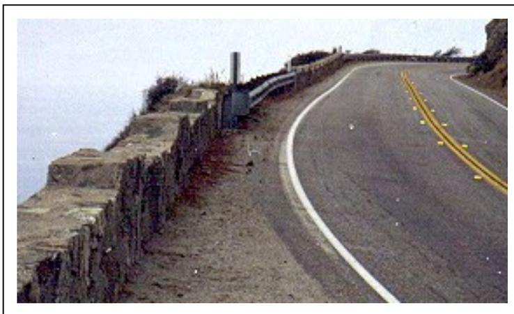
*Figure 18: A contemporary metal beam guardrail spans an original gap between two historic stone masonry parapets (atop retaining walls). At other locations, metal beam guardrail has been placed in front of rock wall sections (i.e., between the road and the wall).*
