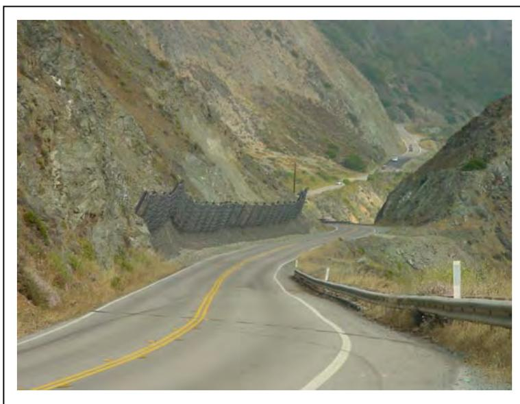
*Figure 15: A rocknet installation at Cow Cliffs prevents falling debris from reaching the road. Accumulated rock debris is periodically removed as part of maintaining the system. The raw nature of these sites, and the ingenuity required to keep the road open, is also part of the living character of Highway 1 along the Big Sur Coast.*
