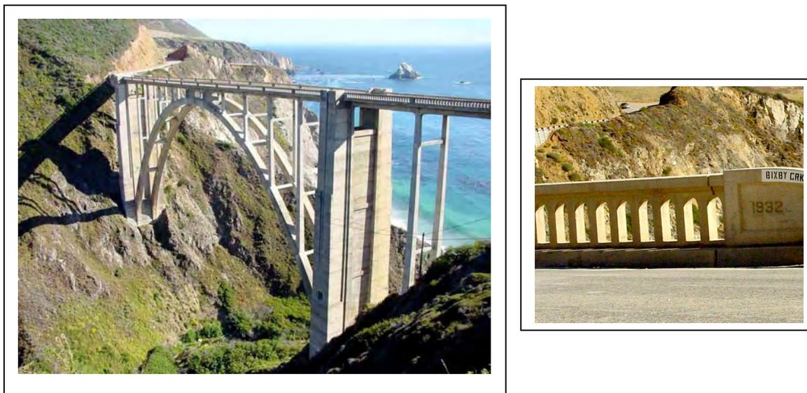
Figure 10: The internationally famous Bixby Creek Bridge in 2002. A close-up of the open balustrade bridge rail (right photo) is characteristic of the historic bridges along the Big Sur Coast.
