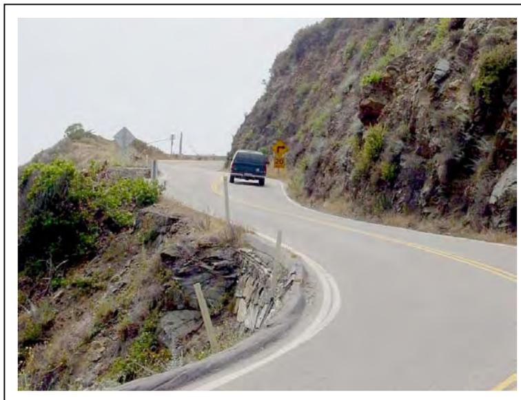
*Figure 4: Highway 1 on the southern section of the Big Sur Coast. In contrast to the Big Sur Valley area (see Figure 3), this section features a tighter plan and profile which requires slower travel speeds.*
