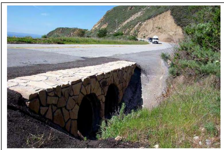
*Figure 14: The masonry on this newly constructed headwall is an example of design excellence that honors the overall aesthetic of the historic character and is distinguishable from the stone rubble masonry associated with the original highway construction. (Photo: Caltrans)*
