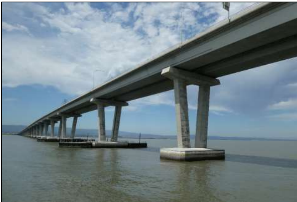
Photograph 4: Bents on Dumbarton Bridge, 8/17/2022, camera facing west.
