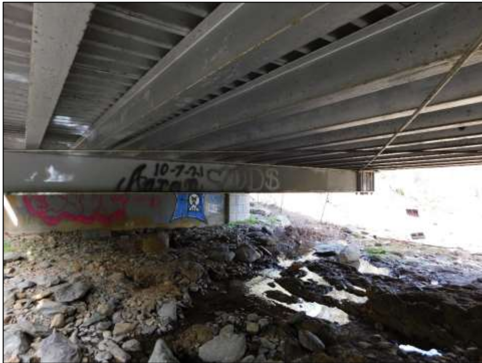
Photograph 6: Steel stringers, cross-beam, decking, and north abutment, camera facing northeast, March 2, 2022.
