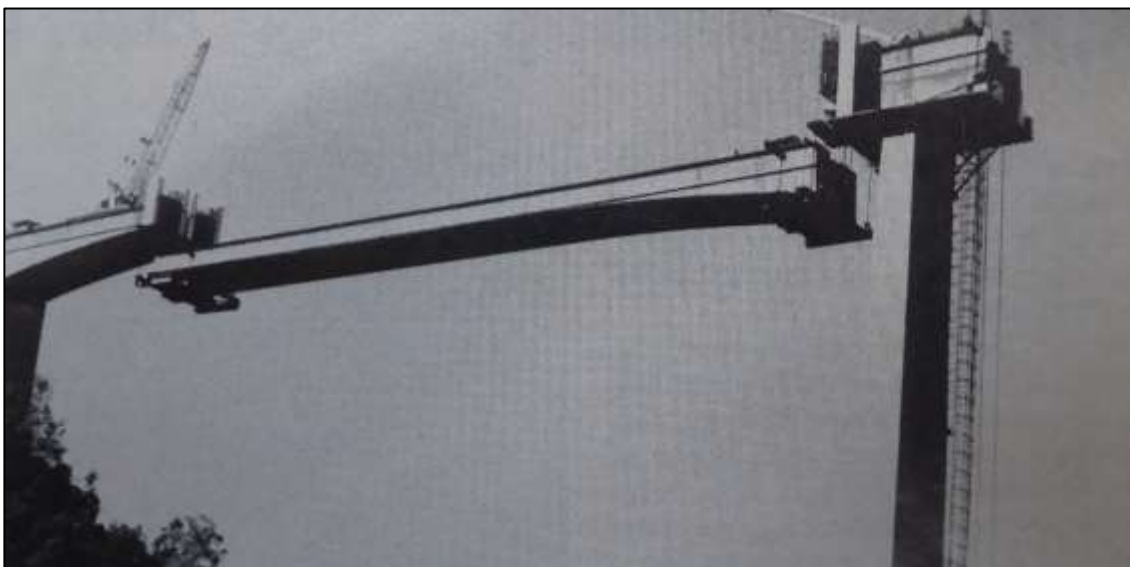
Plate 1. A 975-ton, 344-foot section between Piers 3 and 4 lifted into place in August 1975. 3
