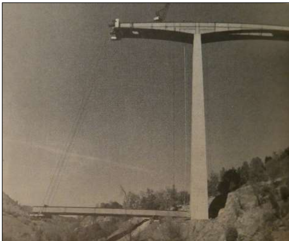
Plate 2. The center section of the main span being fabricated at the base of Pier 4. 4
