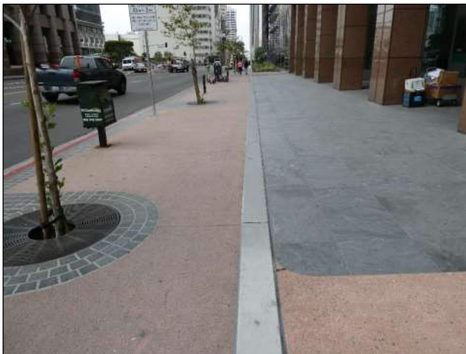
Photograph 9: Steel cover plate on sidewalk defines the edge of the viaduct, camera facing southwest, May 18, 2022.
