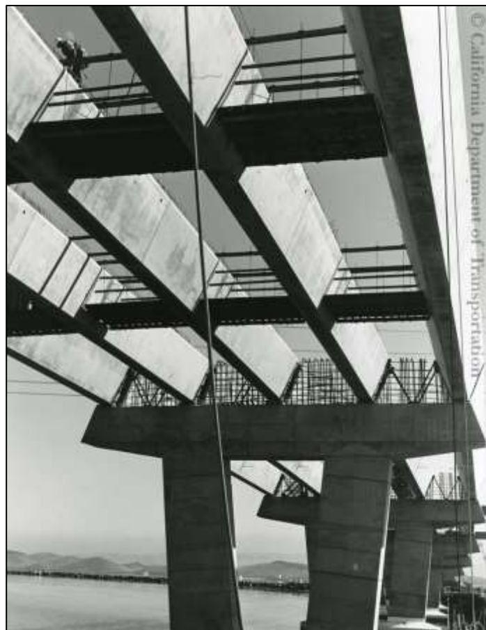
Plate 2. East concrete girder section under construction. 4
