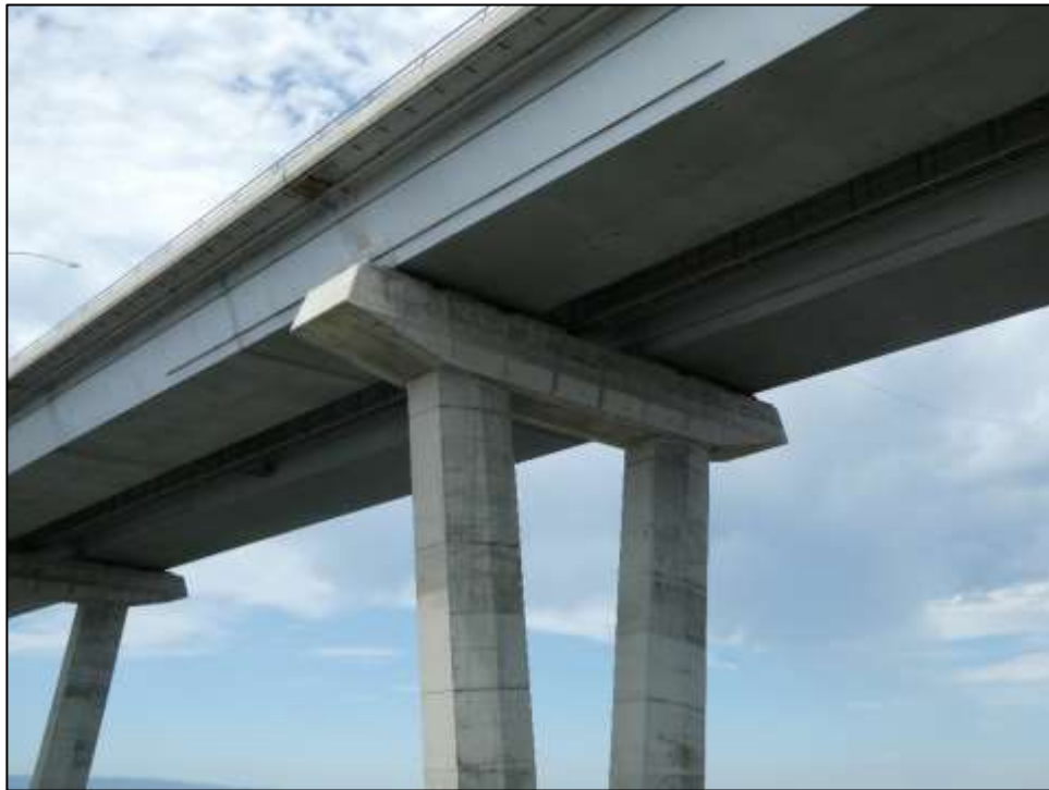
Photograph 6: Photo showing bent cap / steel box girder interface, camera facing west, August 17, 2022.
