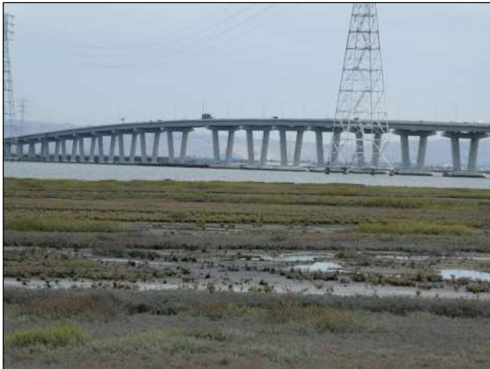
Photograph 2: North elevation showing steel box girder section, camera facing southeast, August 17, 2022.
