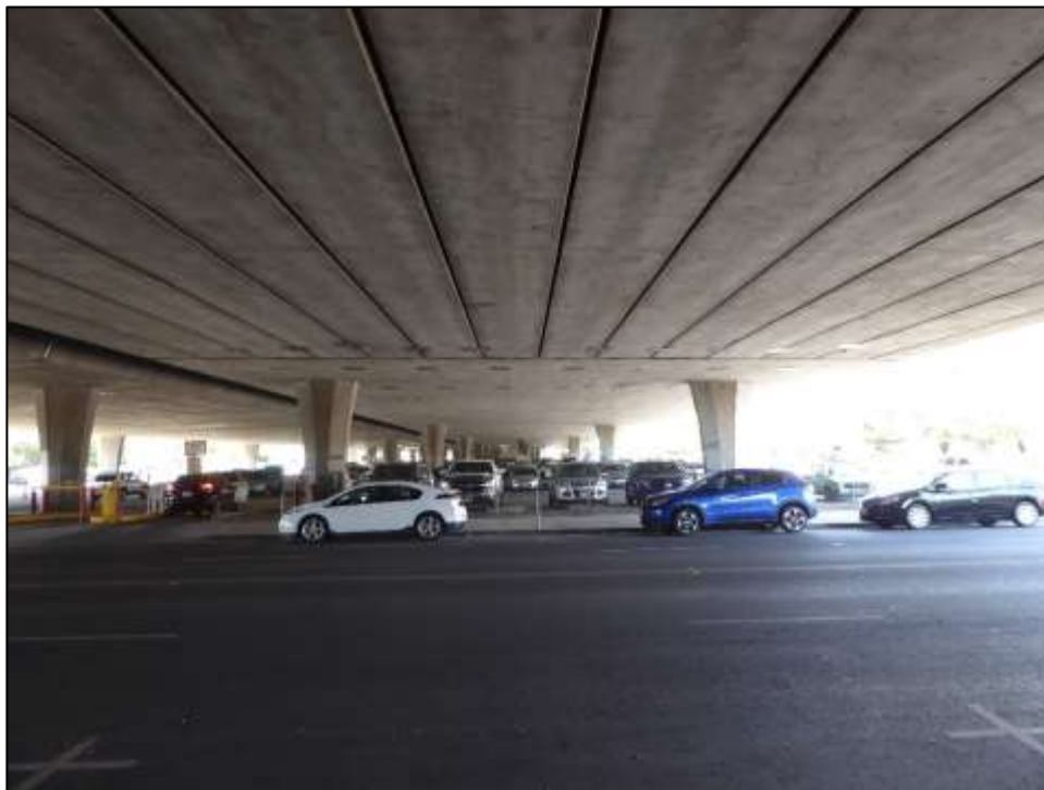
Photograph 4: Soffit of inverted T-girder span at South Sutter Street, camera facing west, April 28, 2022.
