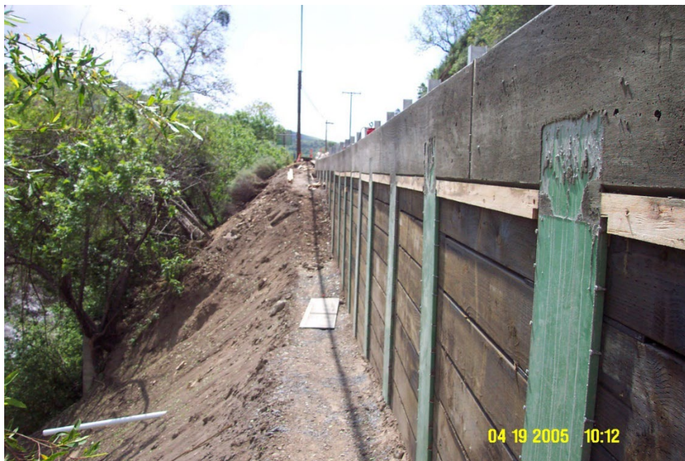
Figure 7-2. Soldier Pile Wall with Cap Beam
