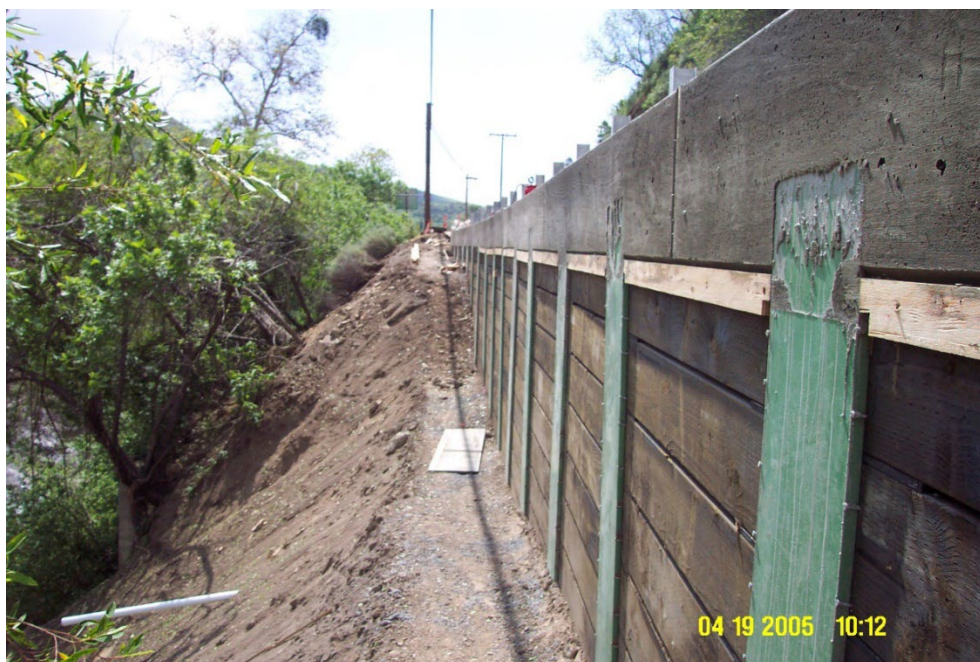
Figure 7-2. Soldier Pile Wall with Cap Beam
