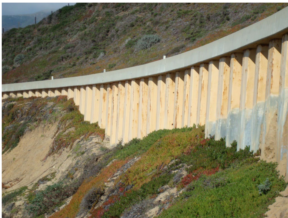
Figure 7-1. Sheet Pile Wall with Cap Beam
