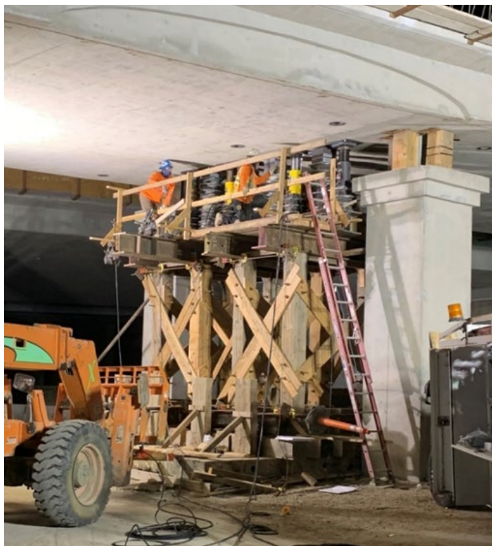
Figure 9-2. Temporary Support for Bridge Lowering
