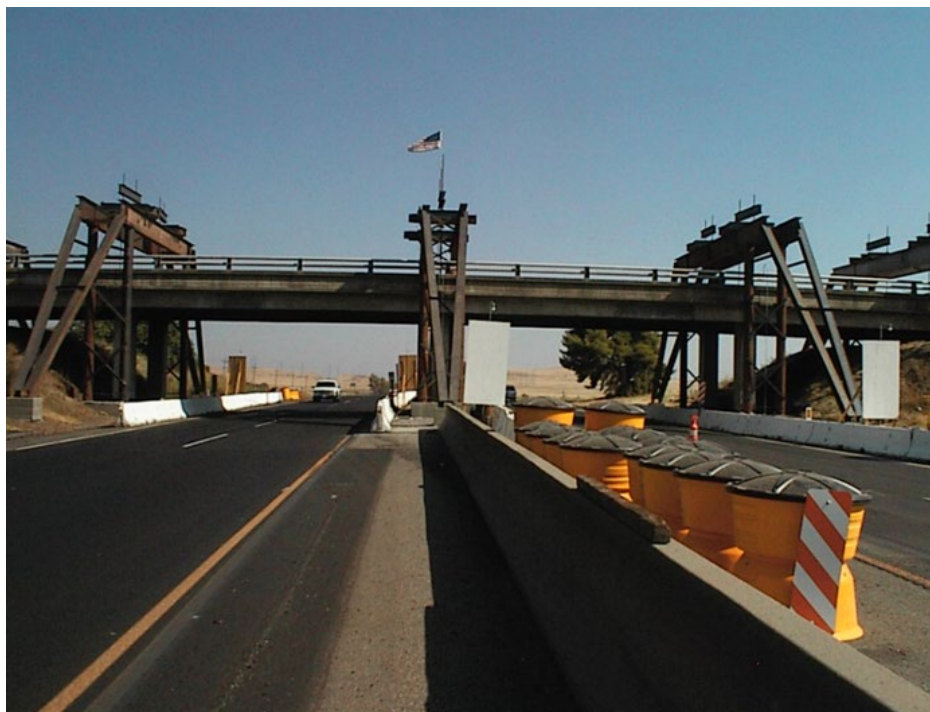
Figure 9-3. Temporary Support Highway 70 Bridge Raising
