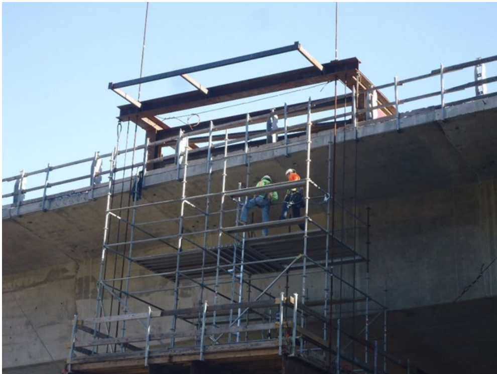
Figure 7-1. Conventional Scaffold System Supported by Structure
