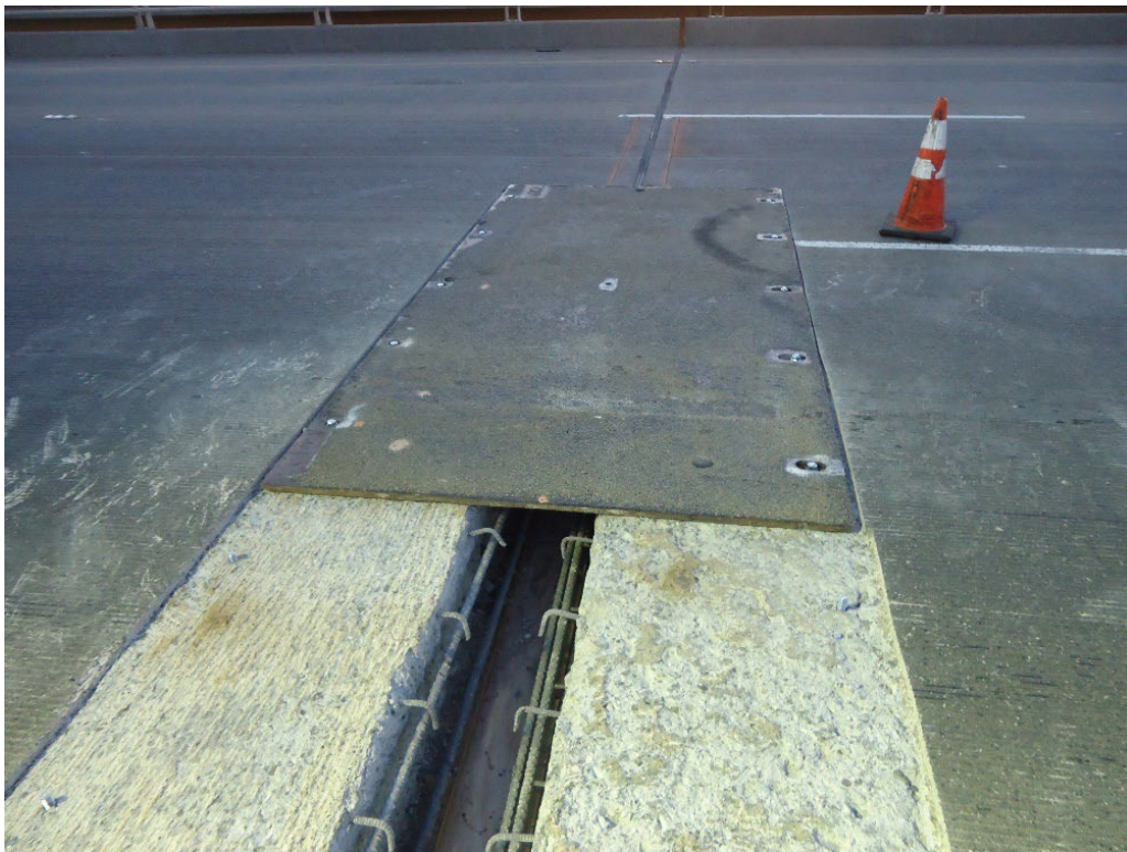
Figure 6-1. Recessed Deck Plates Installed for Deck Joint Replacement Sacramento River BOH, Bryte Bend (Br. NO. 22-0026). Route: 80
