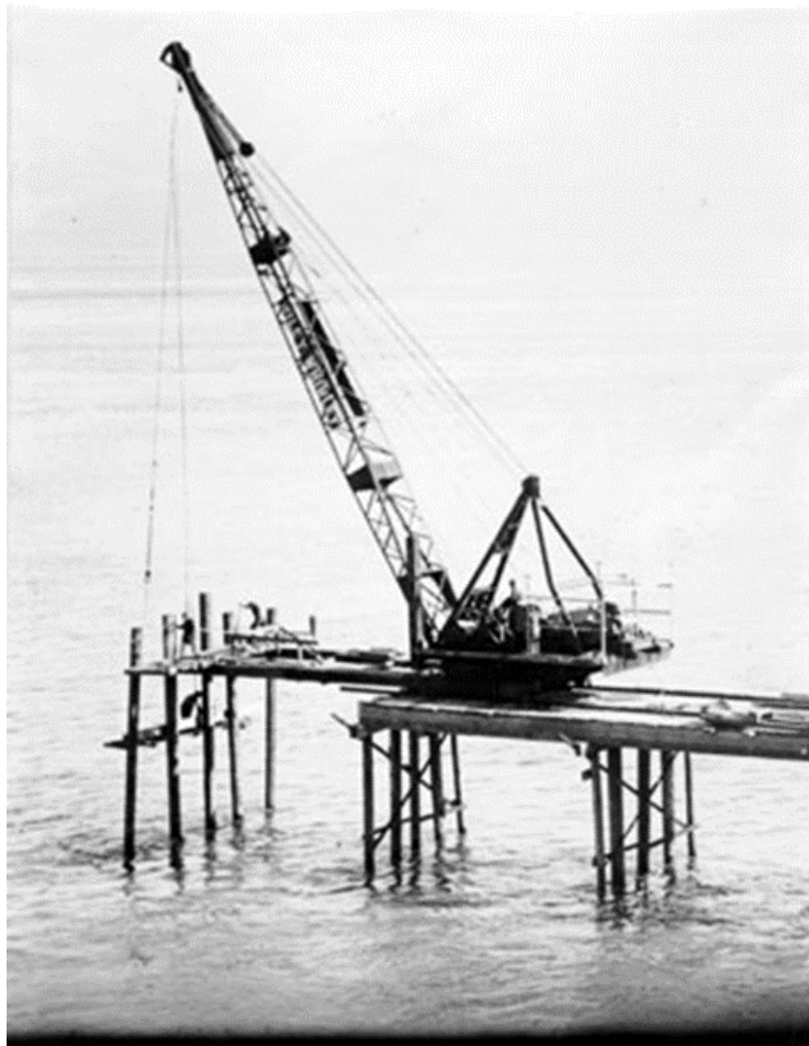
Figure 4-12. Trestle Used at Golden Gate Bridge, c.1934
