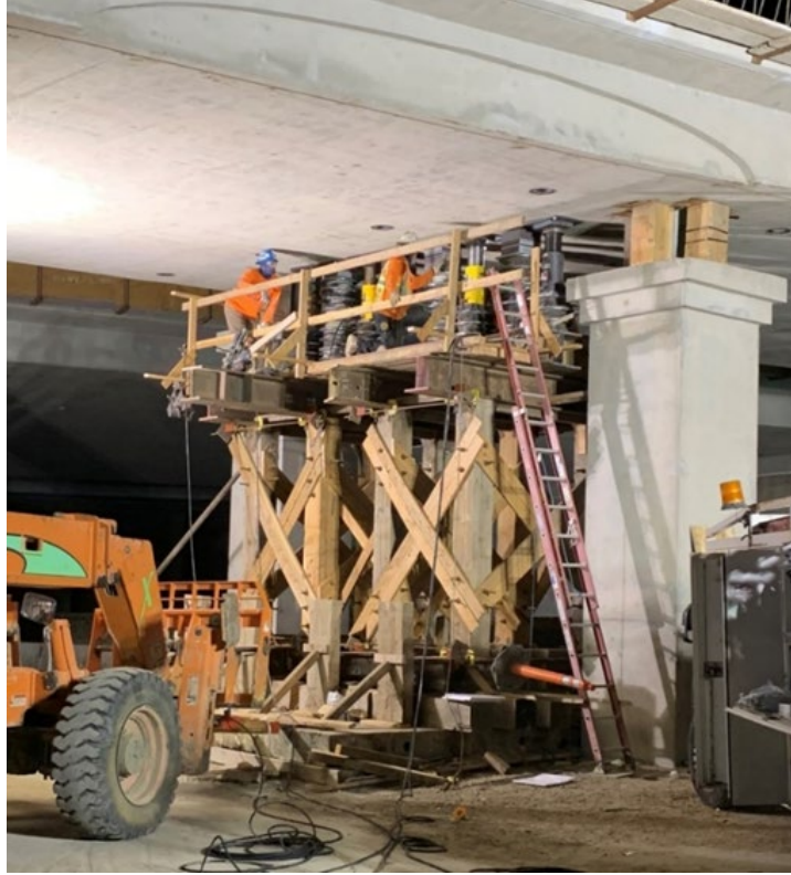
Figure 9-2. Temporary Support for Bridge Lowering
