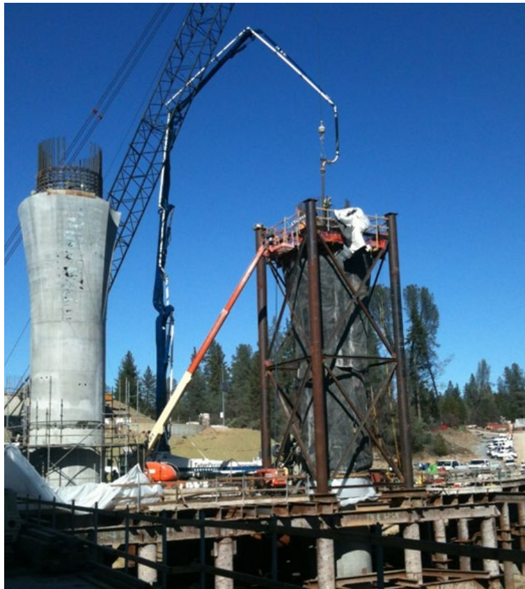
Figure 5-2. Support Frame System, Antlers Bridge
