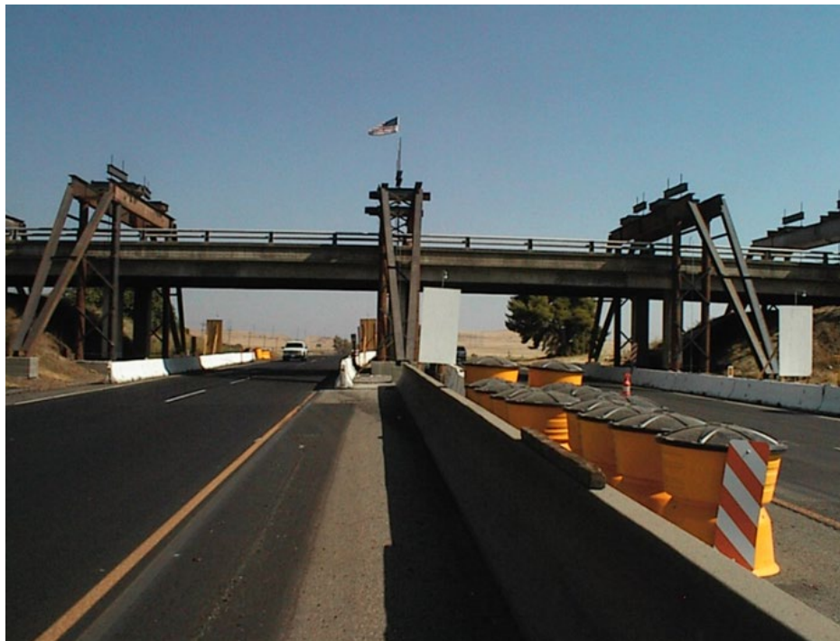
Figure 9-3. Temporary Support Highway 70 Bridge Raising
