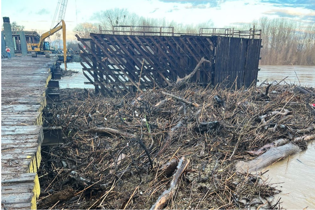
Figure 4-10. Debris Buildup Against Trestle
