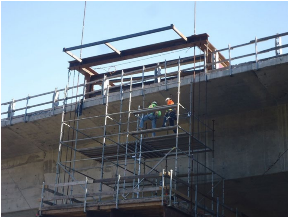
Figure 7-1. Conventional Scaffold System Supported by Structure
