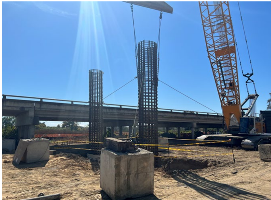
Figure 5-1. Guy Wire System, Butte City Bridge
