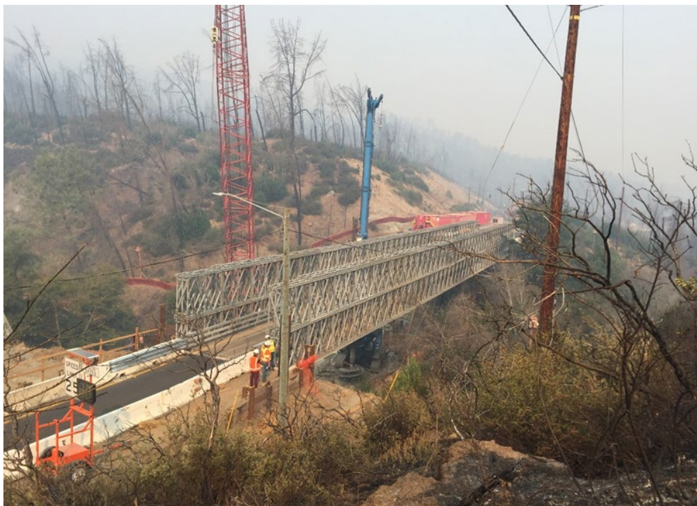
Figure 8-2. Temporary Modular Steel Truss Bridge – Capell Creek
