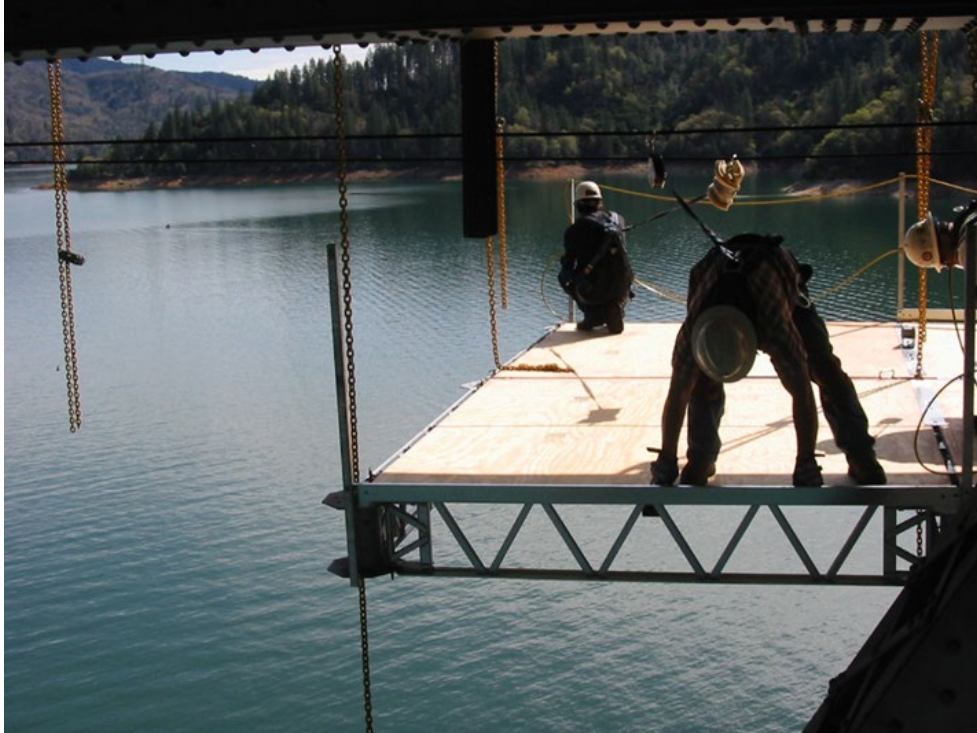
Figure 7-2. Suspended Scaffold System - Quikdeck
