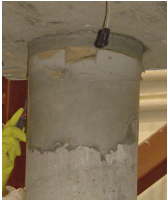
Figure 7-19. Prepared Concrete Column Surface
