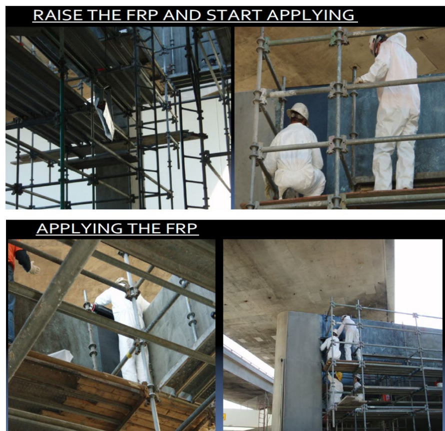
Figure 7-25. Repair of Fire Damage Using FRP
