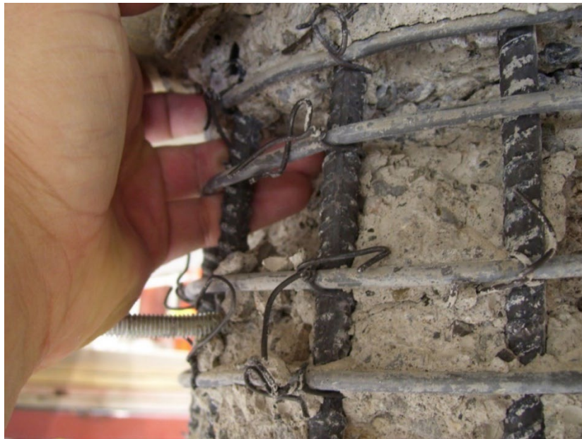
Figure 7-17. Removal of Unsound Concrete (Column Crack Visible)
