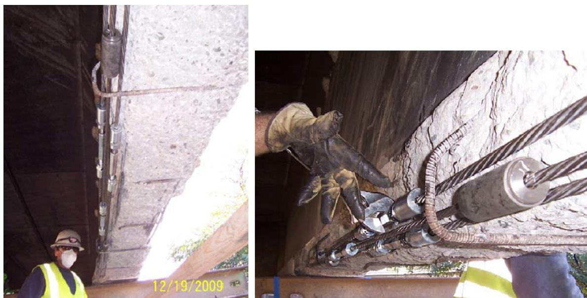
Figure 7-12. Strand Splices Are Staggered
