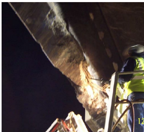
Figure 7-1. Removal of Unsound Concrete
