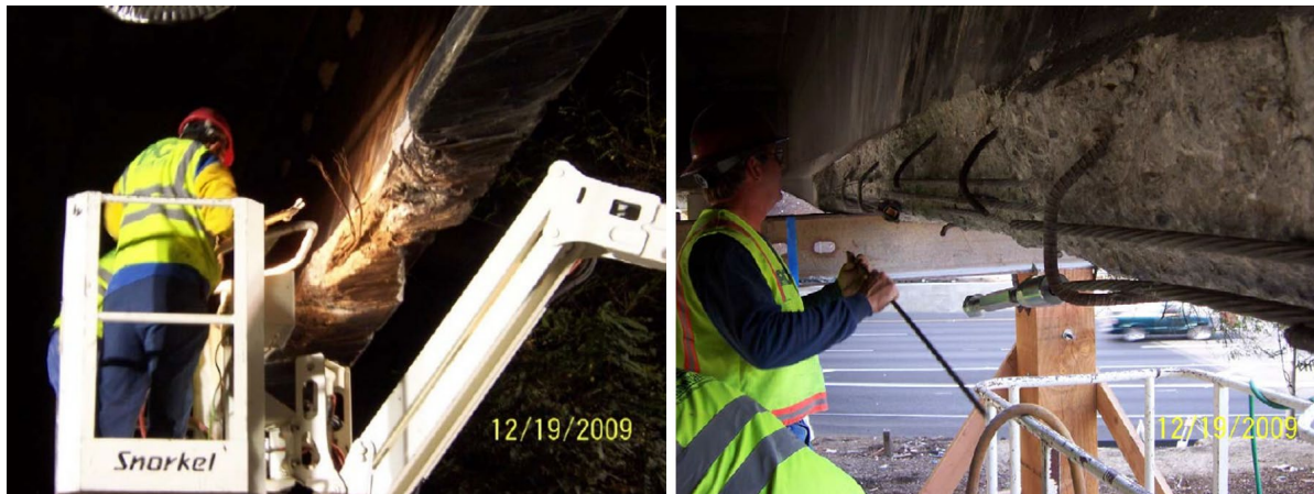
Figure 7-2. Exposing, Cleaning, and Repairing Prestressing Steel
