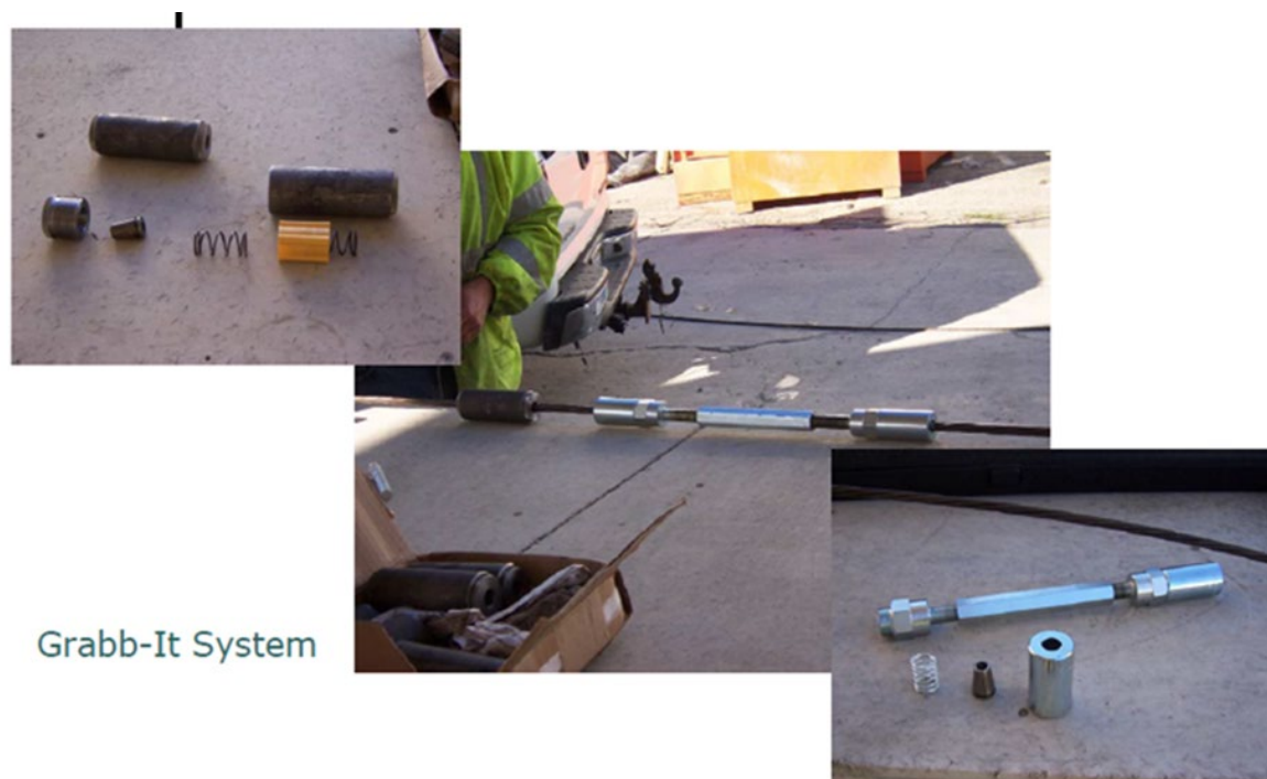
Figure 7-8. Single Strand Splice
