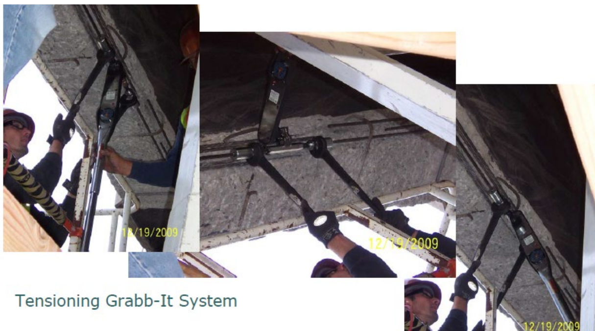
Figure 7-11. Installation of Splicing System
