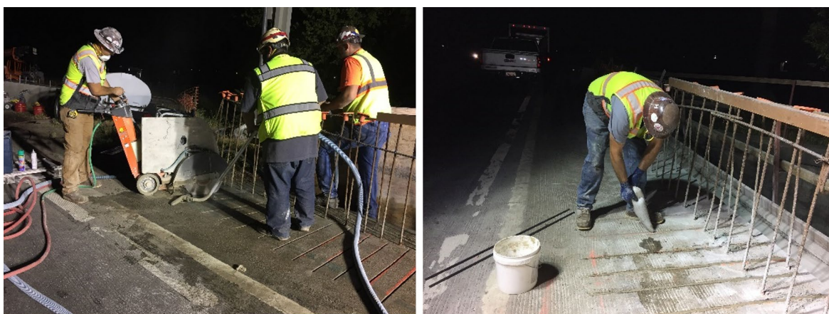
Figure 7-27. Construction of Overhang Retrofit Using FRP
