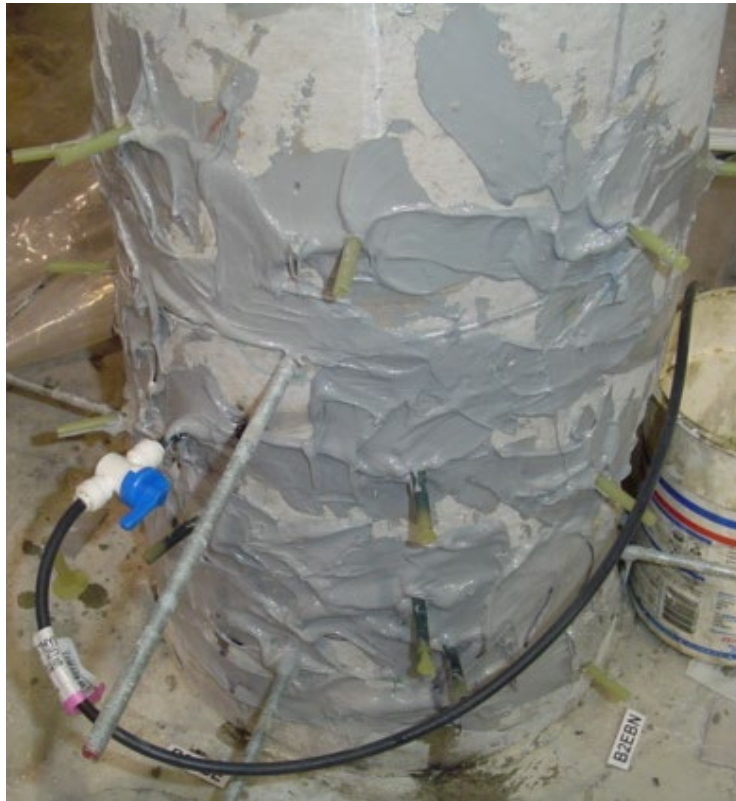
Figure 7-18. Epoxy Injection to Fill Cracks
