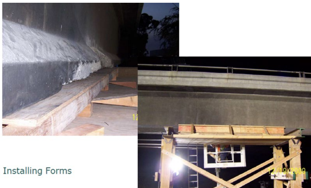
Figure 7-4. Forming for Recasting of Concrete
