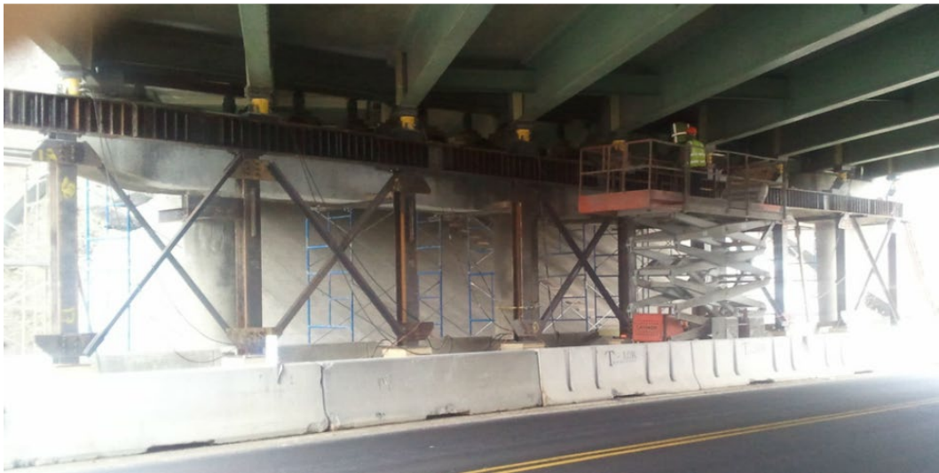
Figure 6-6. Temporary Support Example
