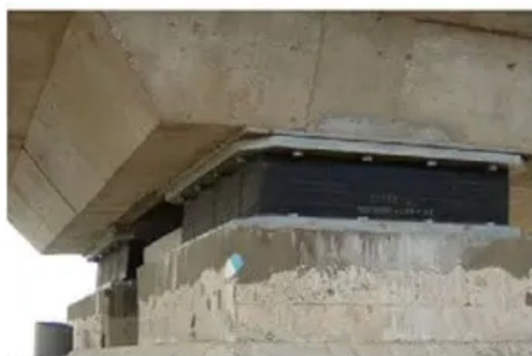
Figure 6-4. PTFE/Elastomeric Bearing
