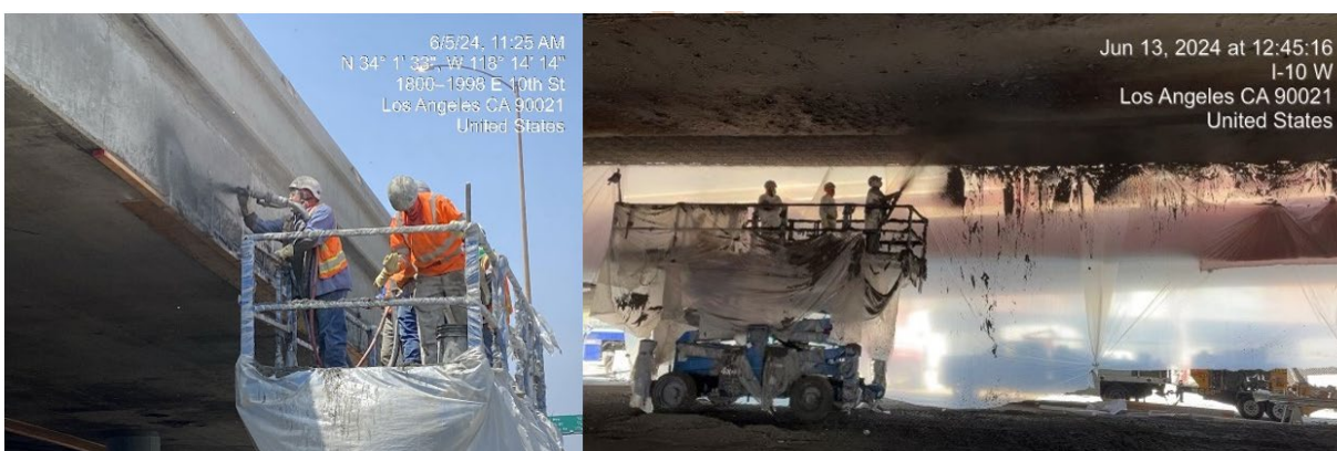
Figure 5-25. Shotcrete Used to Repair Exterior Girder and Soffit
