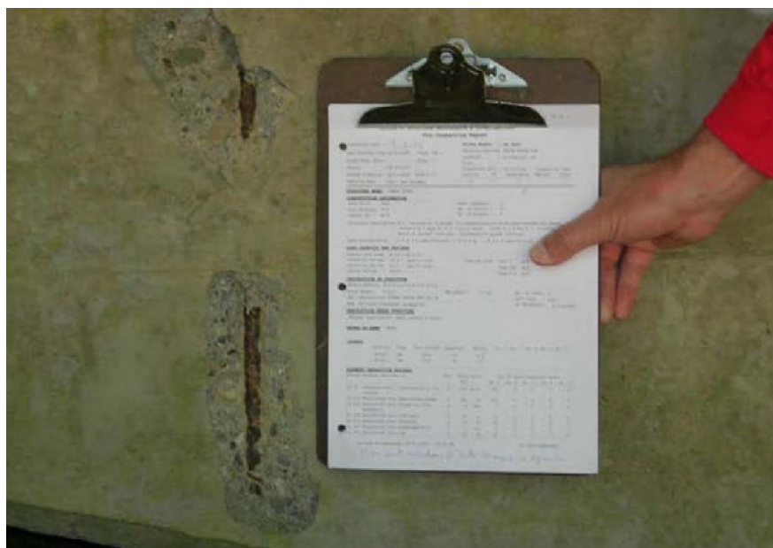
Figure 5-5. Spalling
