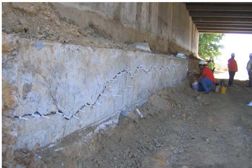
Figure 5-26. Installing Injection Ports
