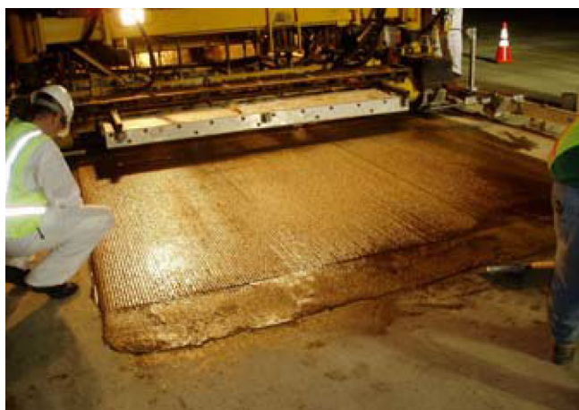
Figure 5-53. Trial Polyester Concrete Overlay of a Slab
