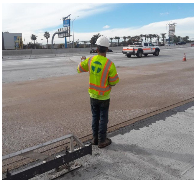
Figure 5-64. Completed Paving Surface using Appropriate Paving Machine
