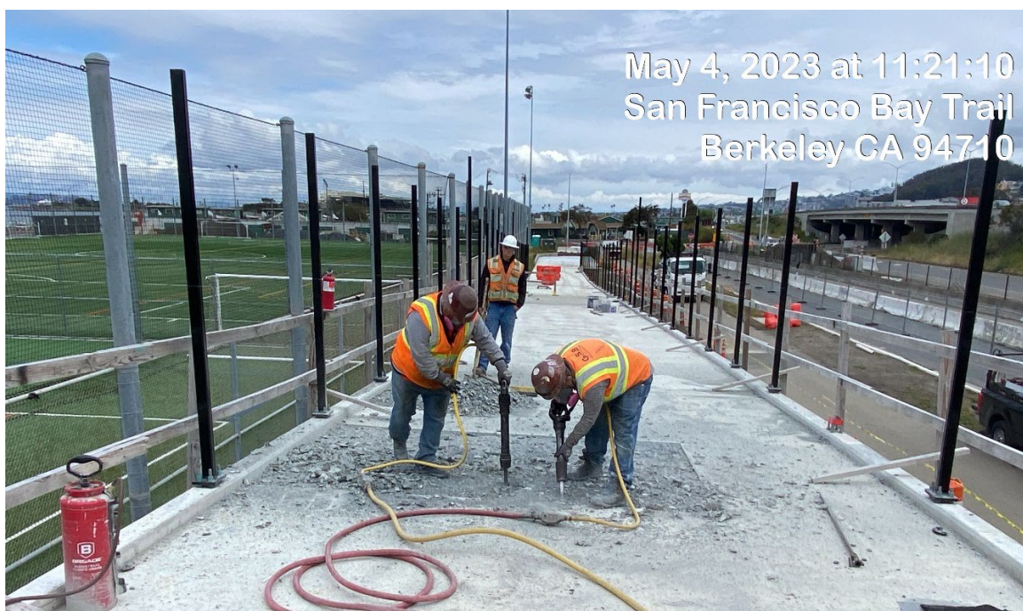
Figure 5-38. Concrete Removal During Bridge Deck Refinishing
