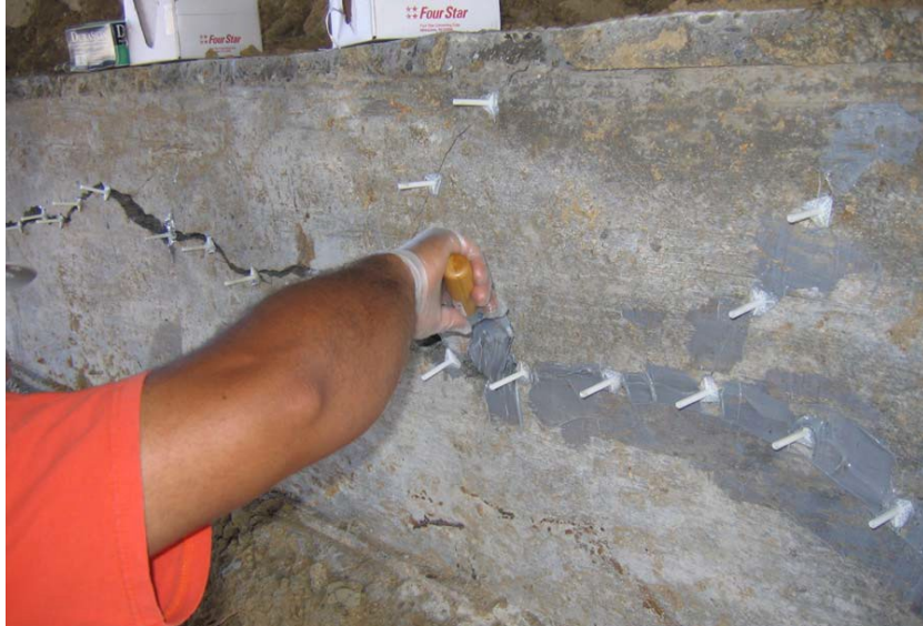
Figure 5-27. Sealing a Crack Between Injection Ports
