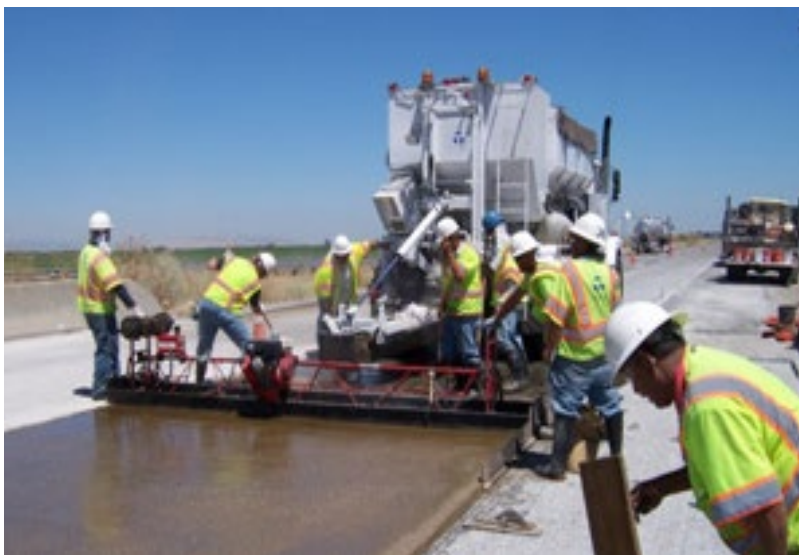
Figure 5-61. “Texas” Screed with Fixed Ski Controlled Grading
