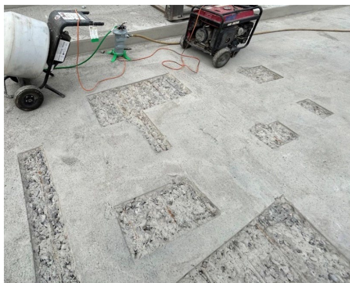
Figure 5-19. Unsound Concrete Removed and Areas Prepared
