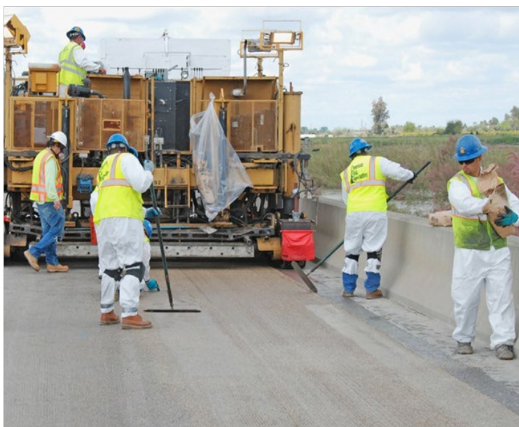
Figure 5-62. Paving Machine with Laser Guided Screed
