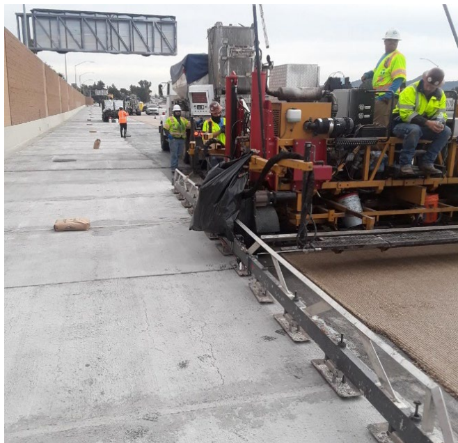
Figure 5-63. Sample Paving Machine with Automatic Screed Control
