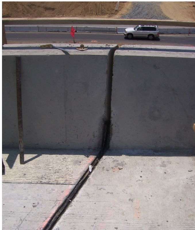
Figure 4-14. Deck Joint Extending through the Barrier
