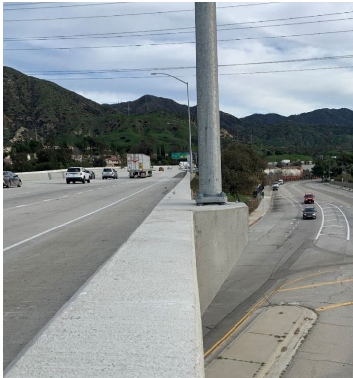
Figure 4-7. Bridge Barrier with Electrolier Pedestal
