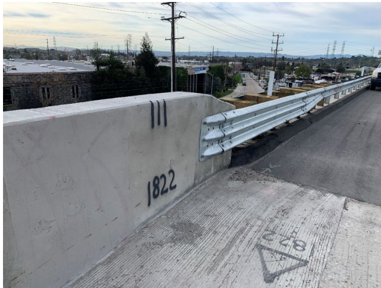
Figure 4-6. Bridge Barrier with Transition to Metal Beam Guard Rail
