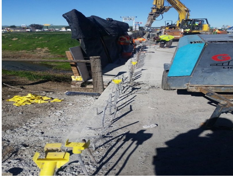
Figure 4-25. Temporary Protective Structure Used for Forming Support and Walkway
