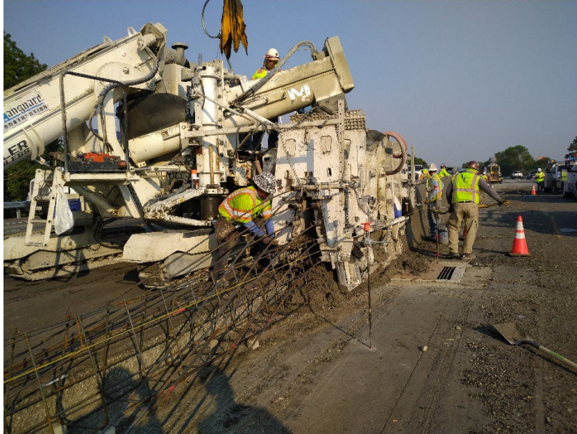
Figure 4-33. Example of Slip-forming
