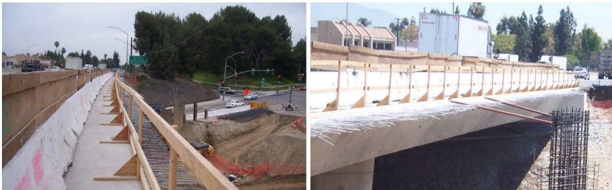
Figure 4-24. Temporary Fall Protection
