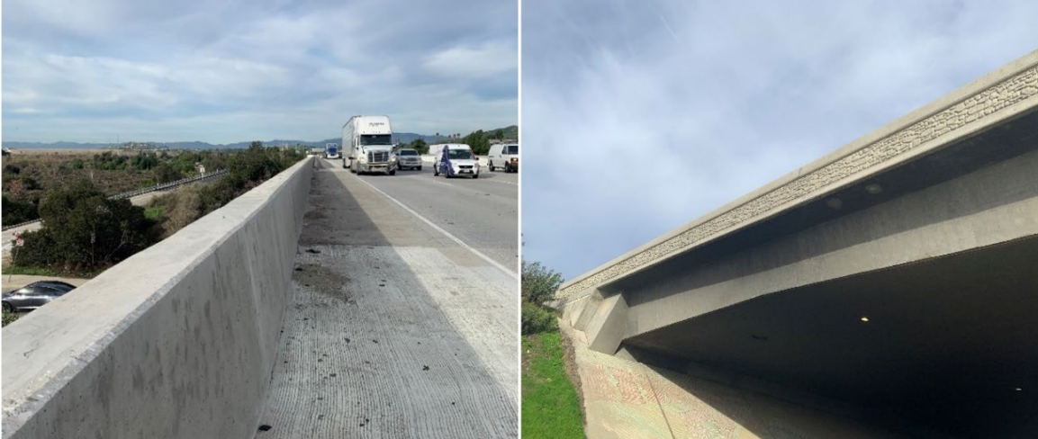
Figure 4-4. Bridge Concrete Barrier at the Edge of Deck
