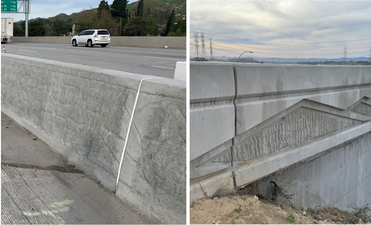
Figure 4-8. Bridge Barrier Expansion Joints
