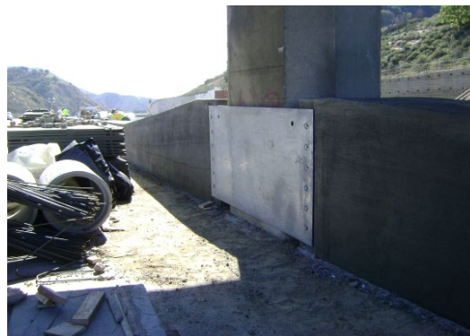
Figure 4-26. Column Protection Steel Cover Plate Installed with Drill and Bond
