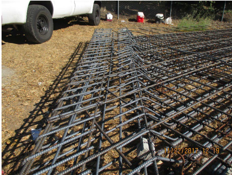
Figure 3-3. Reinforcement to Account for Prestressing Blocks
