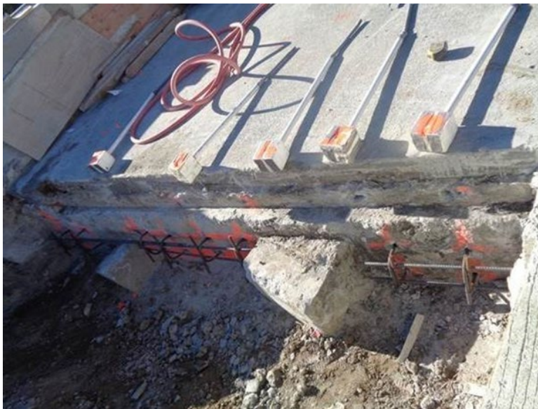
Figure 3-2. Prestressing Blocks
