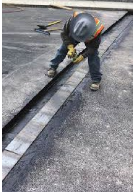
Figure 2-25. Plate over Joint Installed
