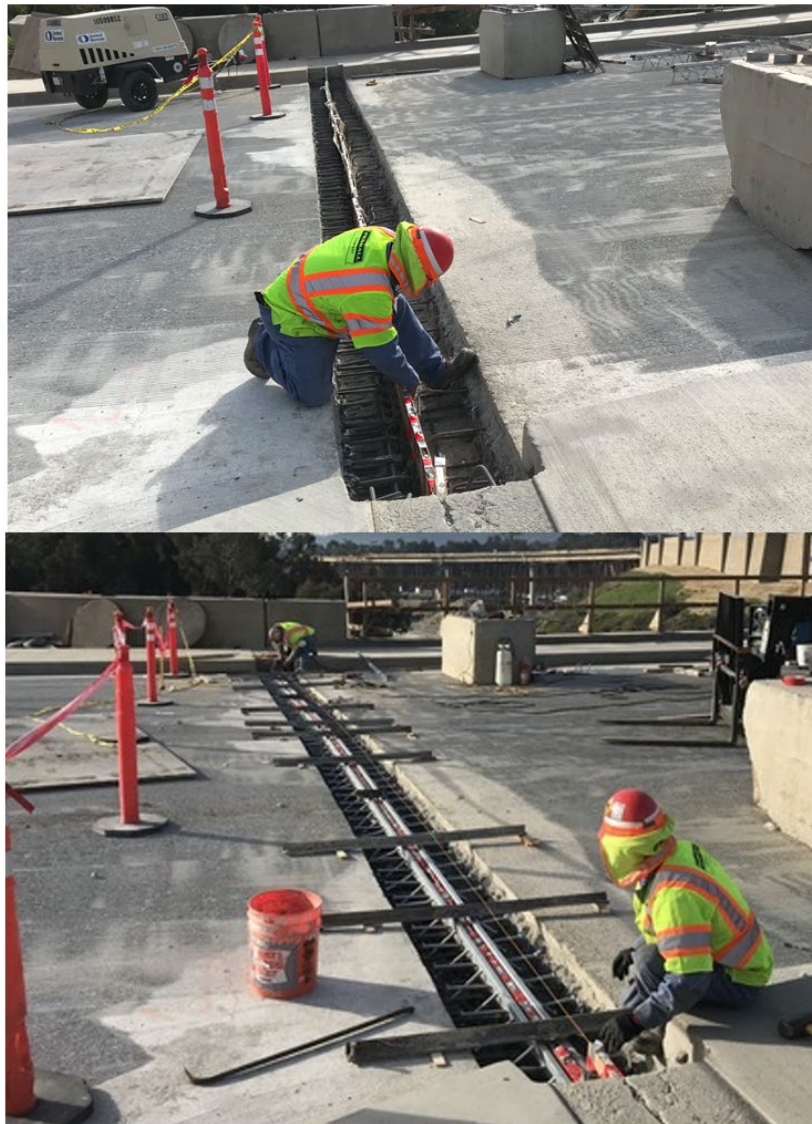
Figure 2-21. Joint Seal Assembly Blockout and Installation
