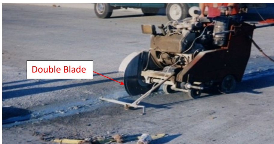
Figure 2-13. Double Blade Saw Cutting to Create Joint Groove
