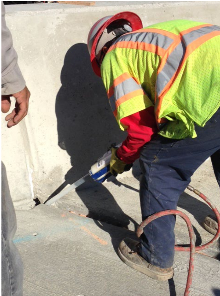
Figure 2-11. Type A Seal Being Poured into the Joint
