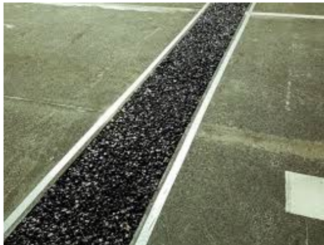
Figure 2-26. Asphalt Binder Mix Is Placed
