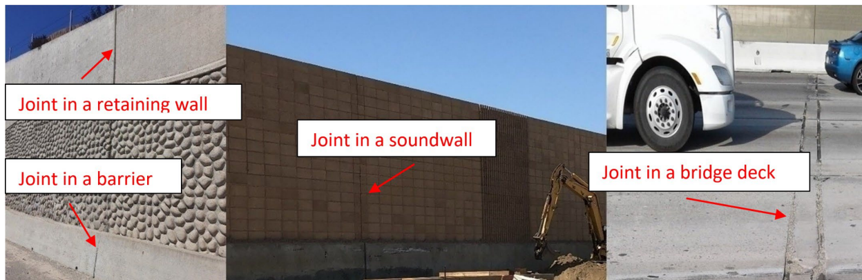
Figure 2-1. Joints in Various Types of Structures
