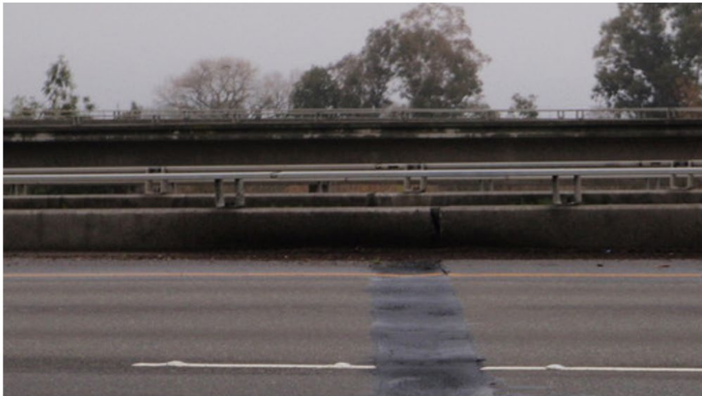
Figure 2-5. Asphaltic Plug Joint Seal
