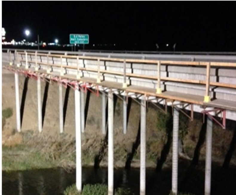
Figure 1-3. Temporary Walkway and Debris Containment
