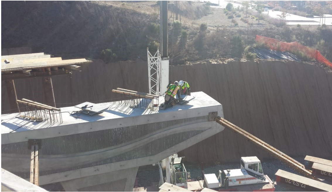
Figure C-3. Installation of PTFE Spherical Bearings (Petaluma River Bridge Project)
