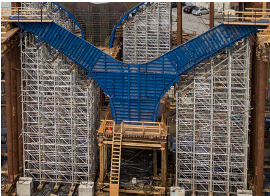
Figure 1-3. Proprietary Shoring System
