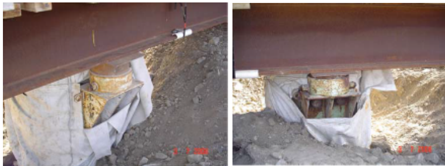
Figure 9-2. Steel Sand Jacks.
