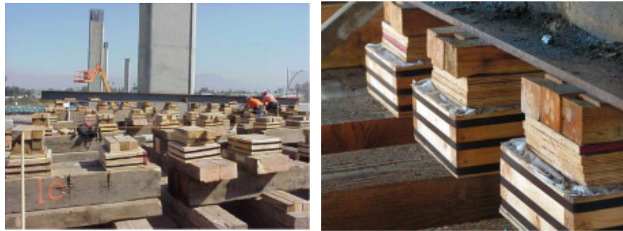
Figure 9-1. Wood Sand Jacks.
