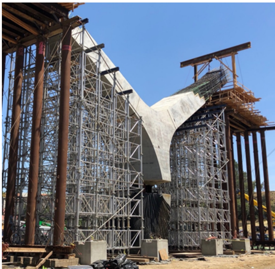
Figure 7-13. Heavy Duty Shoring System.
