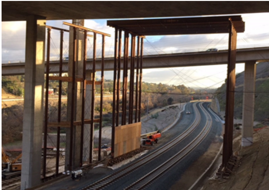
Figure 1-2. Pipe Post Falsework System
