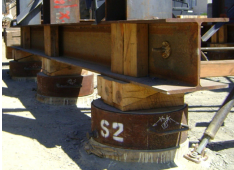
Figure 7-3. Steel Sand Jack.
