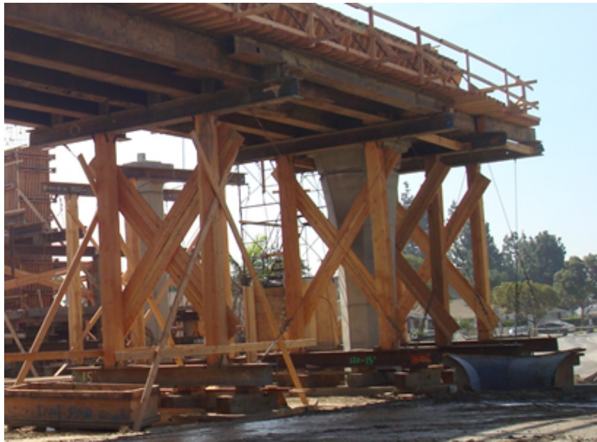
Figure 1-1. Common Falsework System
