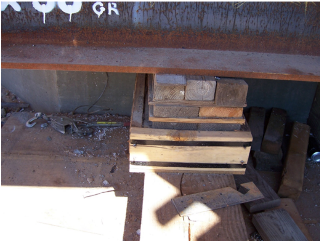
Figure 7-1. Wood Sand Jacks.
